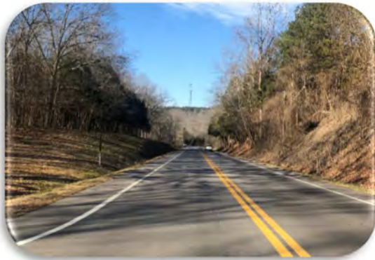
Highway 70 looking Eastbound
