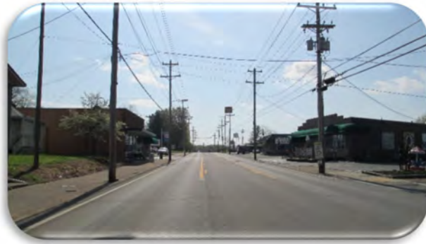
Highway 70 looking Eastbound Sidewalk on Both Sides
