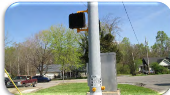
Dark Pedestrian Signal on Northwest corner
