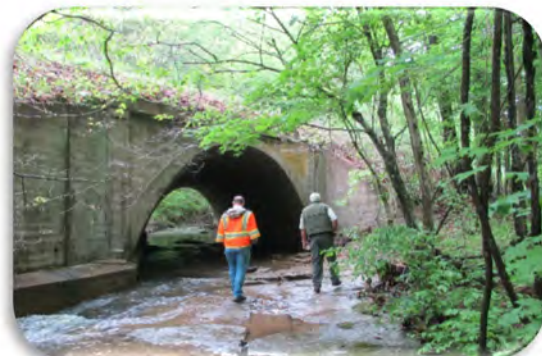
Existing Tunnel under Highway 70
