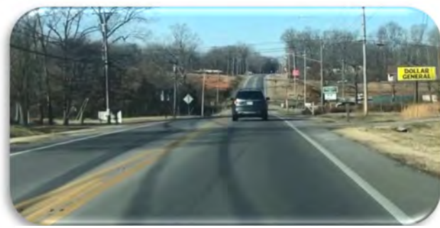
Highway 70 looking Westbound West of SR 47N
