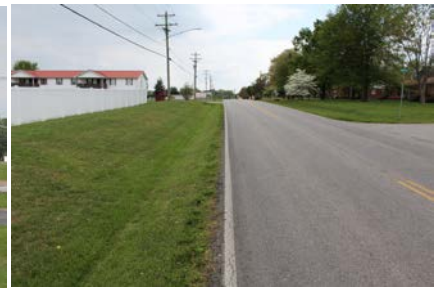
Figure 5: Drainage Ditch Along Roadway
