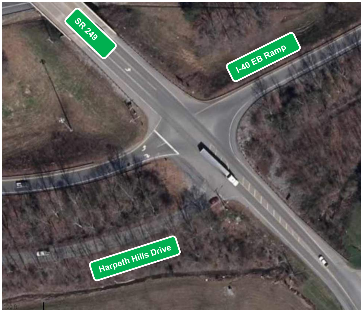
FIGURE 14: HARPETH HILLS DRIVE INTERSECTION
