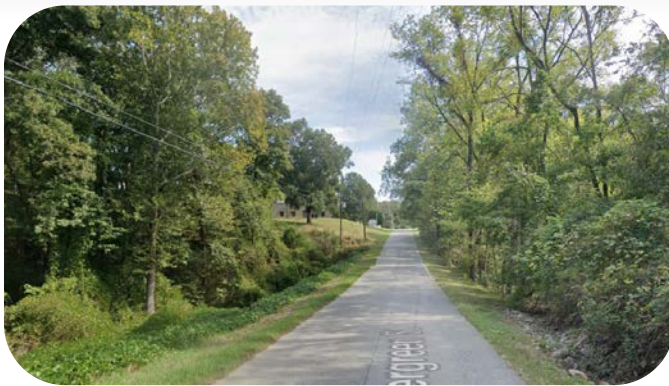
IN NEED OF PEDESTRIAN INFRASTRUCTURE
