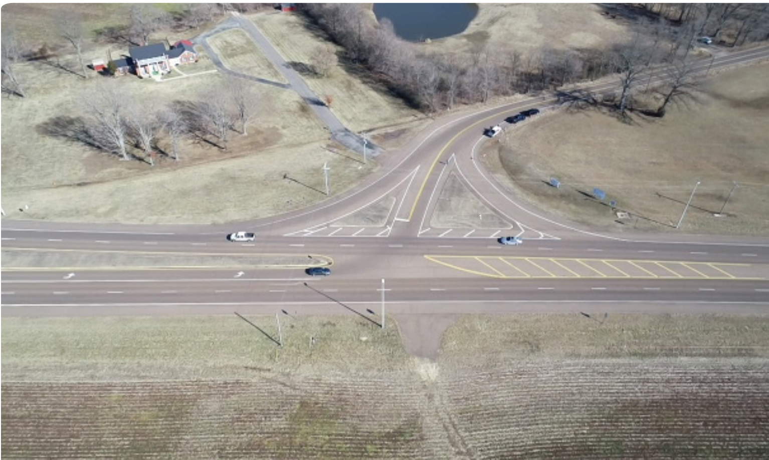
LOOKING EAST AT THE INTERSECTION OF HIGHWAY 22 AND PIKEVIEW STREET.
