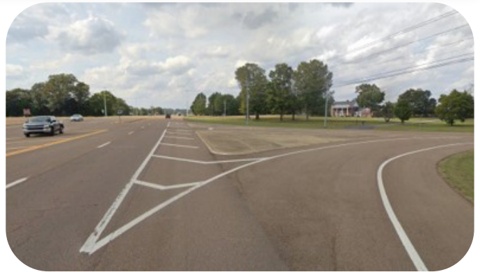
RAMP ONTO HWY-22 NEEDS SAFETY IMPROVEMENTS
