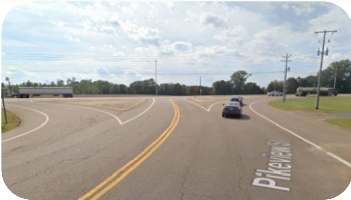
CONCERN ABOUT VEHICULAR SAFETY AT EXIT
