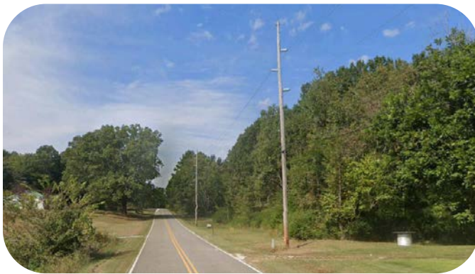
POWERLINES NORTH OF EVERGREEN ST
