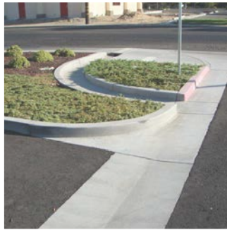
Streets are re-aligned for safety
