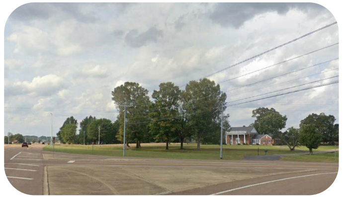
POWERLINES ALONG PIKEVIEW STREET
