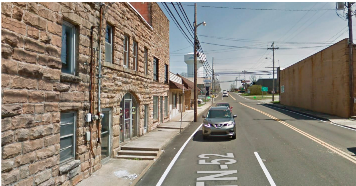
FIGURE 5: CENTRAL AVENUE (SR 52) BETWEEN MAIN STREET AND NORRIS STREET Demonstrates stairs in the sidewalk
