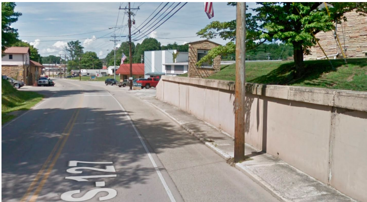
FIGURE 7: MAIN STREET AT MCGHEE STREET Demonstrates sidewalk less than five (5) feet wide and utility pole obstruction
