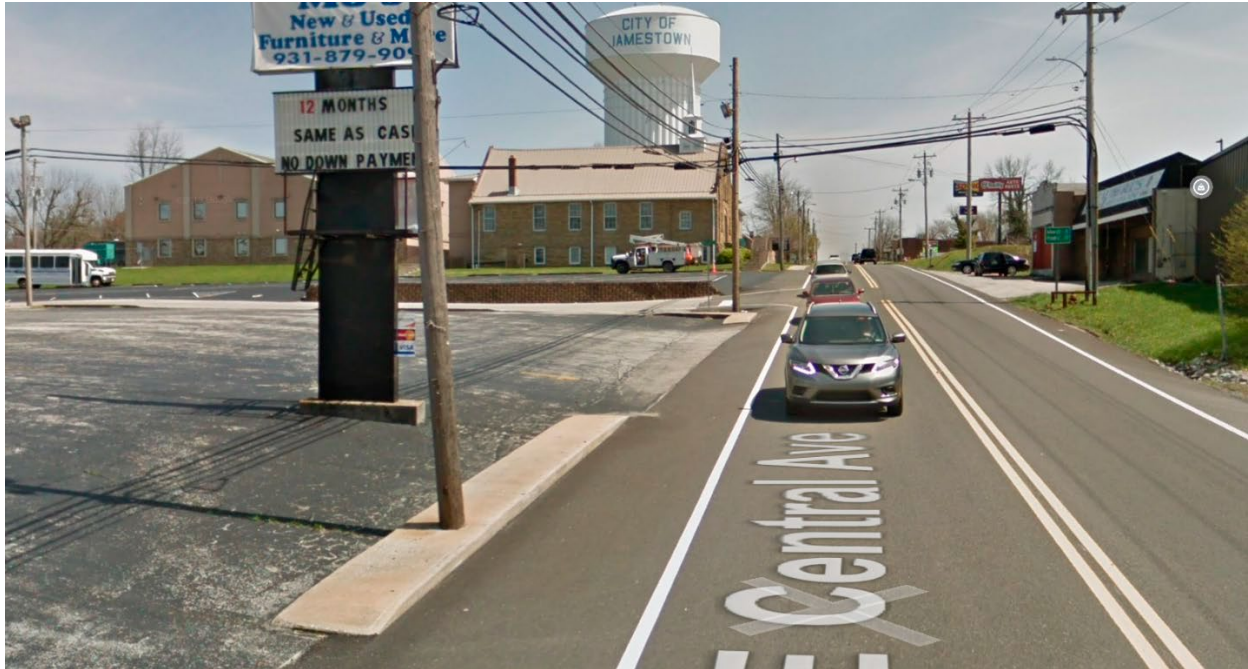
FIGURE 6: CENTRAL AVENUE (SR 52) BETWEEN NORRIS STREET AND WHITE OAK STREET Demonstrates utility pole in the center of the sidewalk, sidewalk less than five (5) feet wide, and open frontage creating gaps in the sidewalk
