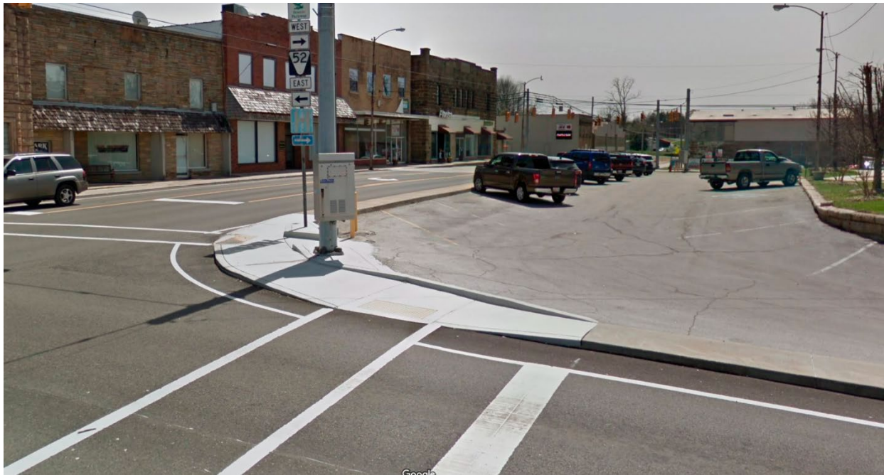
FIGURE 4: CENTRAL AVENUE (SR 52) AT MAIN STREET Demonstrates no pedestrian heads at signalized intersection
