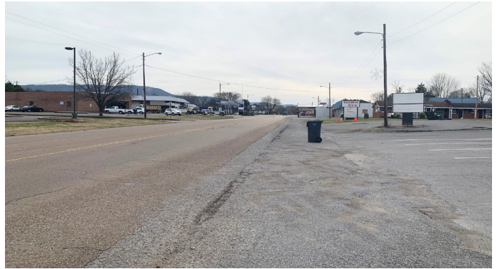
Uncontrolled access to North Main Street from adjoining parking areas.
