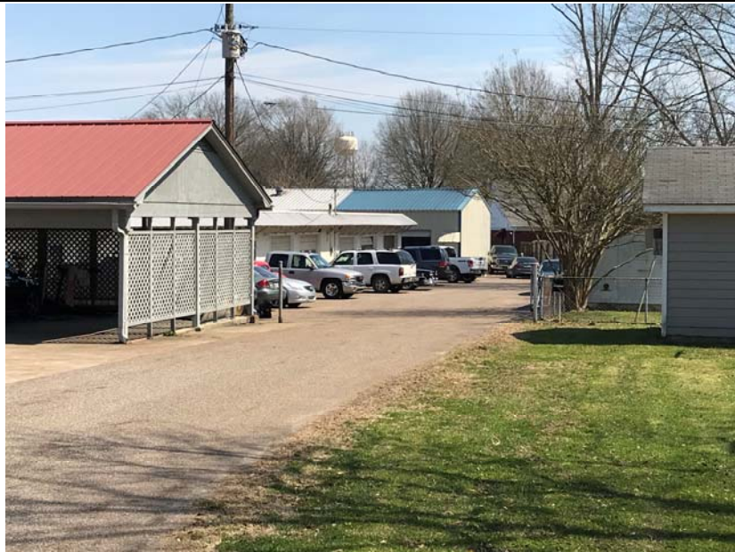
Photo 5. EPA "air pollution" site located at 226 Arendall Street.
