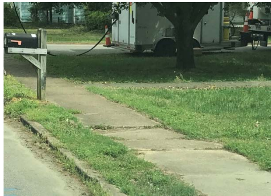
VERTICAL FAULTING
