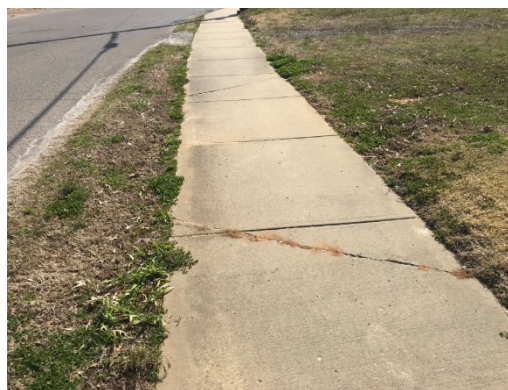
CRACKED PANELS
