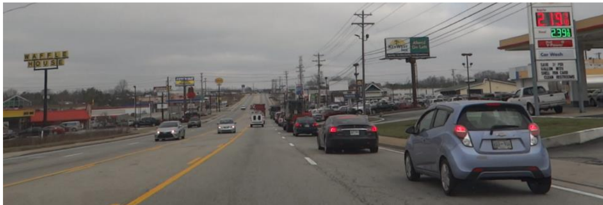
Figure 3: Northbound S. Willow Avenue (SR 135) north of I-40
