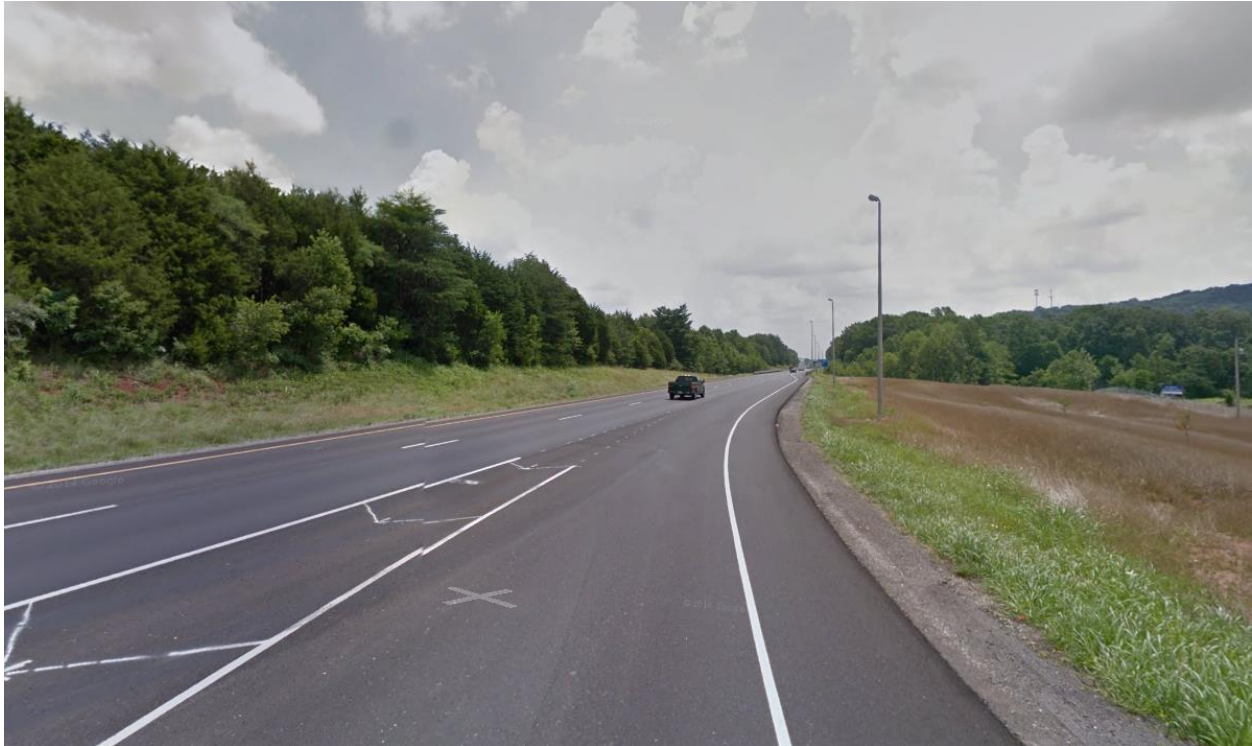
Figure 2: I-40 Eastbound On-Ramp from S. Willow Avenue (SR 135)
