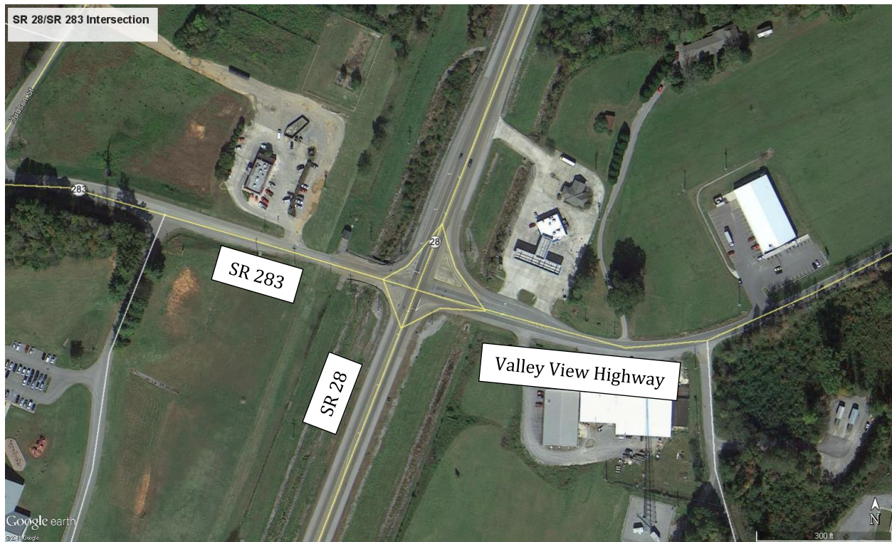
Figure 3-24 Aerial of SR 28/SR 283 Intersection
