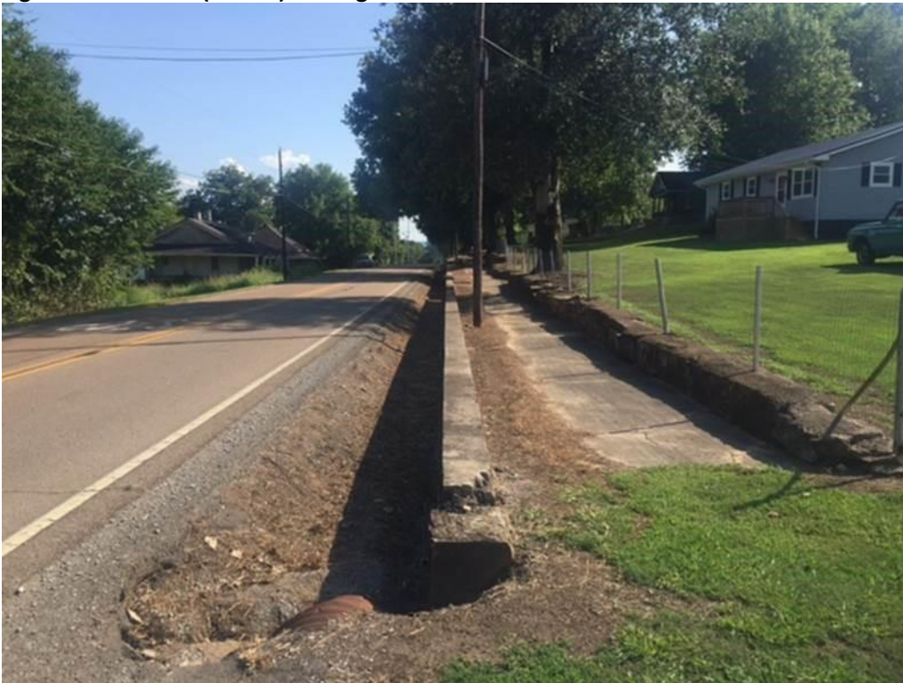
Figure 5-5 Main St. (SR 108) looking North
