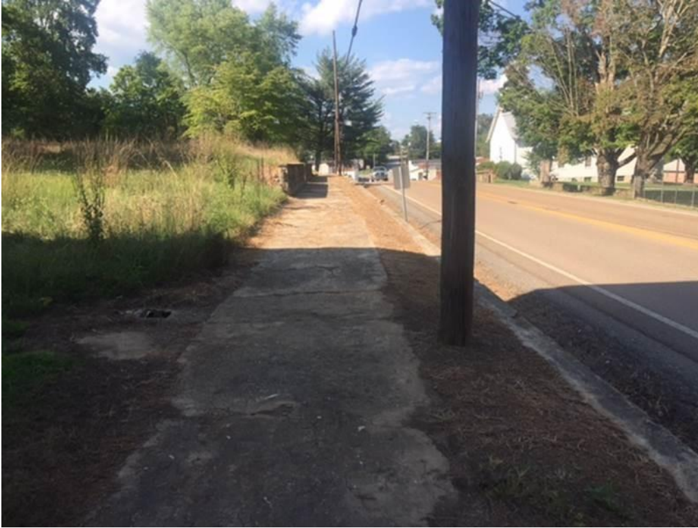
Figure 5-4 Main St. (SR 108) looking South
