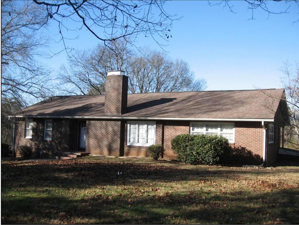
Figure 35: View northwest of a 1960 brick Ranch dwelling at 3405 E. Lamar Alexander Parkway.
