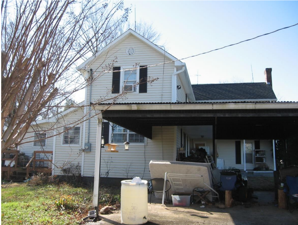
Figure 111: BT-2240 in 2022, view to the west.
