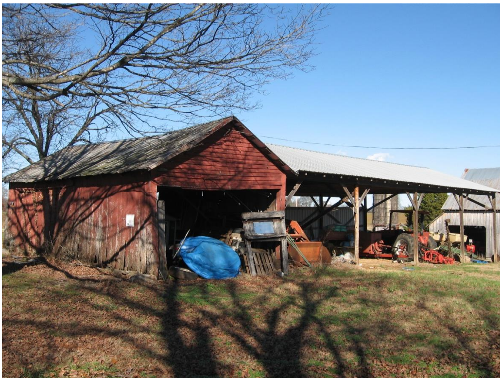
Figure 112: BT-2240, garage and attached equipment shed, view to the northeast.
