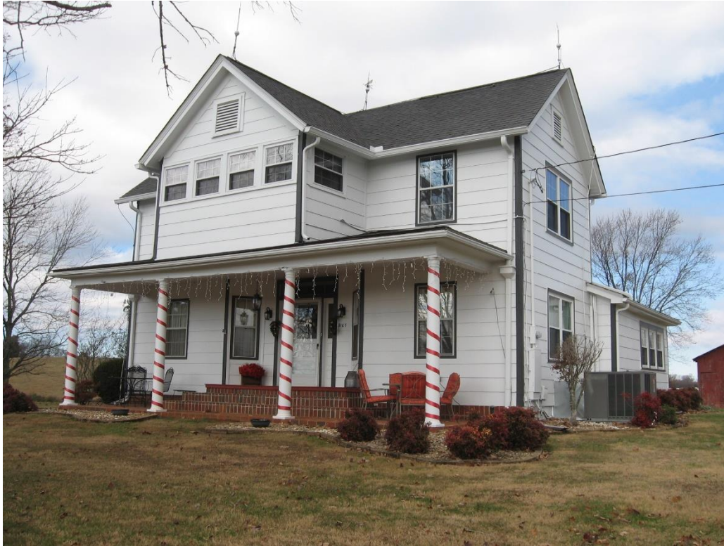
Figure 79: BT-2266 in 2022, view to the northwest.
