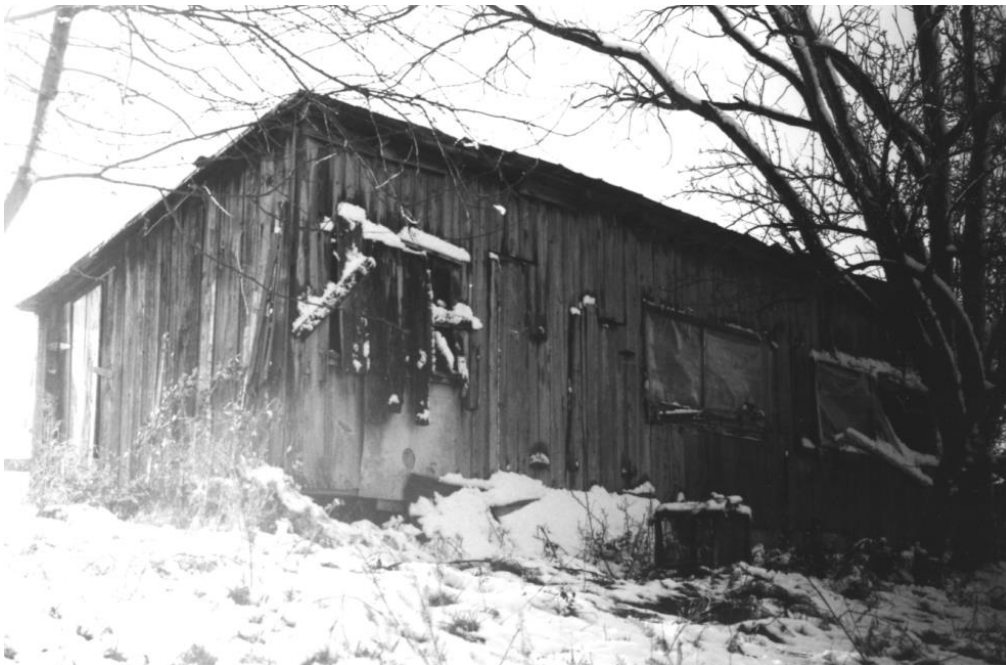
Figure 54: 1982 THC survey photo of BT-2328.
