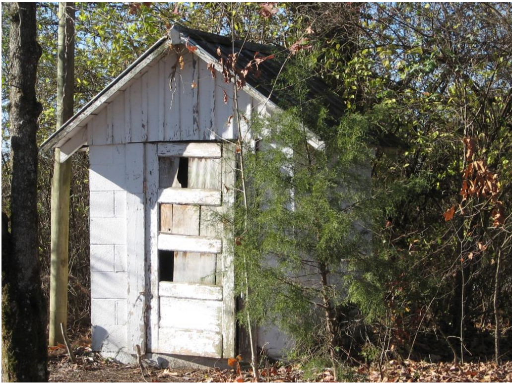
Figure 130: Site of BT-2244, pumphouse, view to the northwest.
