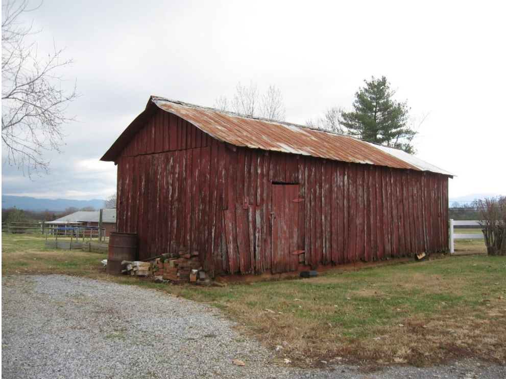
Figure 83: BT-2266, equipment shed, view to the southeast.
