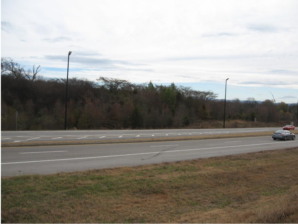
Figure 16: View to the southeast of the proposed right-of-way which will continue through the woods.
