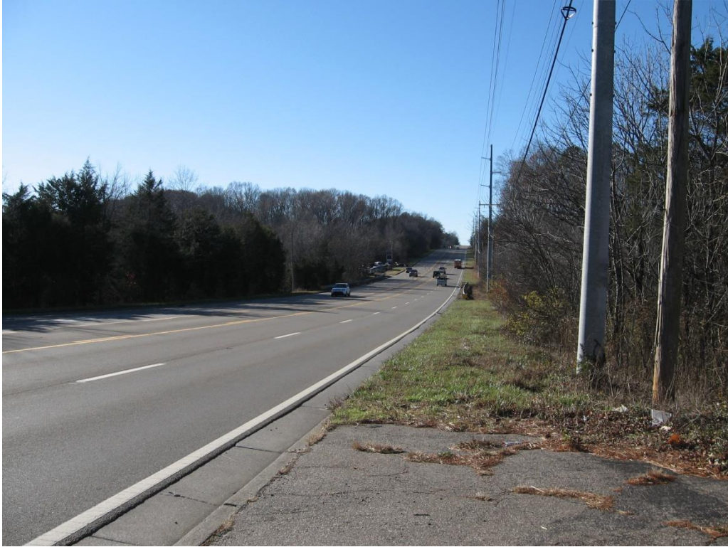
Figure 20: View to the west of the project's ending point at an interchange with SR-73 (Lamar Alexander Parkway/ U. S. 321).
