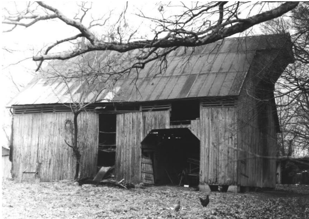
Figure 73: 1982 THC survey photo of BT-2307.
