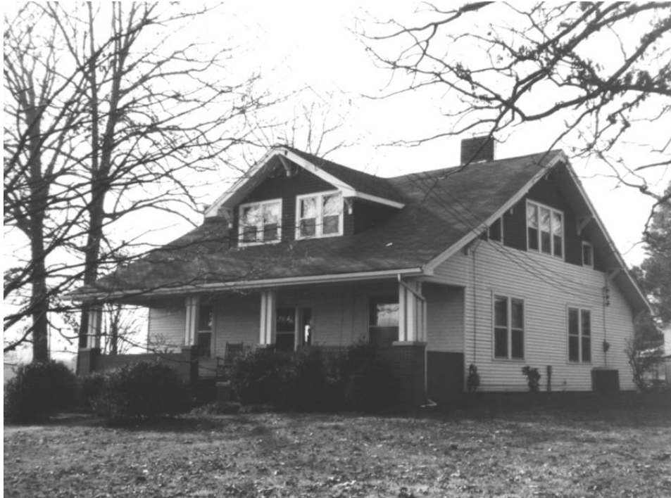
Figure 40: 1982 THC survey photo of BT-2586.
