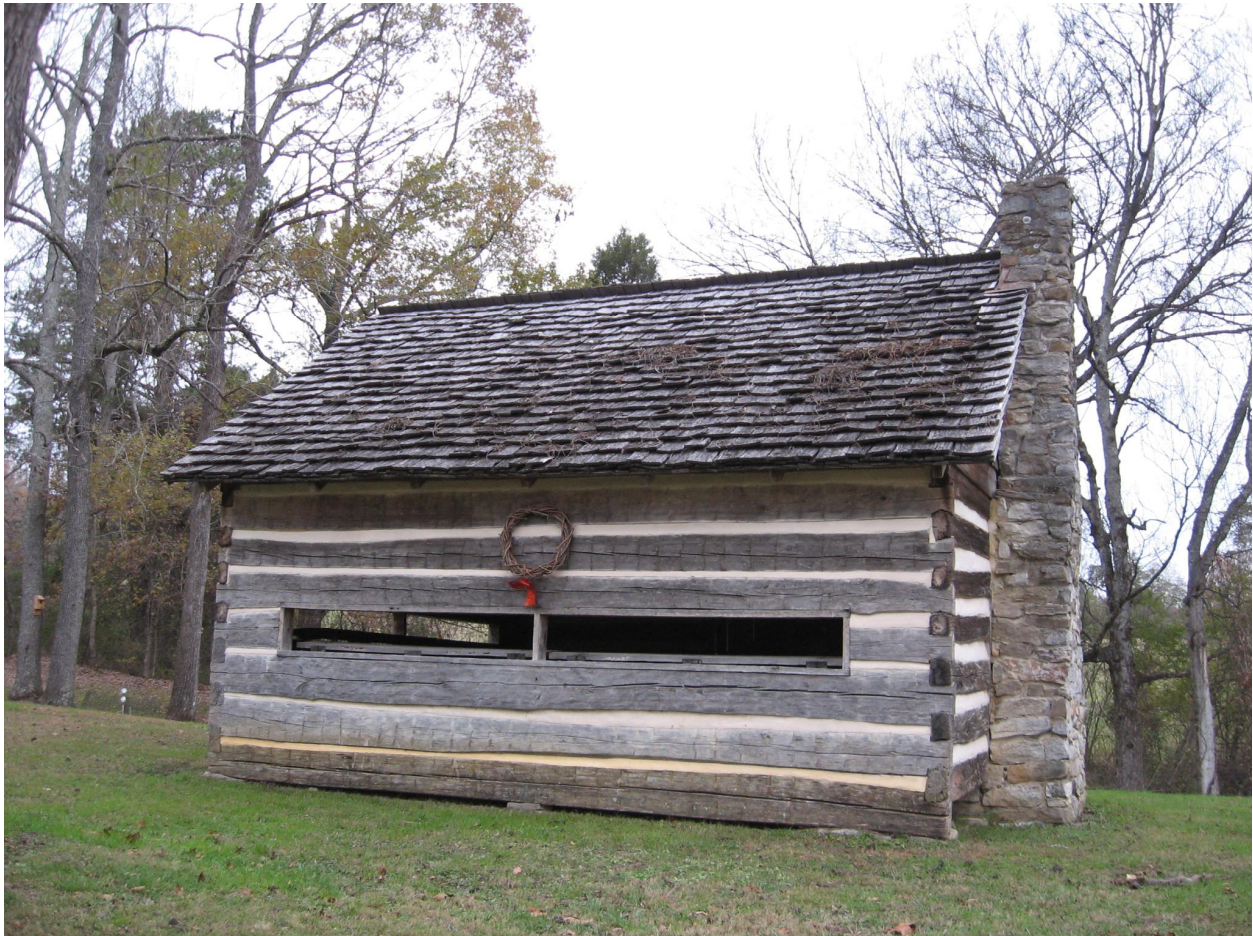
Figure 150: NR-listed Sam Houston School, view to the northeast.
