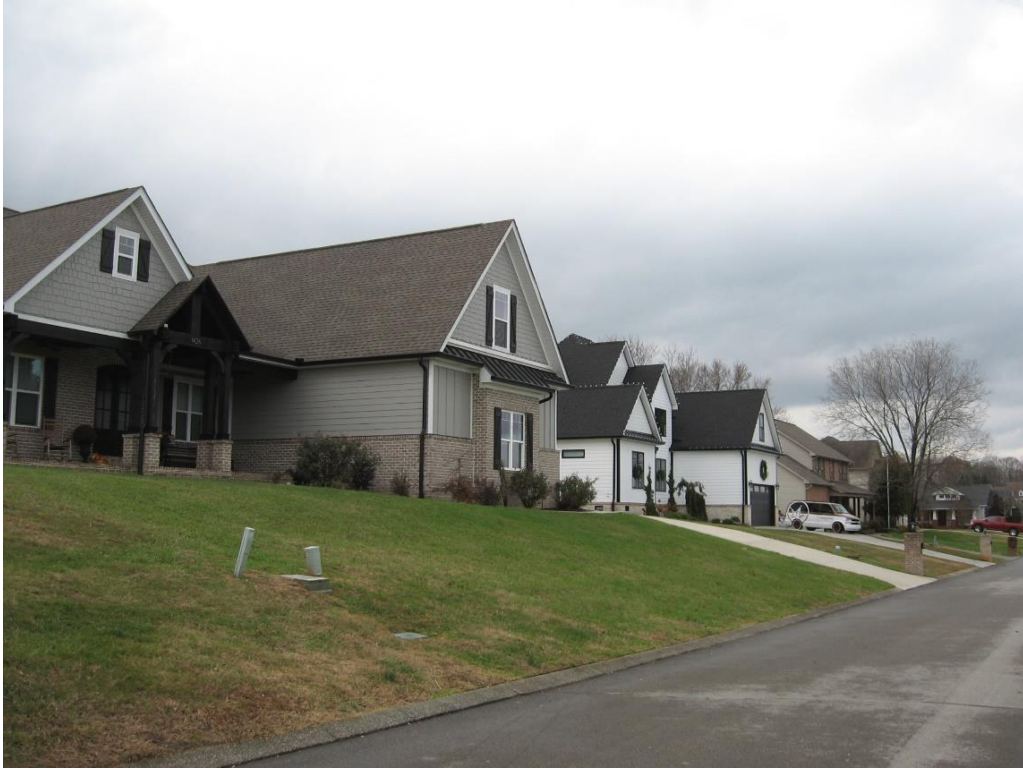
Figure 29: View southwest in the 1400 block of Crestridge Drive.
