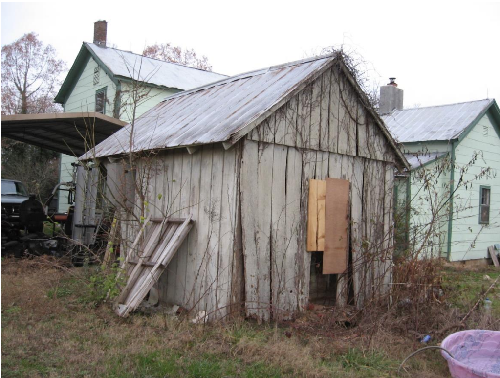
Figure 70: BT-2309 in 2022, view to the southwest.
