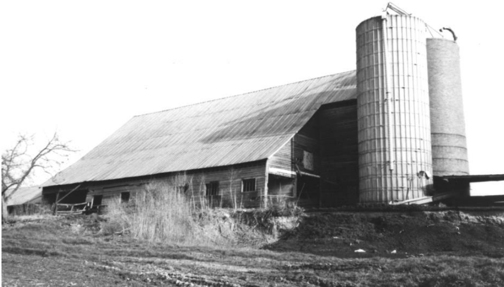
Figure 42: 1982 THC survey photo of BT-2587.
