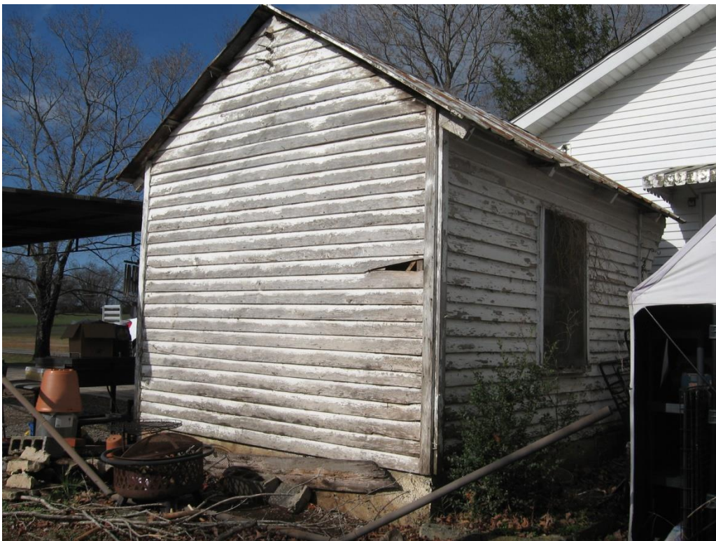
Figure 99: BT-2262 in 2022, view to the northwest.
