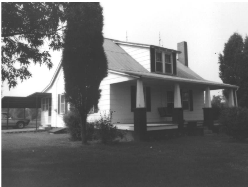
Figure 120: 1982 THC survey photo of BT-4601.
