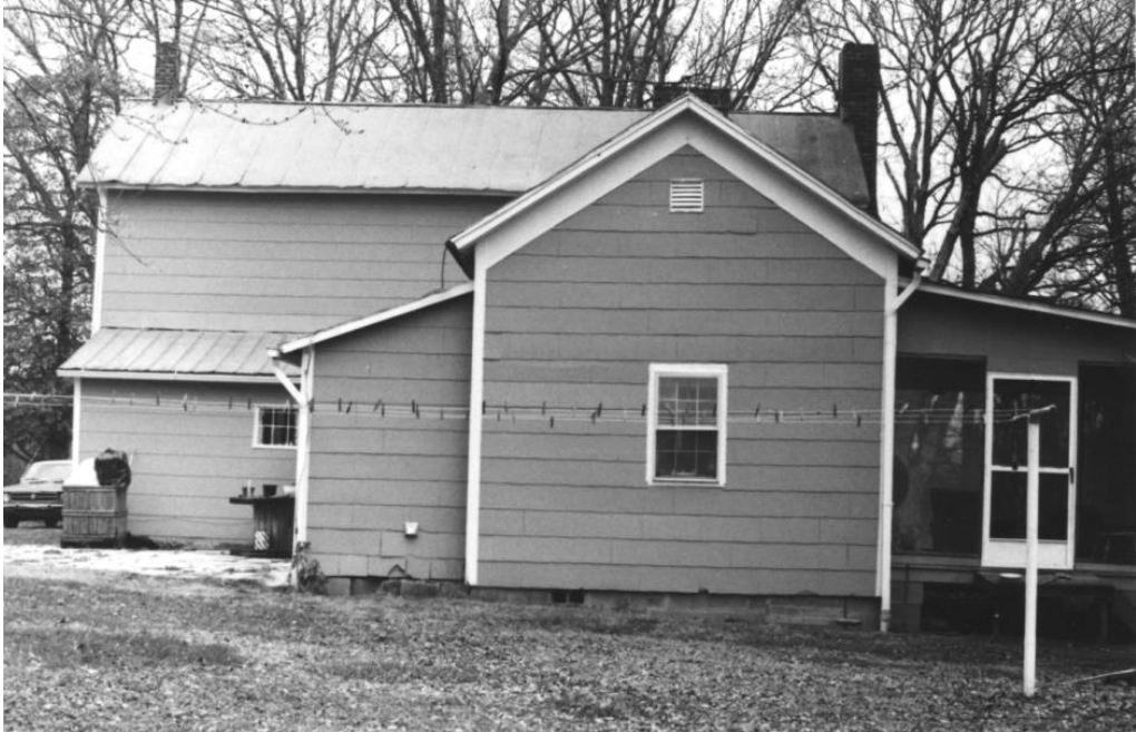
Figure 64: 1982 THC survey photo of BT-2300, rear elevation.
