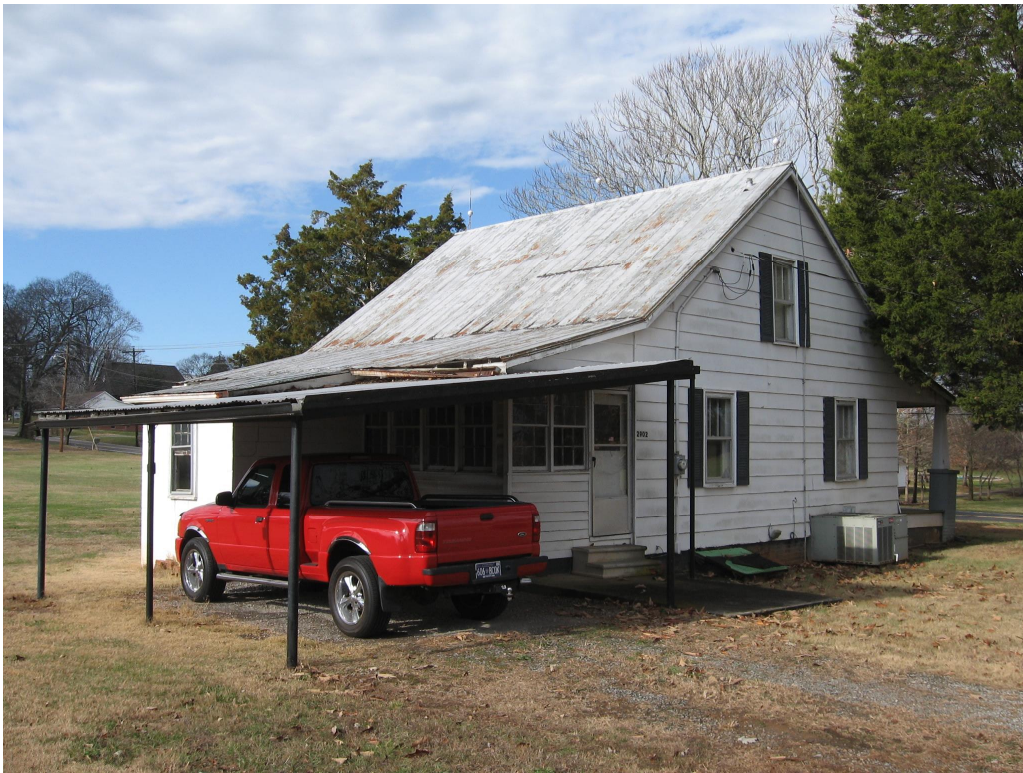
Figure 122: BT-4601 in 2022, view to the northwest.
