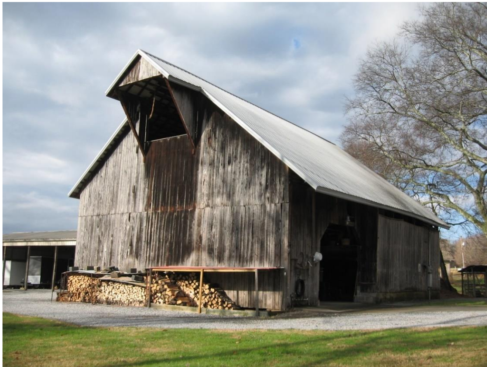
Figure 75: BT-2307 in 2022, view to the northwest.
