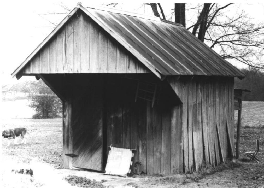
Figure 68: 1982 THC survey photo of BT-2301.
