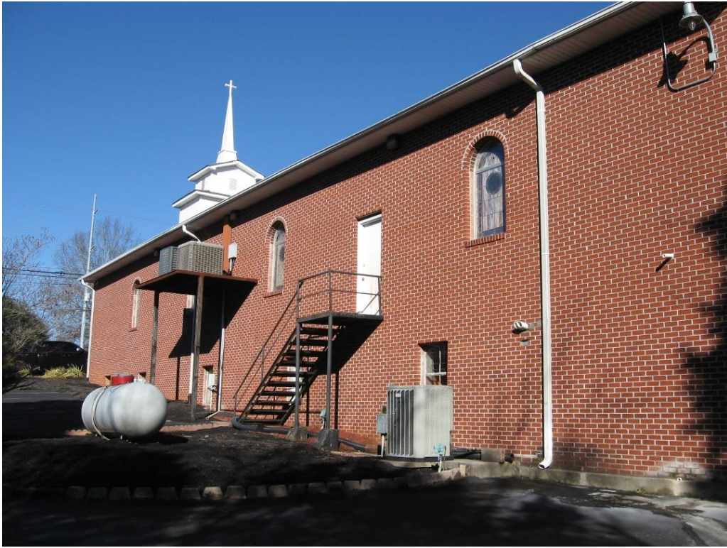
Figure 148: TA-2, View northeast
