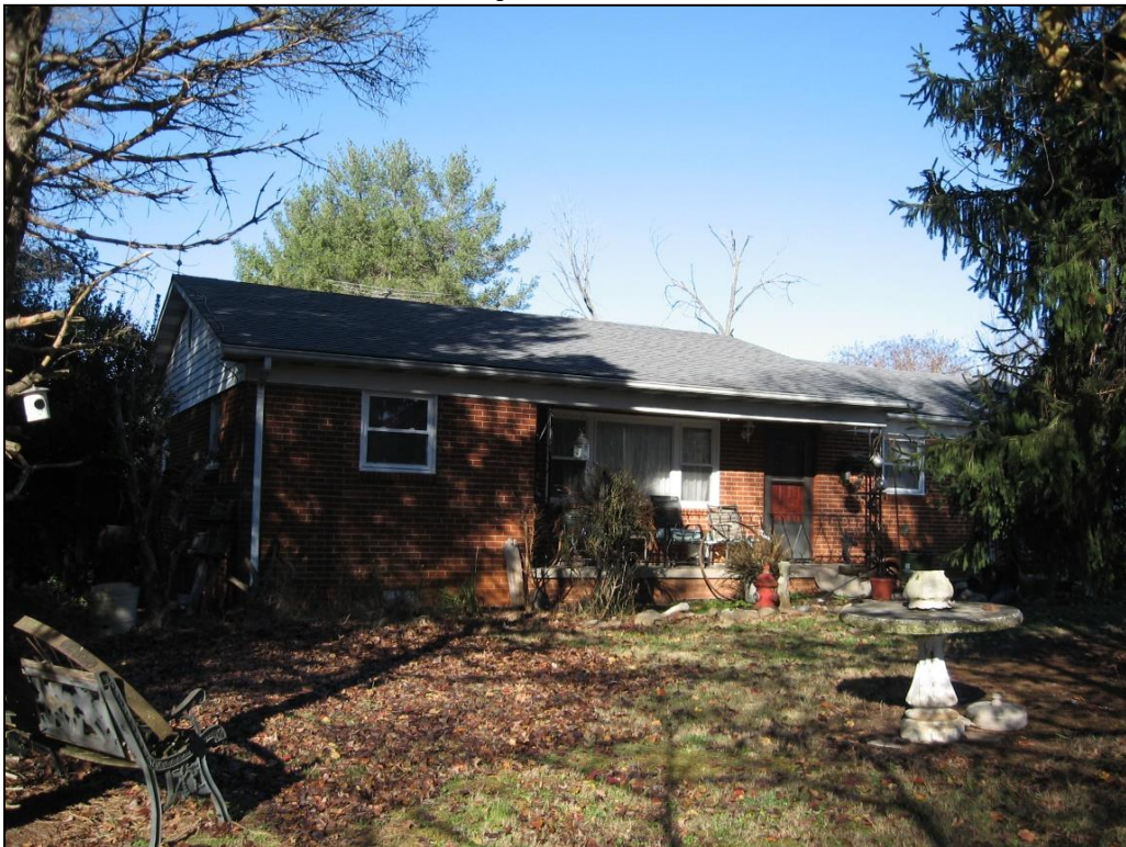
Figure 36: View northeast of 1960 brick Ranch dwelling at 3411 E. Lamar Alexander Parkway.
