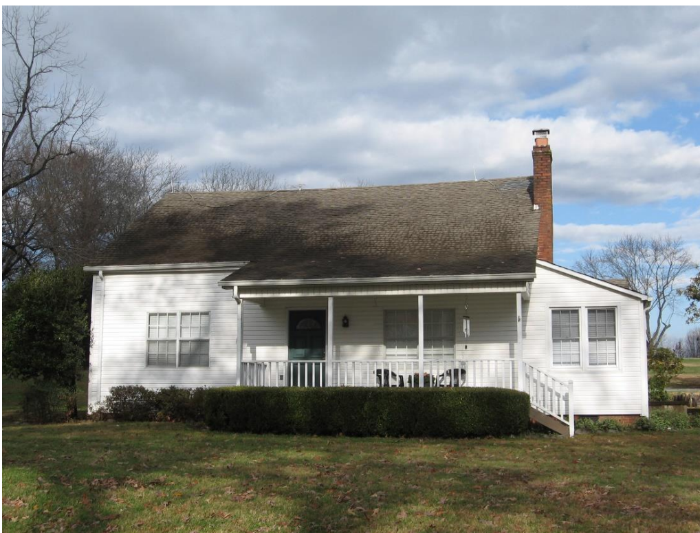
Figure 26: View north of a 1941 altered frame dwelling at 1735 E. Brown School Road.
