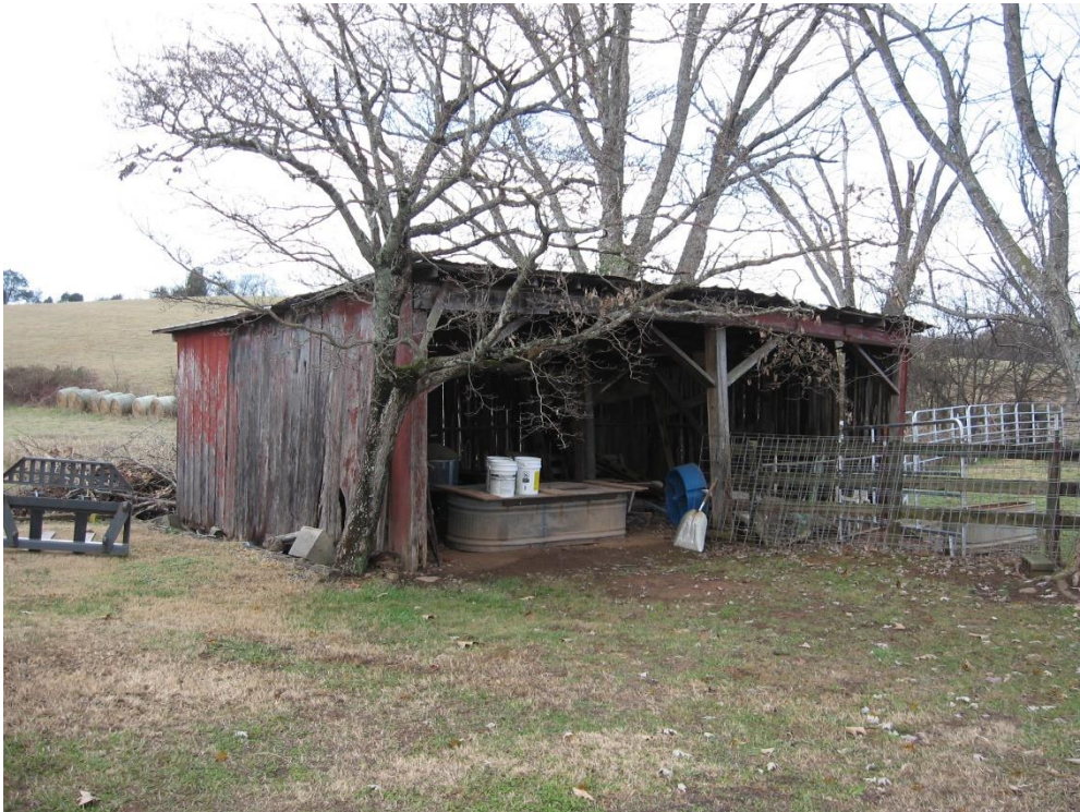
Figure 82: BT-2266, equipment shed, view to the southwest.
