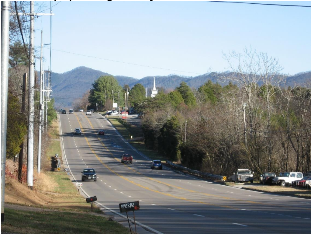
Figure 19: View to the east of the project's ending point at an interchange with SR-73 (Lamar Alexander Parkway/ U. S. 321).
