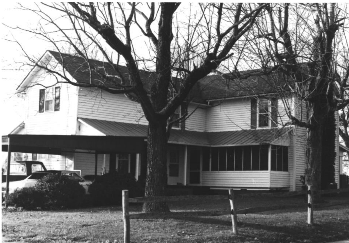
Figure 108: 1982 THC survey photo of BT-2240.
