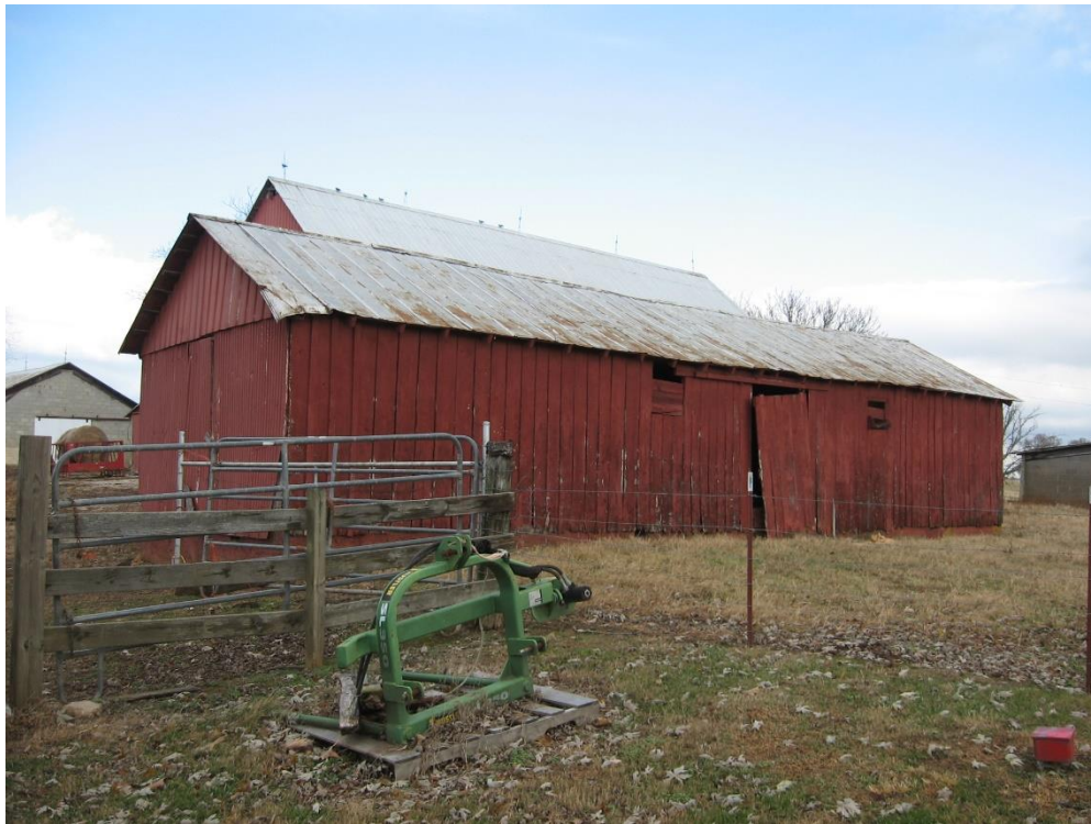
Figure 86: BT-2266, ca. 1940 frame barn, view to the northeast.
