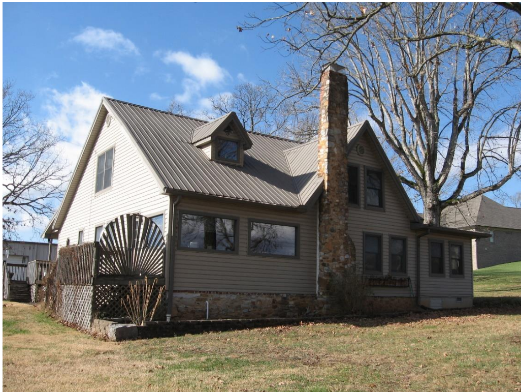
Figure 138: BT-2215 in 2022, view to the northwest.
