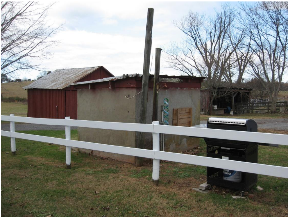
Figure 84: BT-2266, pump house, view to the northwest.
