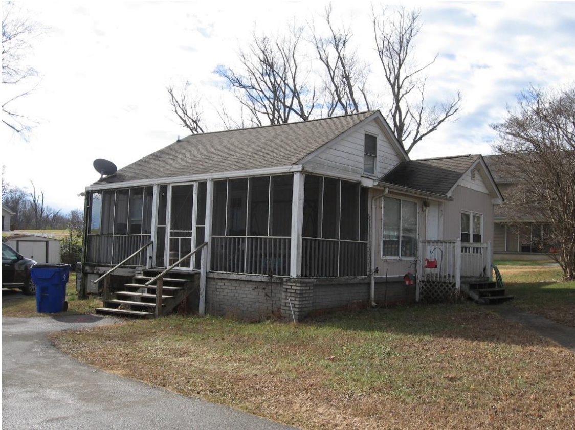
Figure 124: BT-4602 in 2022, view to the southwest.
