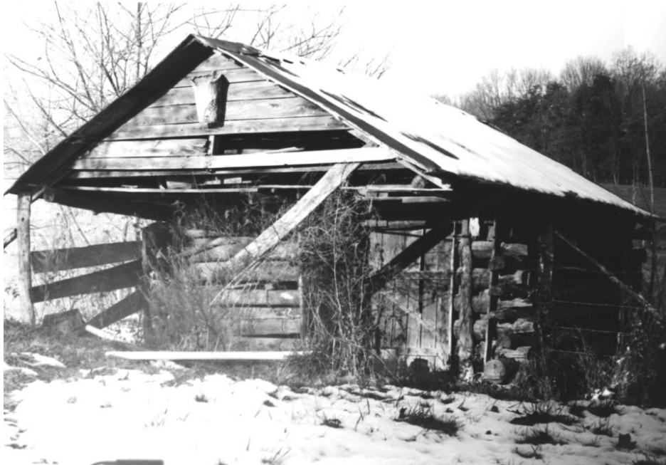
Figure 53: 1982 THC survey photo of BT-2327.
