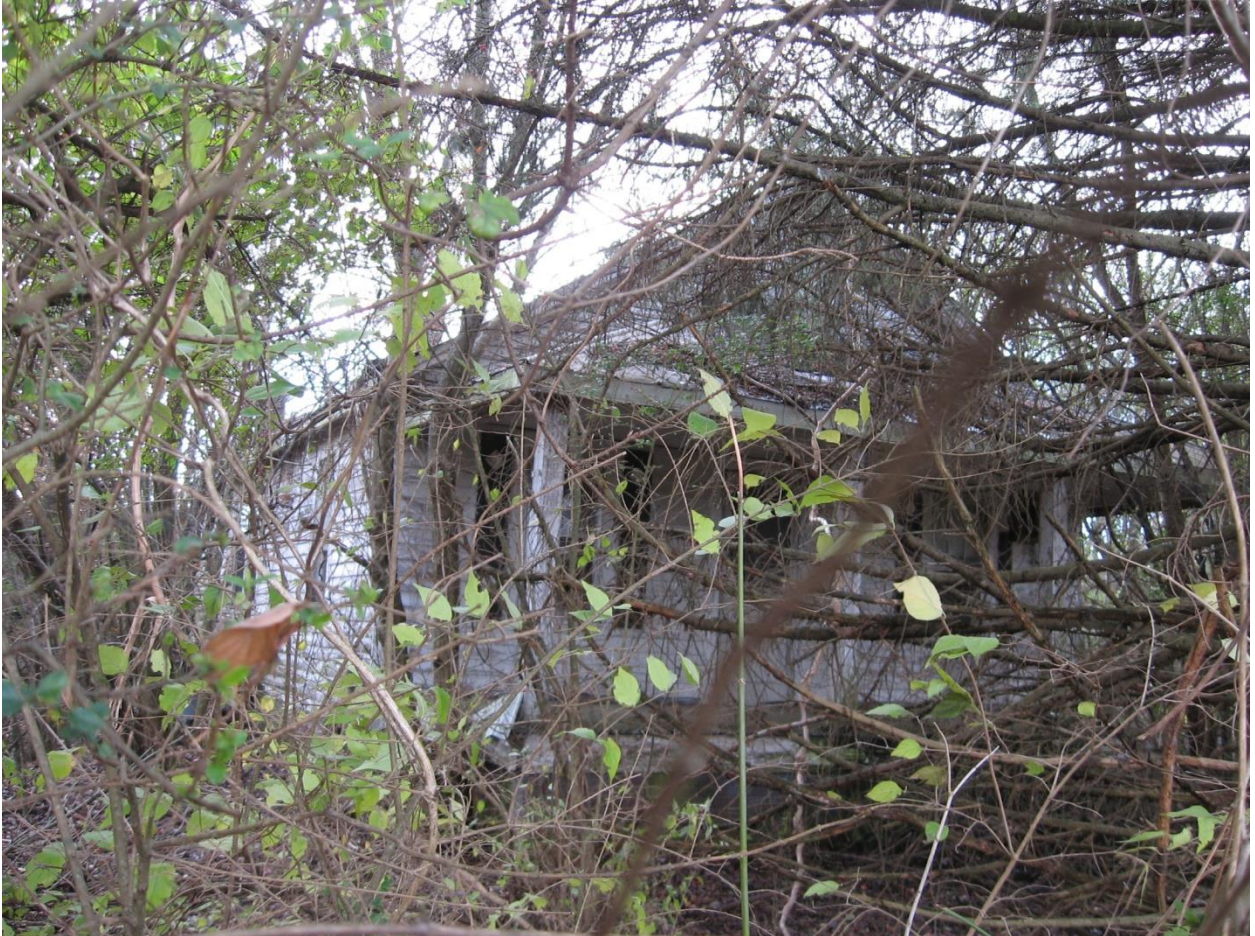
Figure 96: BT-2261, tenant house built in 1935, view southeast.
