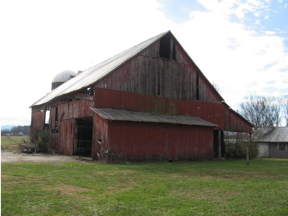
Figure 101: BT-2263 in 2022, view to the southwest.
