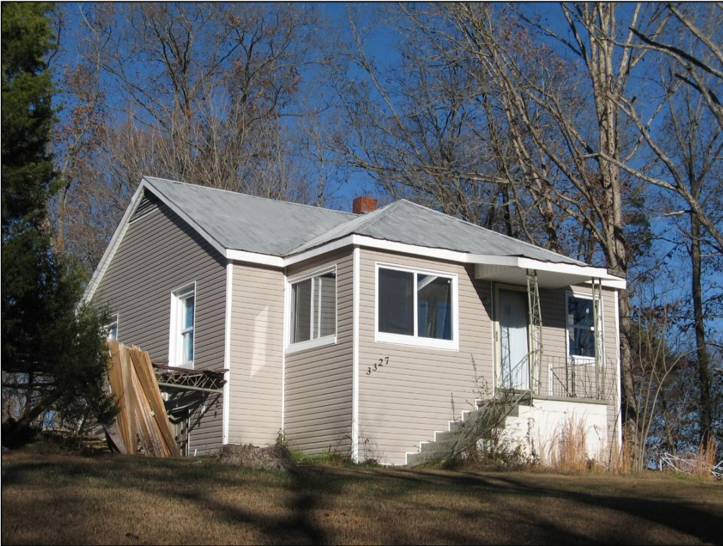
Figure 32: View northeast of an altered 1949 dwelling at 3327 E. Lamar Alexander Parkway.
