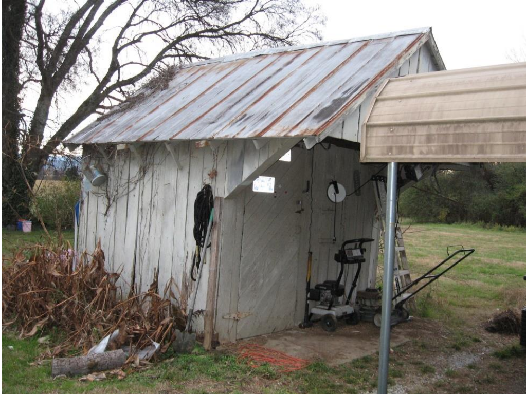
Figure 69: BT-2309 in 2022, view to the southwest.
