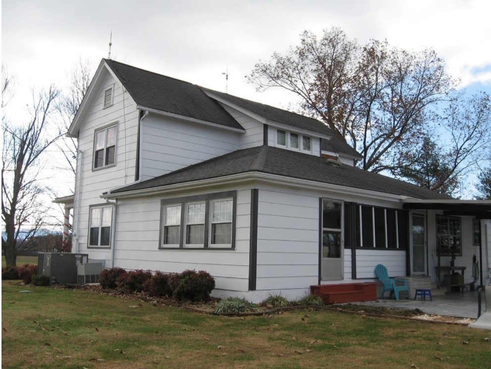
Figure 81: BT-2266 in 2022, view to the southwest.
