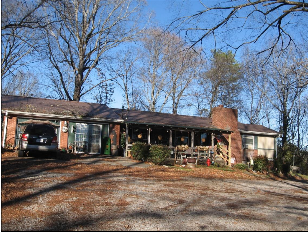
Figure 33: View northeast of an altered 1959 Ranch dwelling at 3335 E. Lamar Alexander Parkway.
