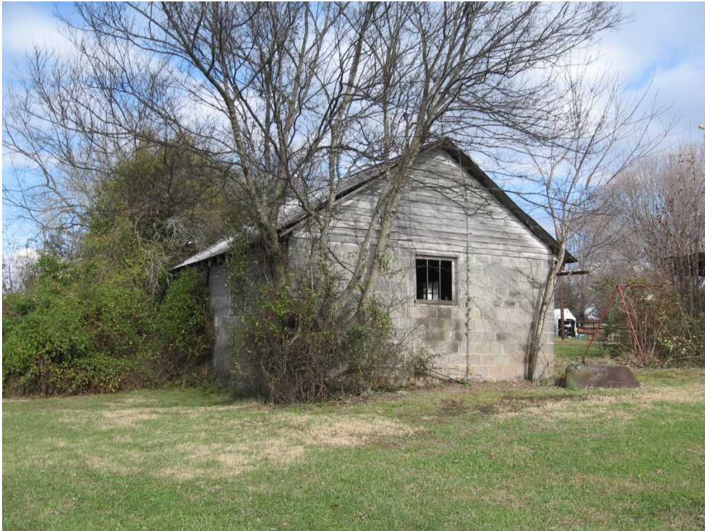
Figure 95: BT-2261, concrete block dairy building, view to the north.
