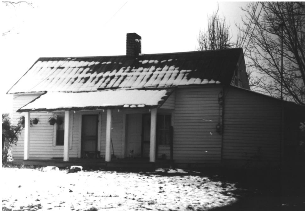
Figure 51: 1982 THC survey photo of BT-2326.
