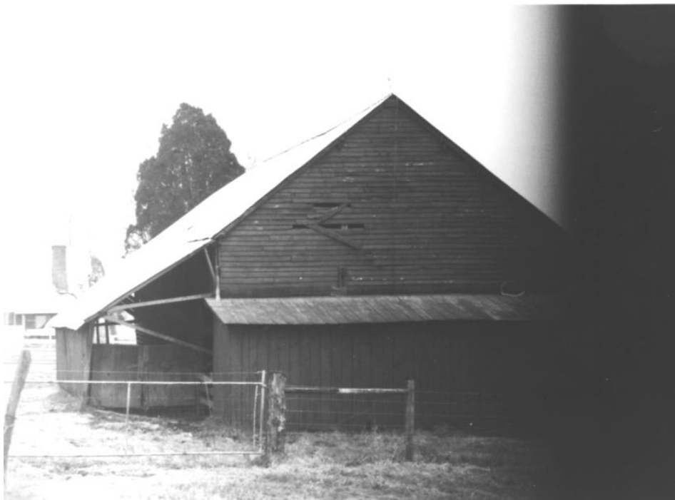
Figure 87: 1982 THC survey photo of BT-2267.
