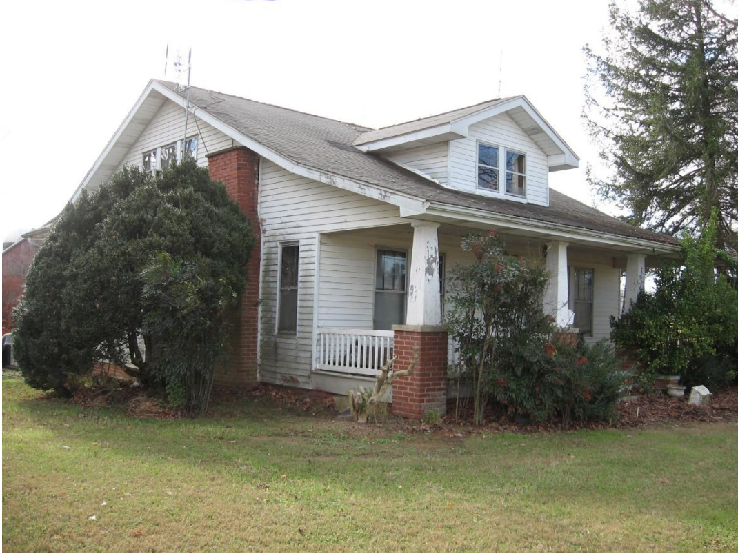
Figure 92: BT-2261 in 2022, view to the southwest.
