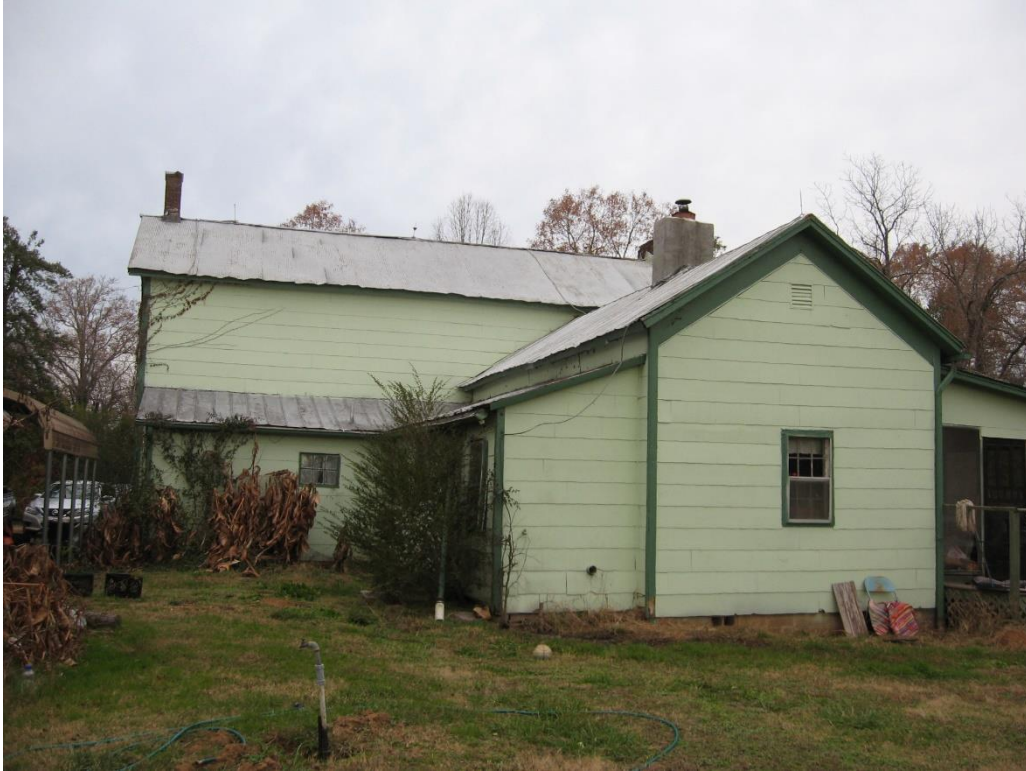
Figure 66: BT-2300 in 2022, view to the north.
