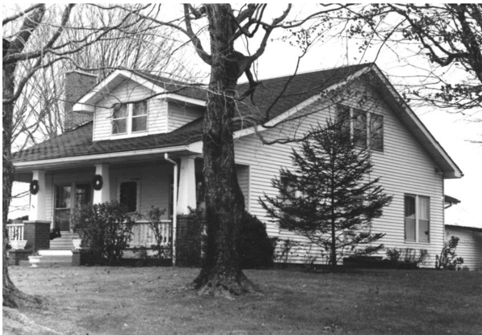
Figure 90: 1982 THC survey photo of BT-2261.
