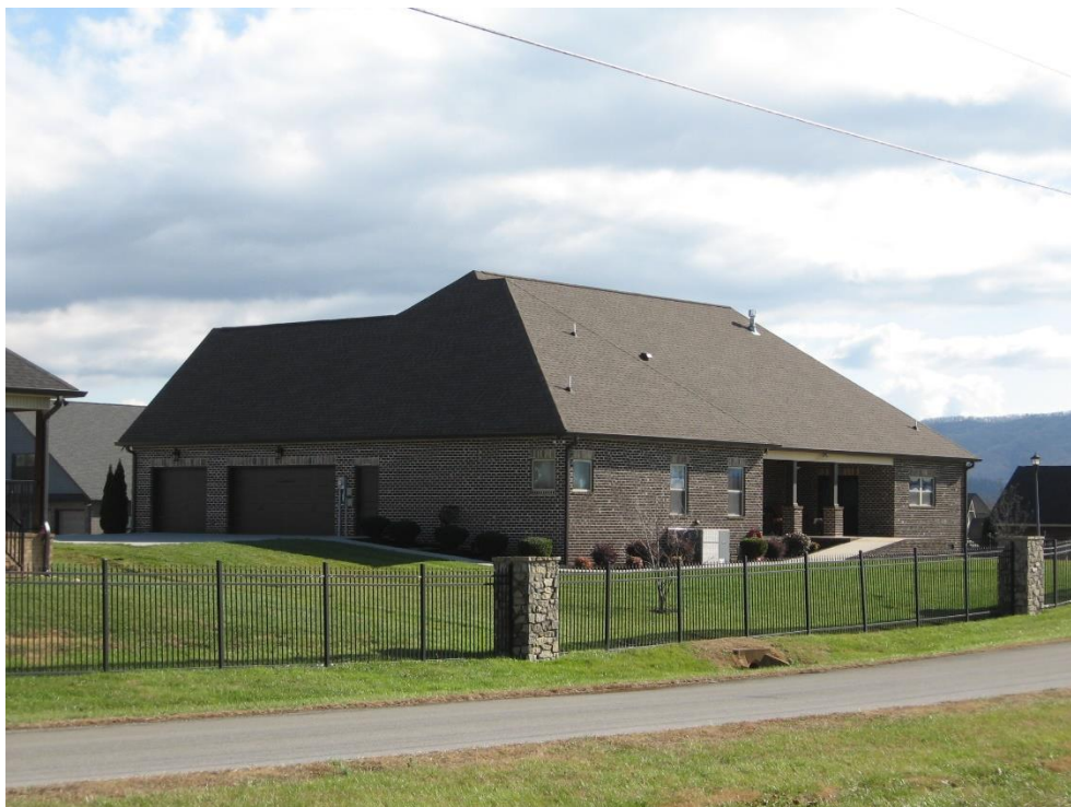
Figure 144: Site of BT-2217, view southeast.
