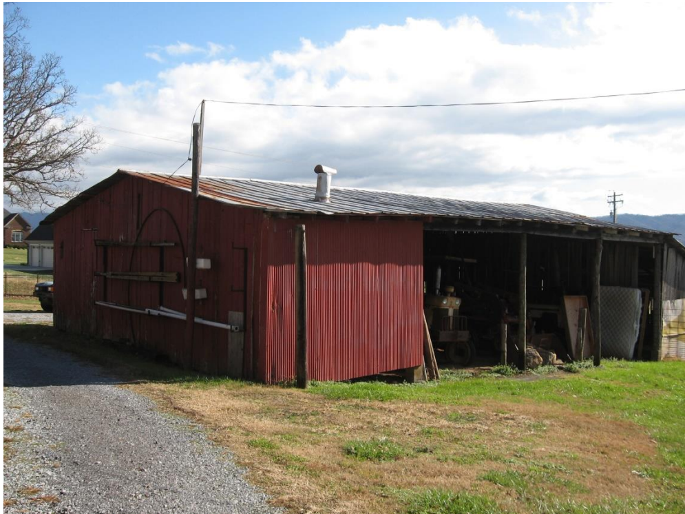
Figure 142: BT-2215, equipment shed, view to the southeast.
