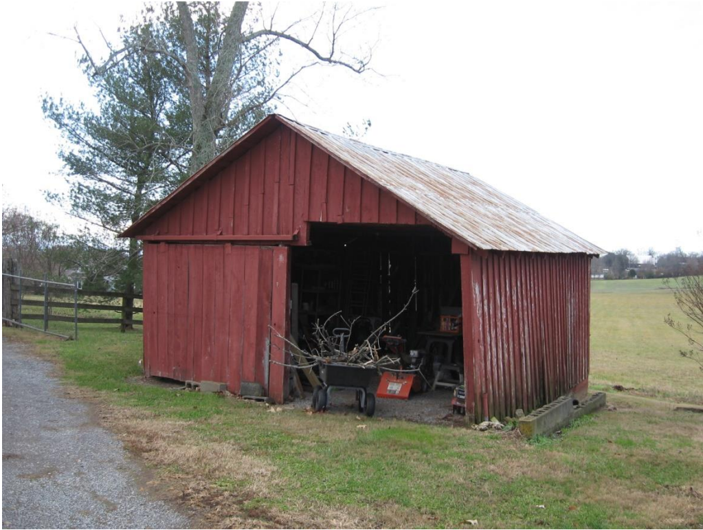
Figure 85: BT-2266, garage, view to the southwest.
