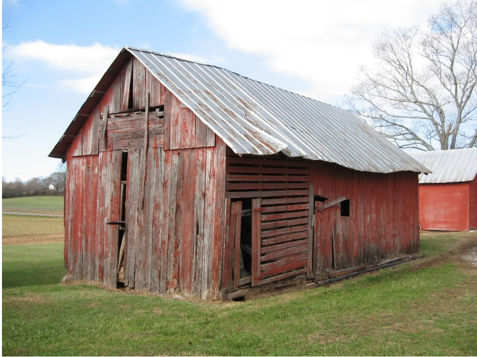
Figure 104: BT-2264 in 2022, view to the northwest.
