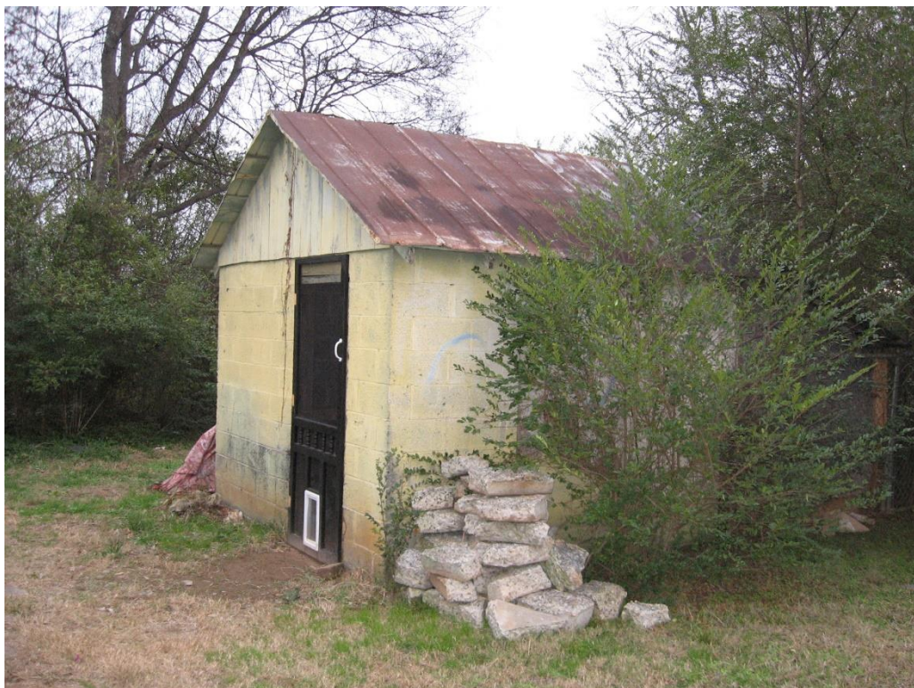
Figure 67: BT-2300 in 2022, pump house, view to the southeast.
