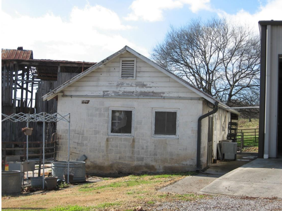
Figure 141: BT-2215, dairy building, view to the west.
