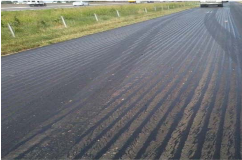
Improper Tack Coat, Zebra Strip/Corn Rows. Unacceptable.
