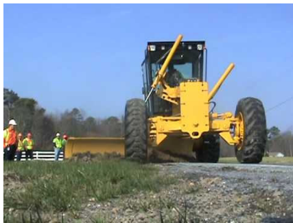
Clipping the shoulder with a motor grader
