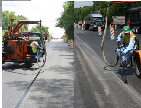
Overbending longitudinal joints 4" wide with PG binder
