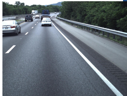
Shoulder only partially overlaid with OGFC
