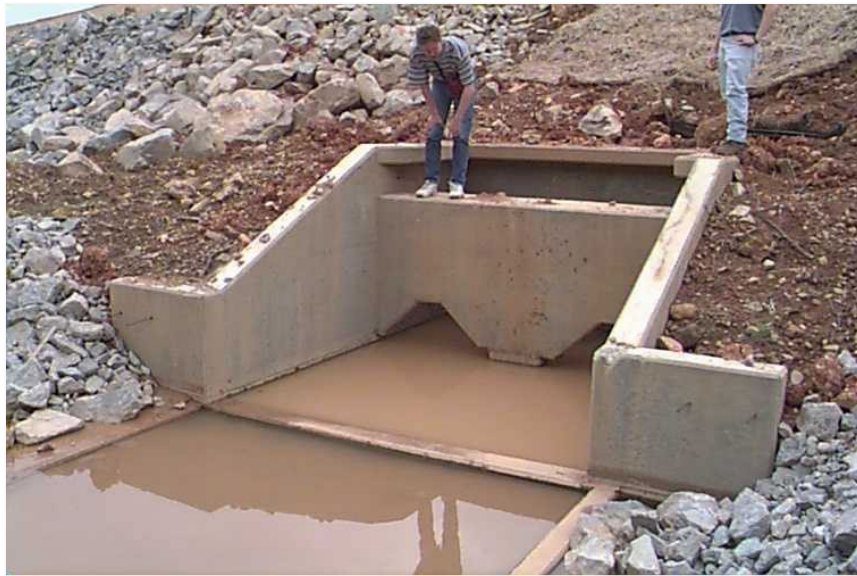
Figure 9-6: Typical USBR Type VI Baffled Dissipator
