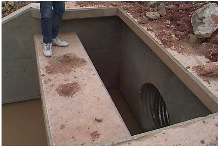
Figure 9-7: Top of the Baffle in a USBR Type VI Energy Dissipator
