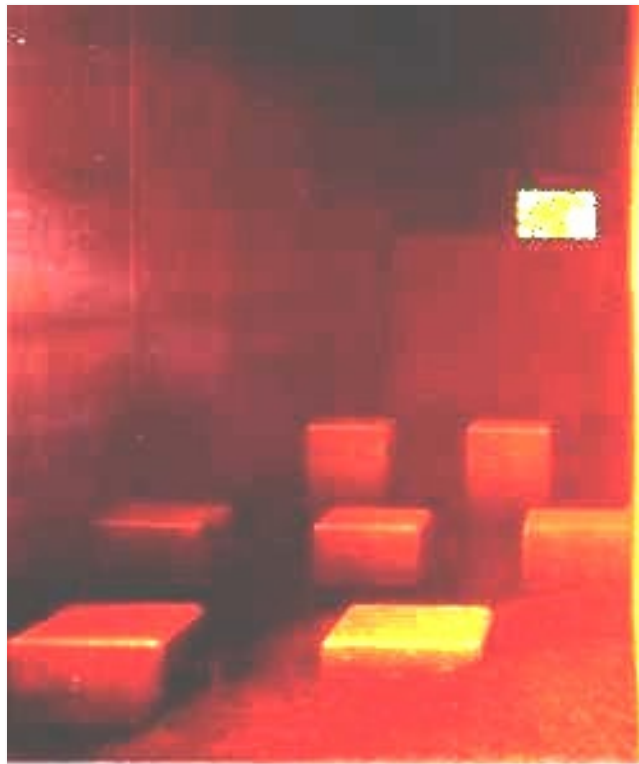
Figure 9-3: Roughness Elements Inside of a Box Culvert
