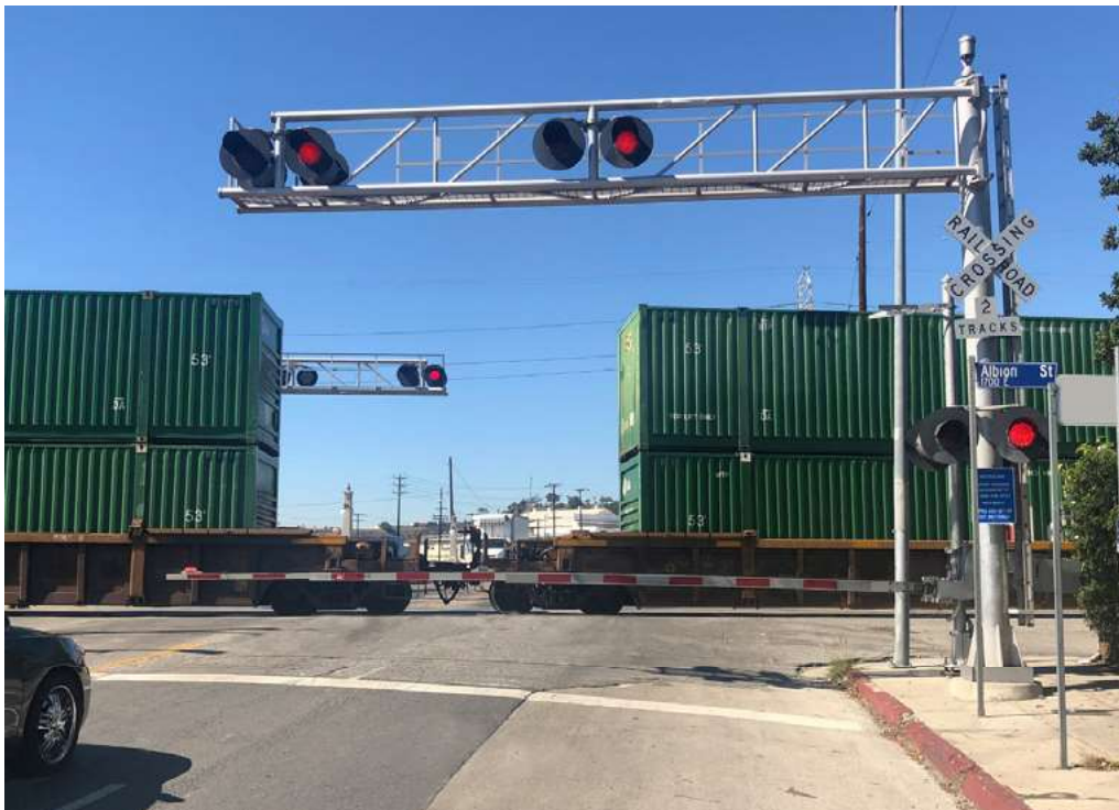
Figure 21. Illustrative Example Showing Cantilever with Flashing-Light Devices
