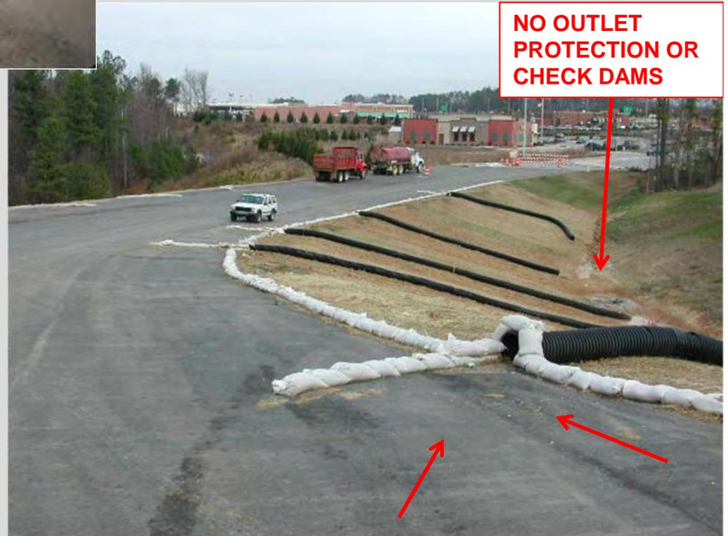
Super elevated road sections diverted into slope drains
