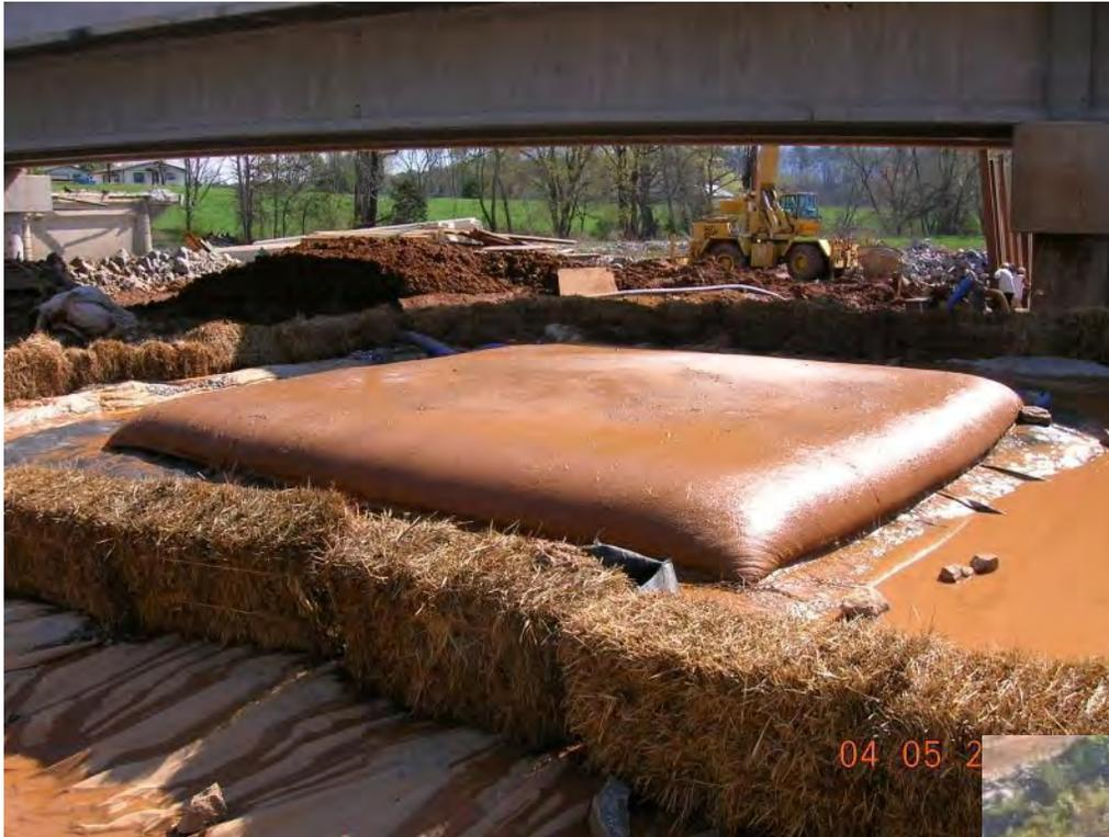
Sediment filter bags are not designed to remove fine sediments or control turbid water
