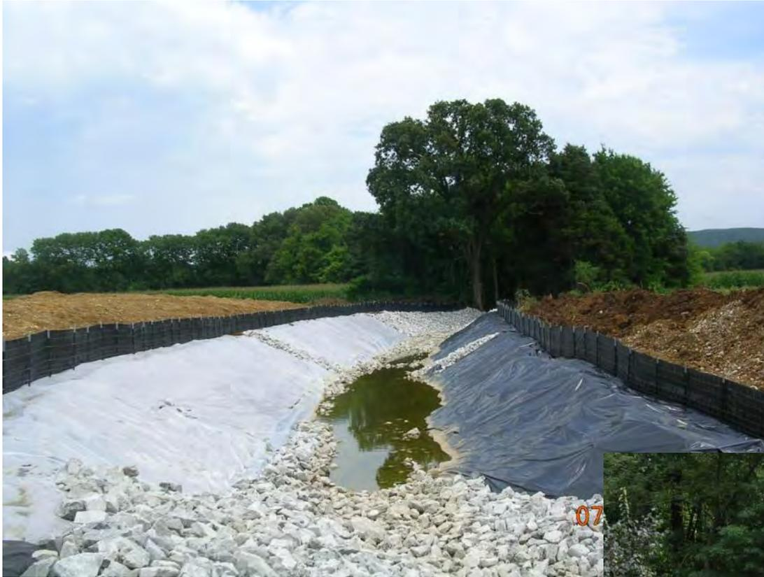
Temporary stream diversion and crossing to construct a box culvert.
