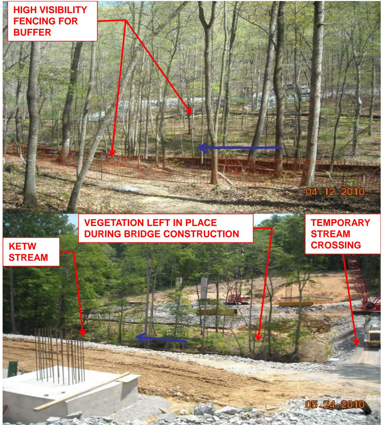
Vegetated buffer and equivalent measures along a temporary stream crossing
