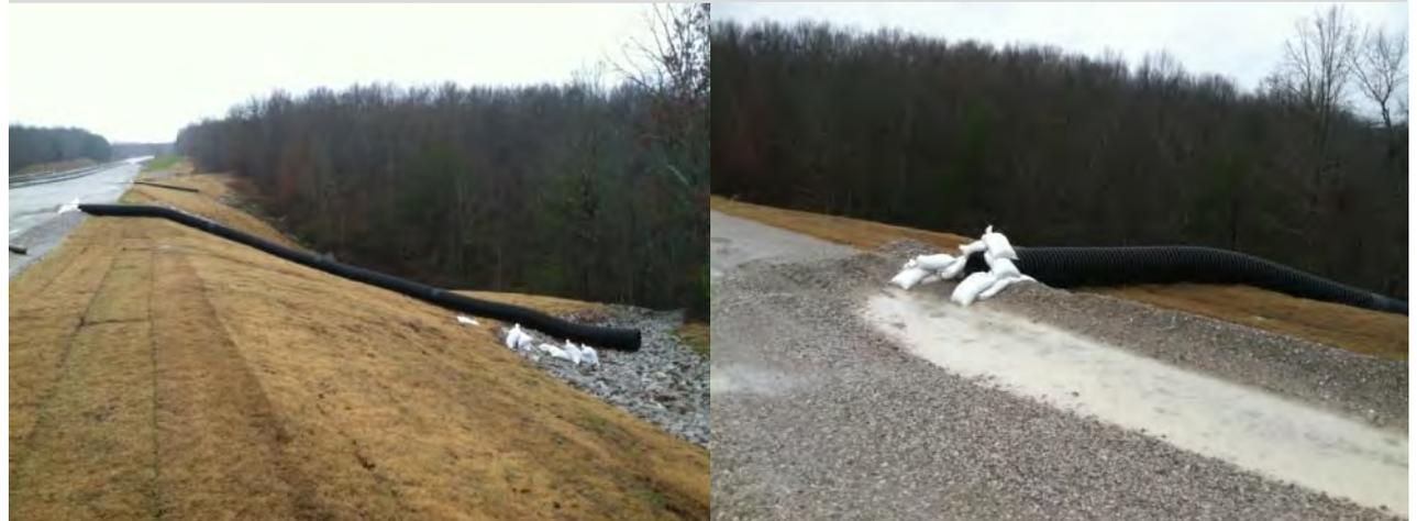
Slope drain without outlet protection
