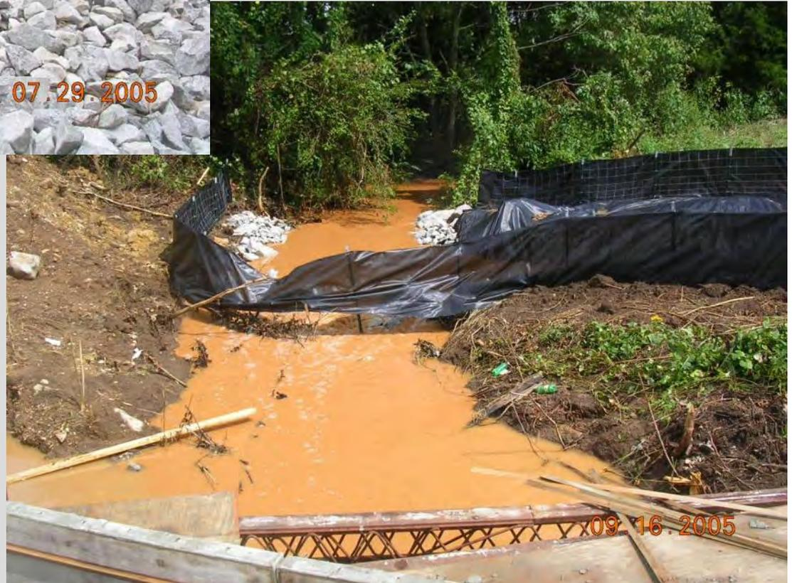
Verify that the channel lining specified in the stream diversion can handle the velocities during the design storm event.
