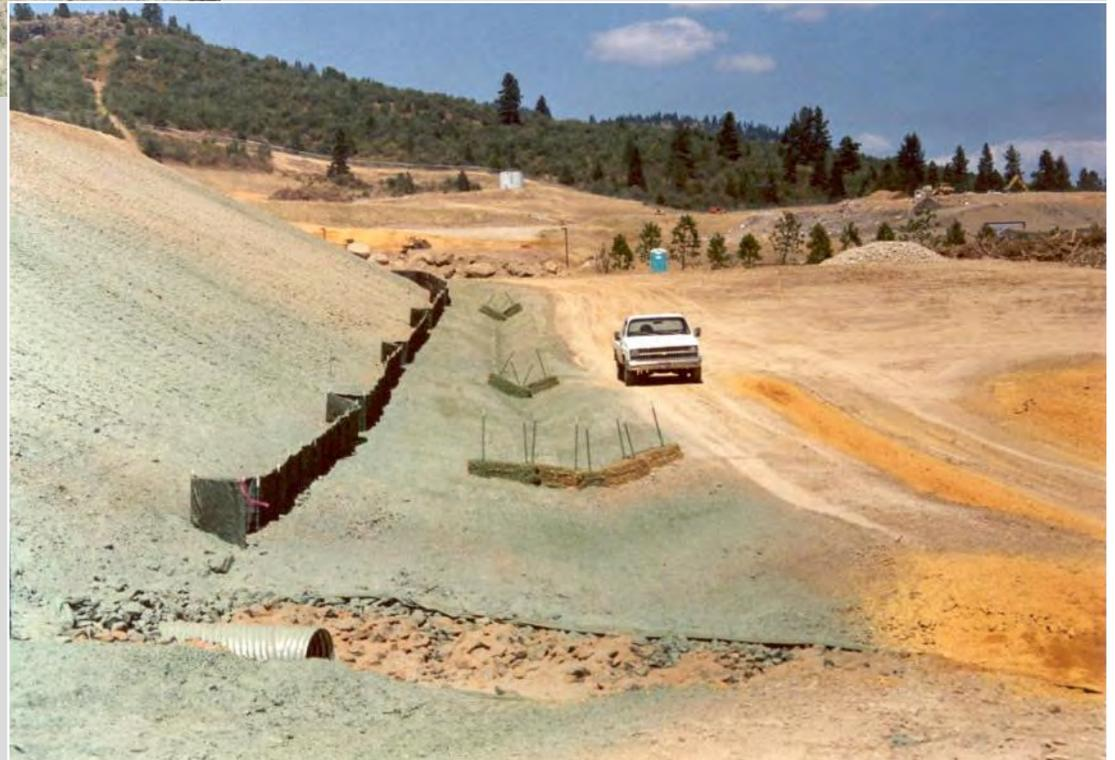
Silt fence shouldn't be depicted perpendicular to contours. No outlet provided at low point in silt fence at toe of slope resulting in silt fence being overtopped during storm event
