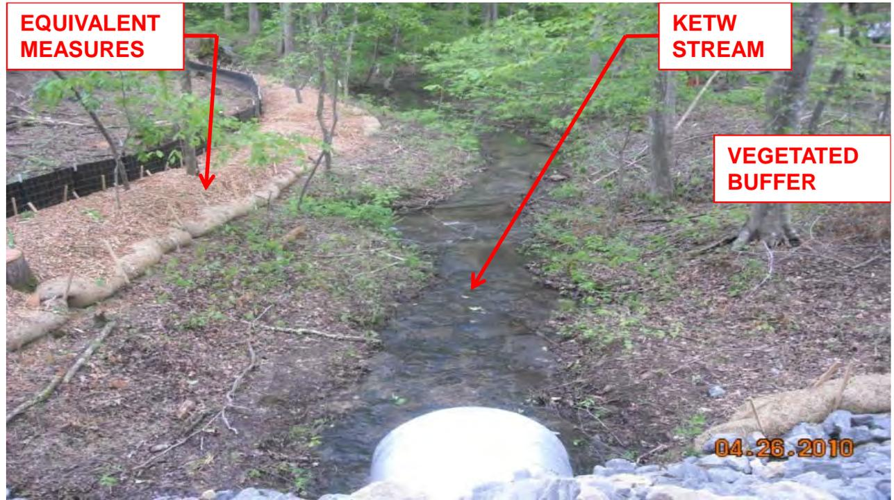
Vegetative buffer left in place during bridge construction
