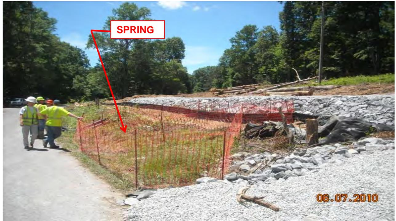
High visibility fencing identifying clearing limits and buffer zone adjacent to a wetland
