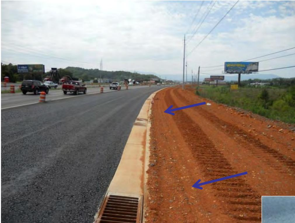
Curb inlet protection Type 1-4 needed to protect inlets from sediment
