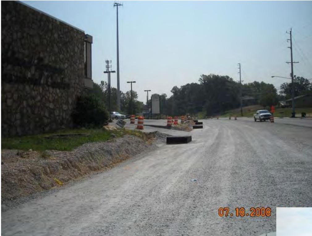
Catch basin filter assemblies placed over curb inlets during different phases of construction
