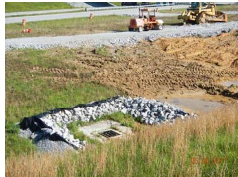
**Closed Drainage System Inlets - Last Place to Capture Sediment**
