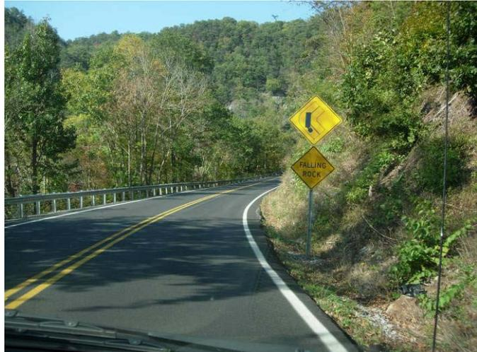
New pavement marking, guardrail and advanced warning signs approaching 15 mph curve (2009)
