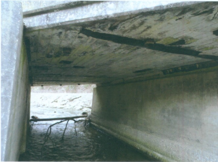
VIEW UNDER THE DECK
