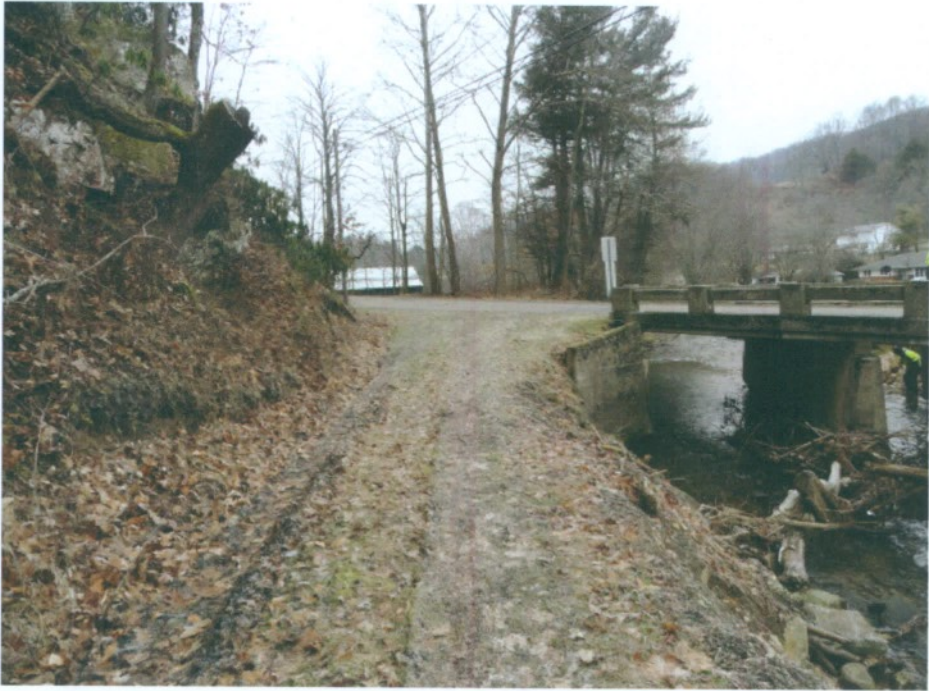
VEHICLE ACCESS TO REC BUILDING (LOOKING NORTH)
