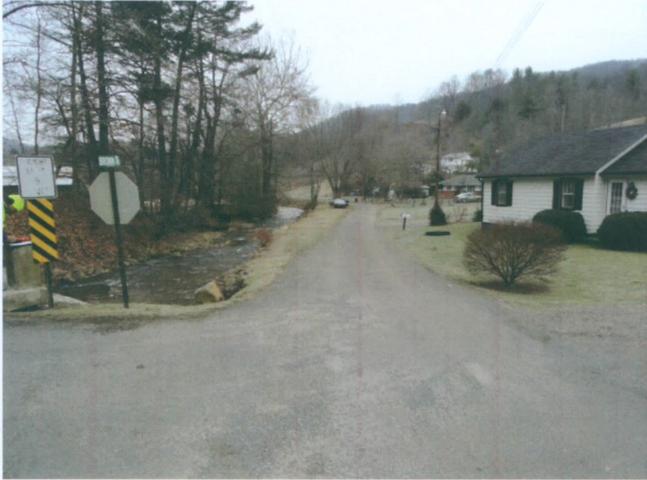
BROWN ROAD (LOOKING NORTH)
