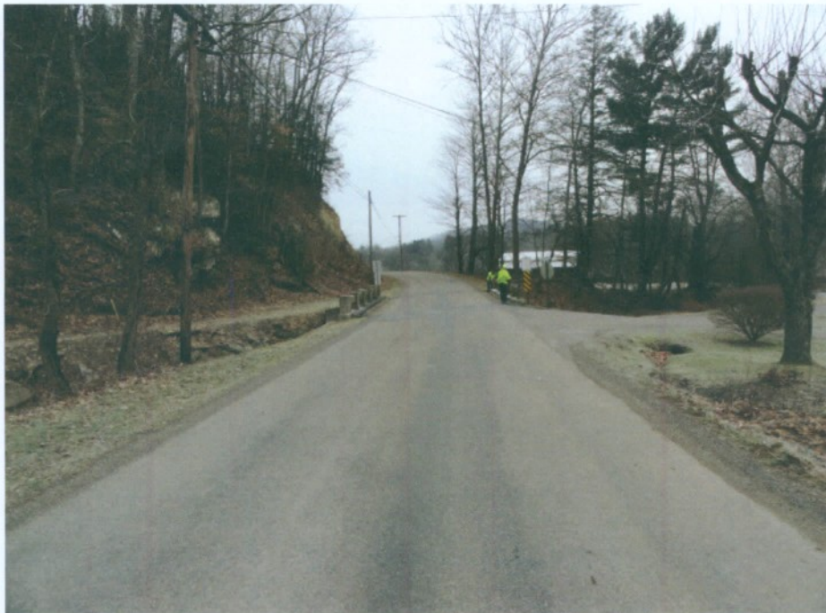
WESTBOUND APPROACH (LOOKING EAST)
