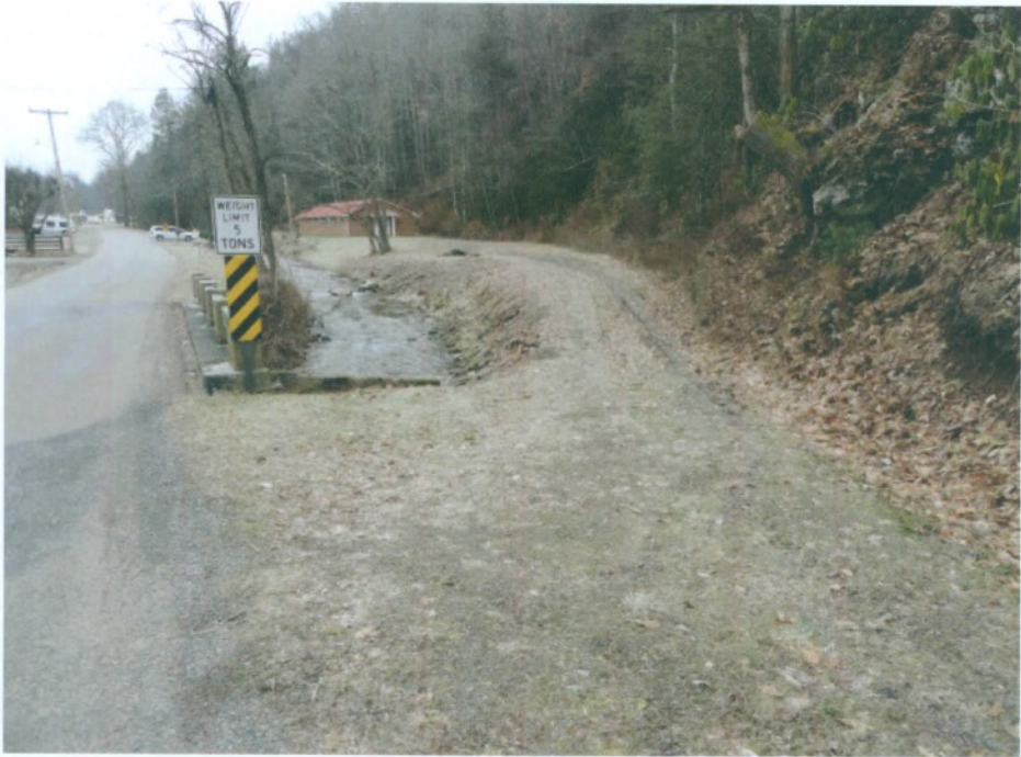
VEHICLE ACCESS TO REC BUILDING (LOOKING SOUTH)
