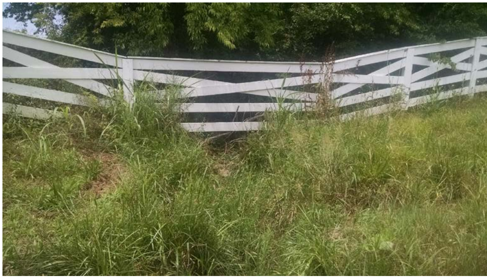
Photo 8. STR-2 u/s of Saturn Pkwy looking West. 35.7429, -86.9489
