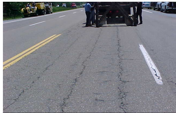
Extensive cracking from oxidized pavement, no structural damage
