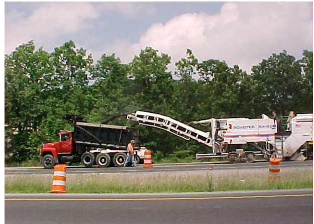
Milling machine in operation
