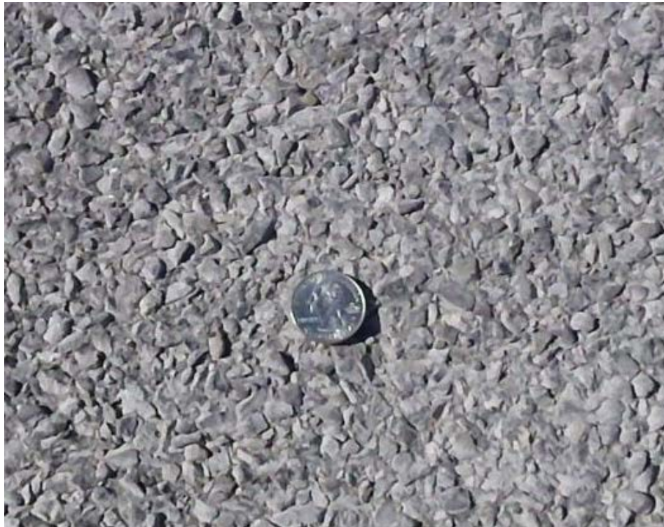
Chip Seal prior to Thin Lift of Hot Mix Asphalt being placed
