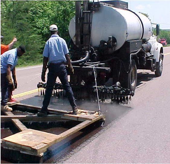
Application of asphalt sealer
