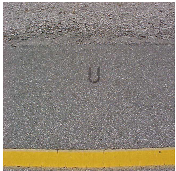
Under-drain location needs remarking
