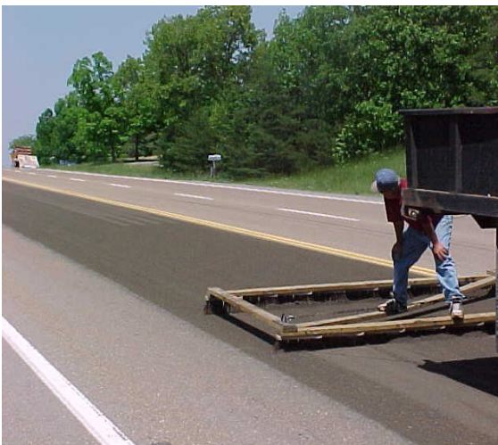
Brooming of aggregate cover material
