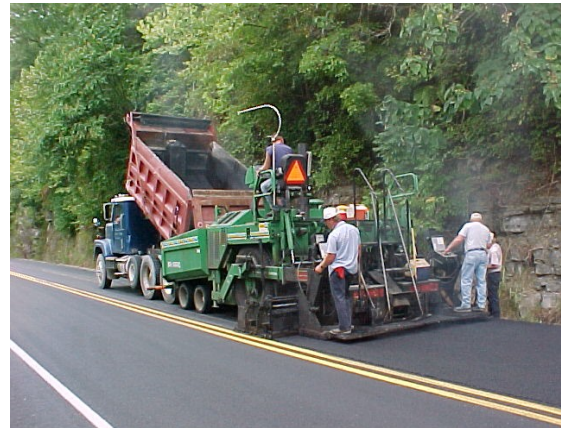
Placement of "B-M" Mix at 1\text{-}1/2"
