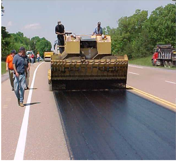
Aggregate applied to asphalt sealer
