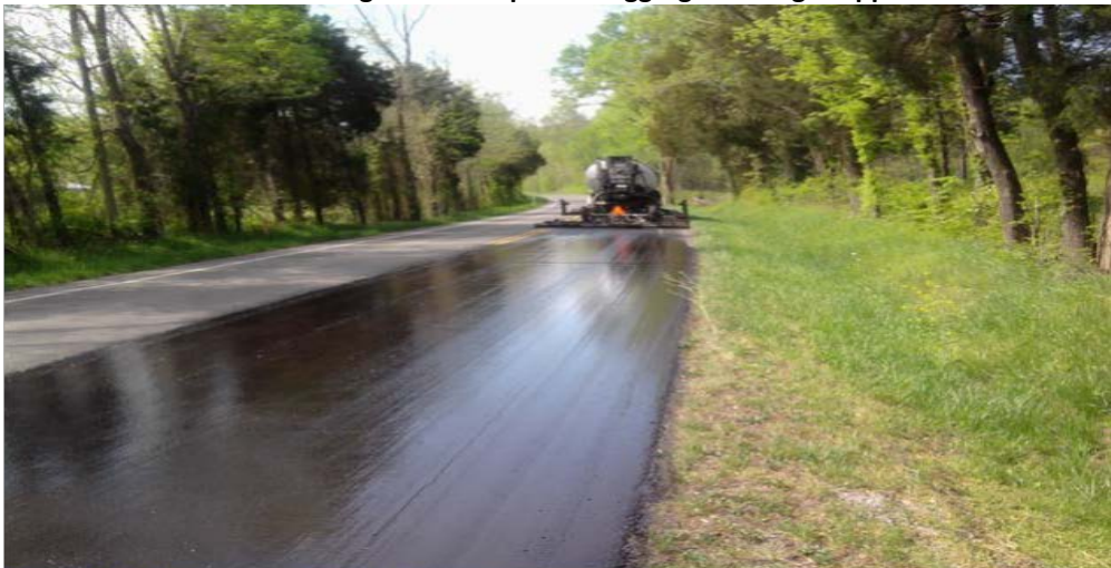
CRS2P Emulsion filling the cracks prior to aggregate being dropped
