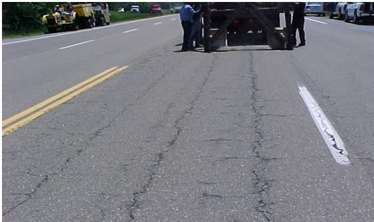
Extensive cracking from oxidized pavement, no structural damage
