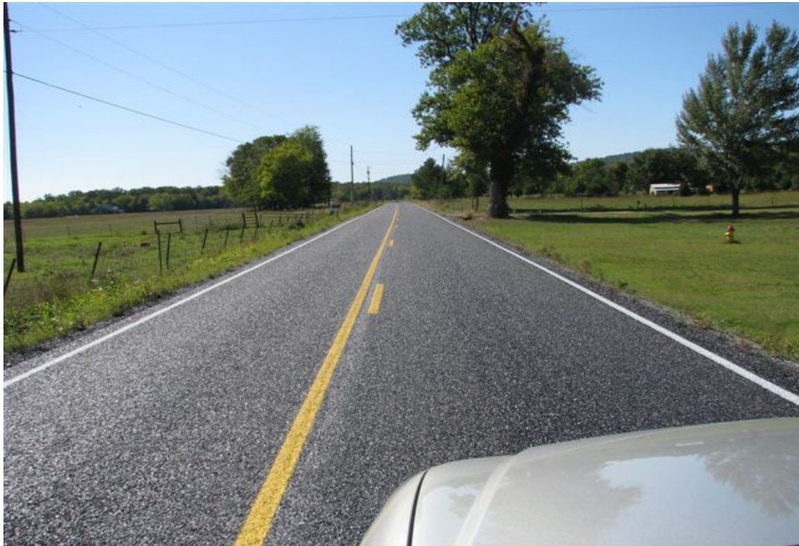
Completed Chip Seal w/ Fog Seal
