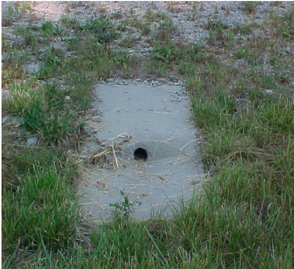
End wall properly functioning
