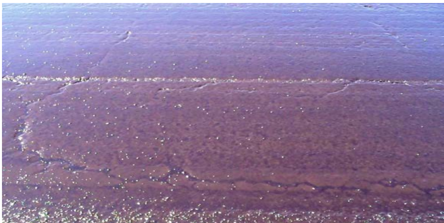
CRS2P Emulsion filling the cracks prior to aggregate being dropped
