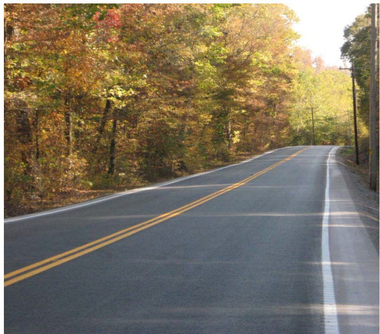
Completed Chip Seal with Thin Overlay
