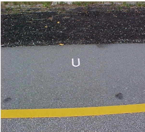
Under-drain marked on shoulder
