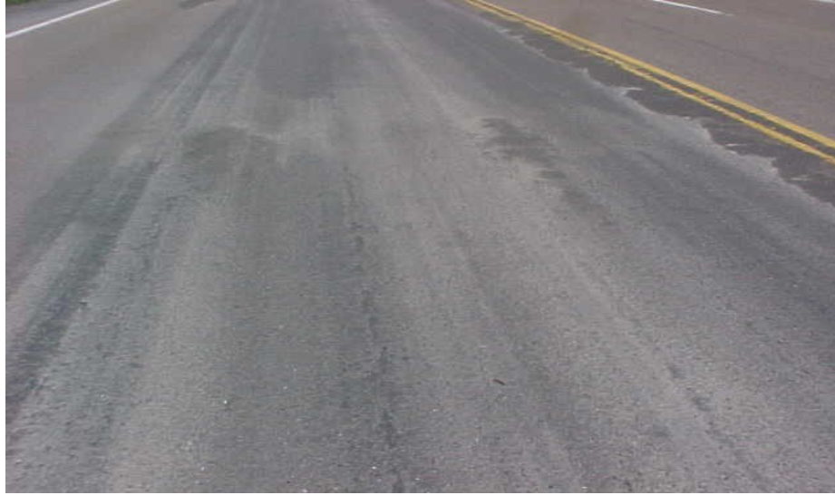
Scrub Seal approximately one year after placement salt is present from winter treatment
