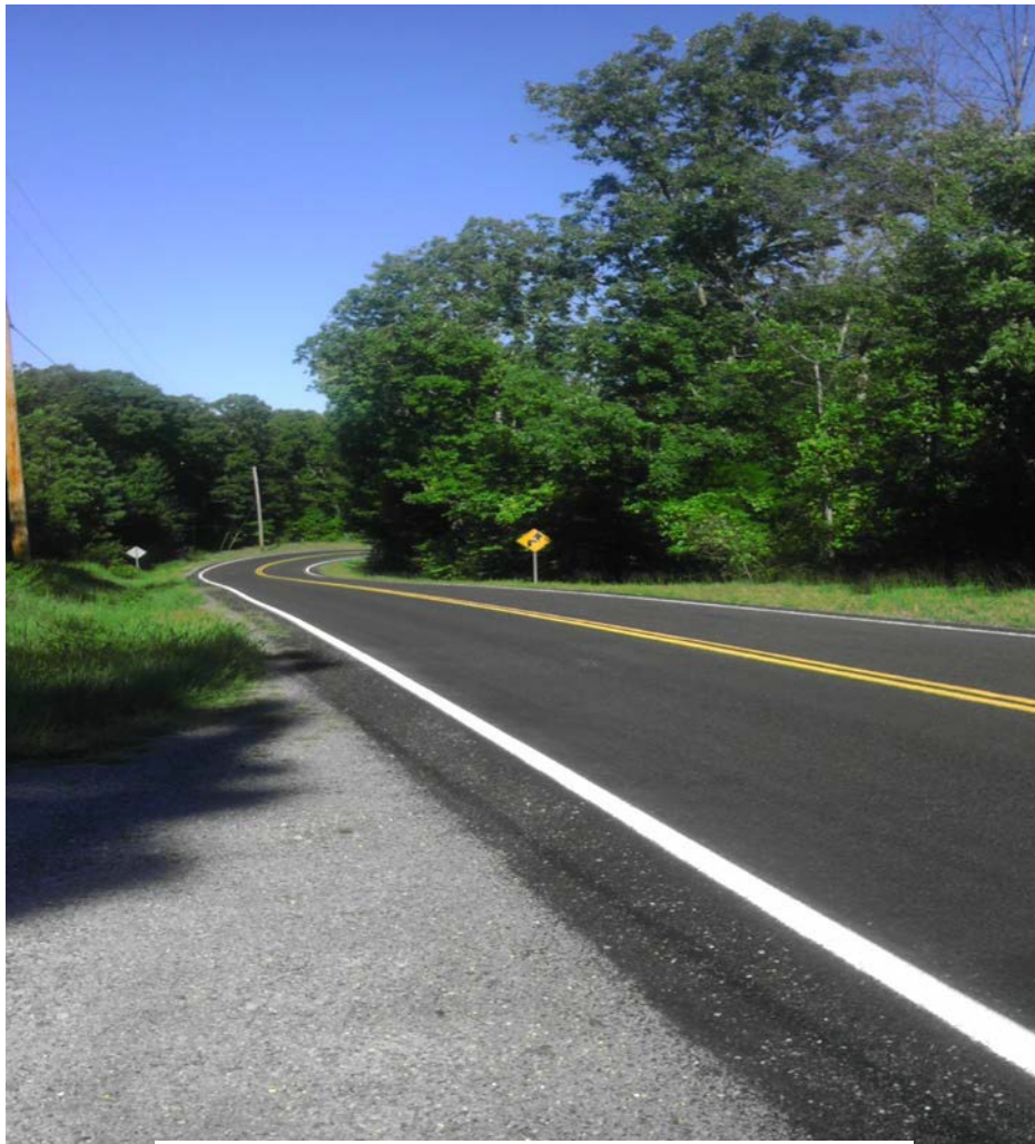
Fog Seal Applied after Chip Seal is complete to help curing and lock aggregate in place
