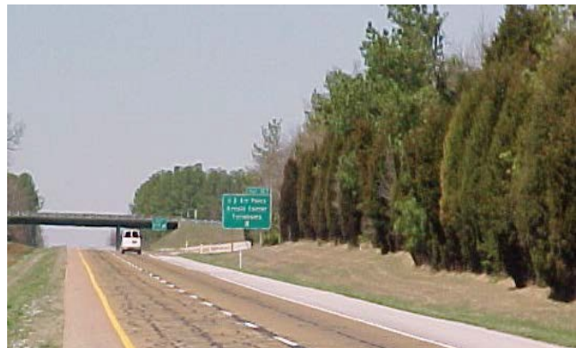
Excessive crack sealing of secondary cracks creating safety concerns
