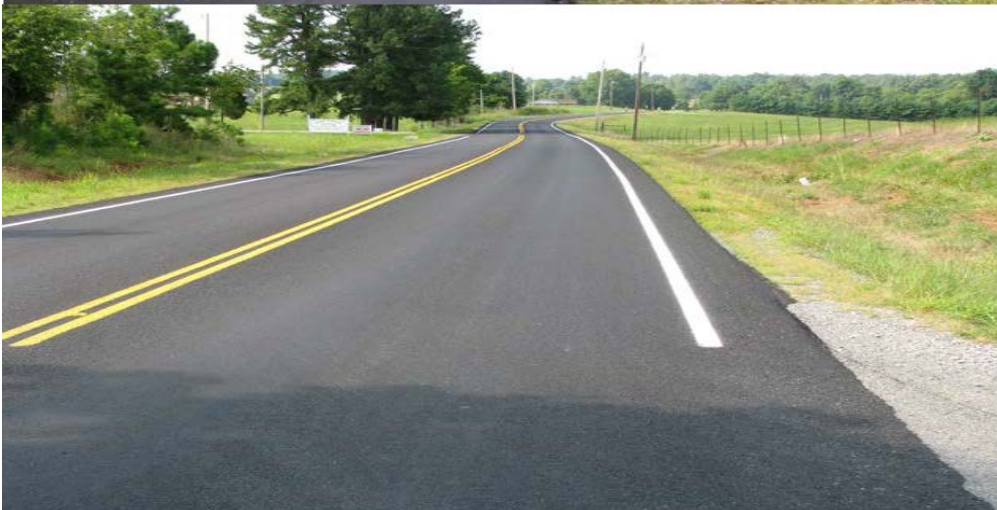
Completed Chip Seal with 24 lbs/SY Microsurfacing
