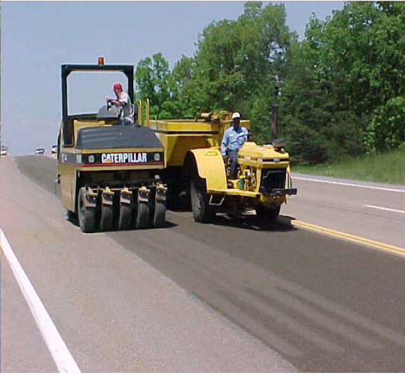
Rolling of aggregate cover material – 2 passes
