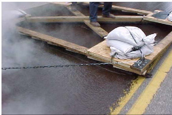
Ribbon of material in front of broom for filling cracks
