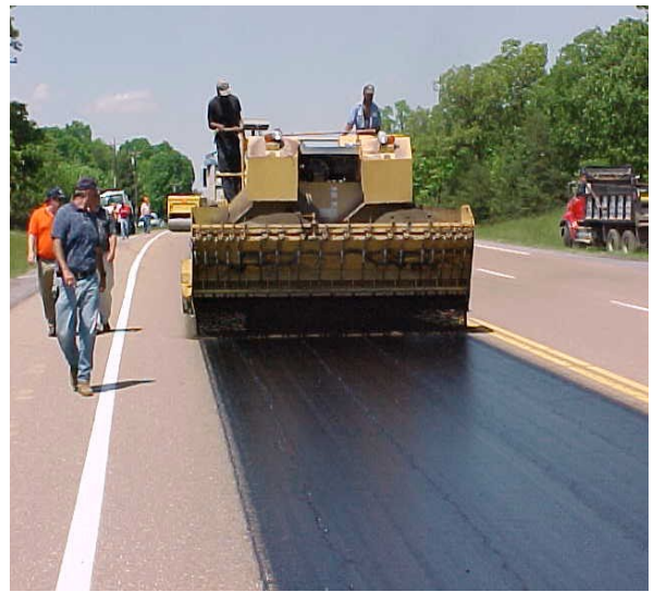
Aggregate applied to asphalt sealer
