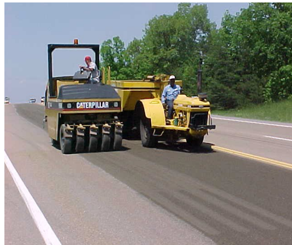
Rolling of aggregate cover material – 2 passes
