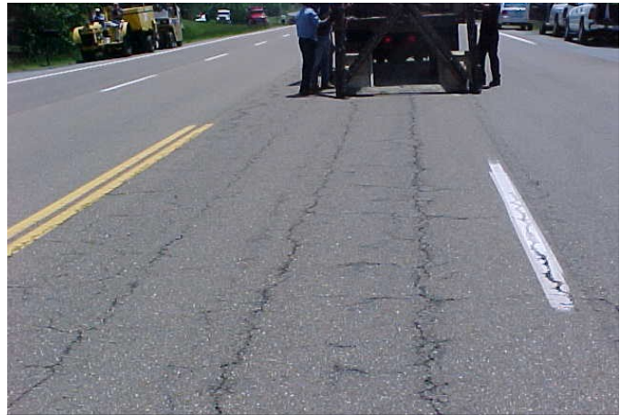
Extensive cracking from oxidized pavement, no structural damage
