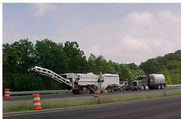
Milling machine and water truck
