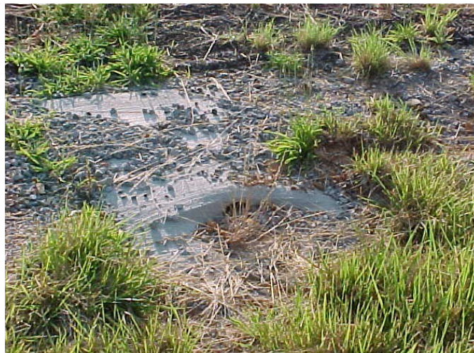
End wall restricted by siltation and vegetation
