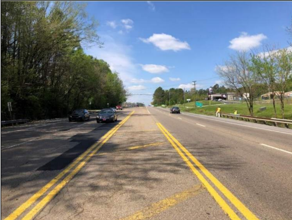
From bridge looking west along roadway
