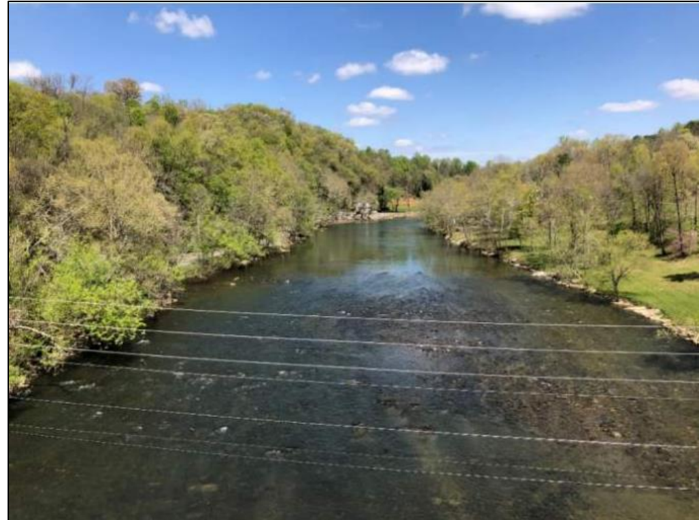
From bridge looking upstream
