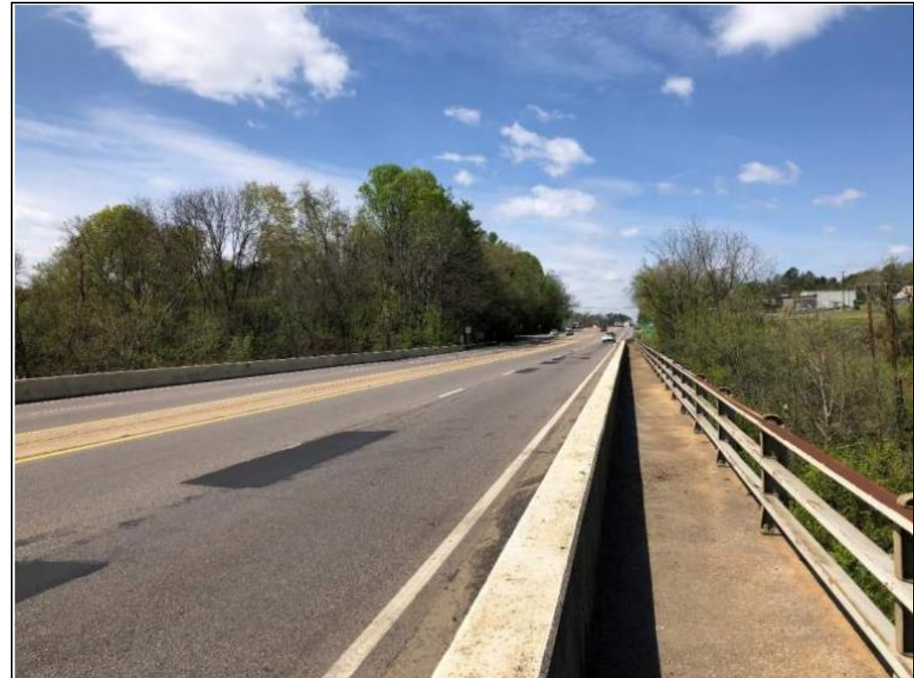
Concrete and steel rail system on bridge
