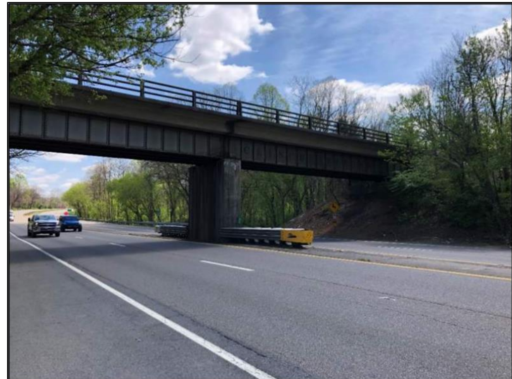
From bridge looking east along roadway
