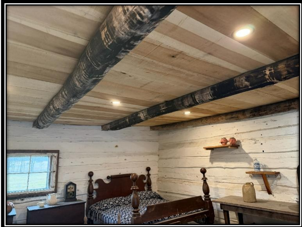
The non-original bead board ceiling in Alfred's Cabin was replaced with a historically appropriate Tulip Poplar wood plank ceiling, December 2025.
