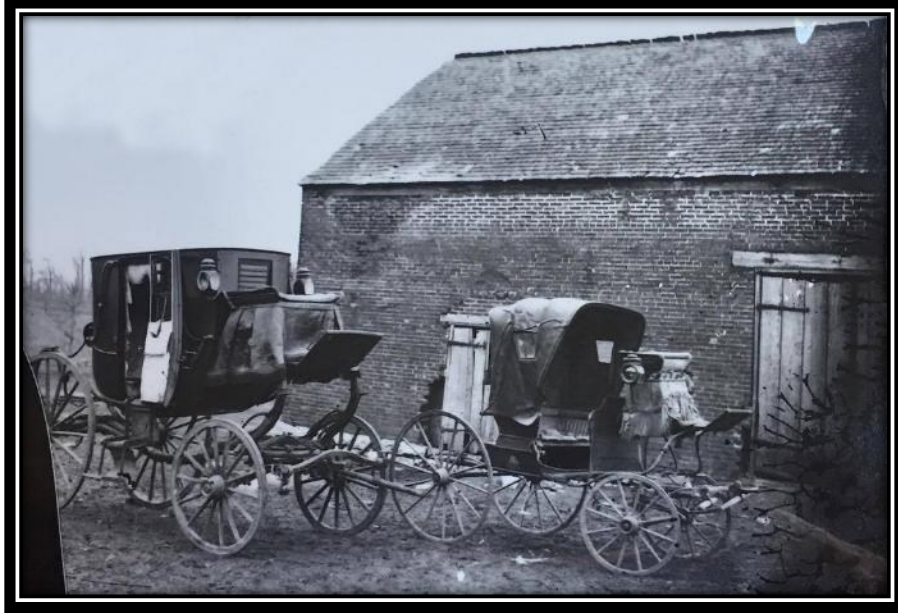
C. 1867 photograph of the Carriage House and Stable, destroyed by fire in the early 1870s.
