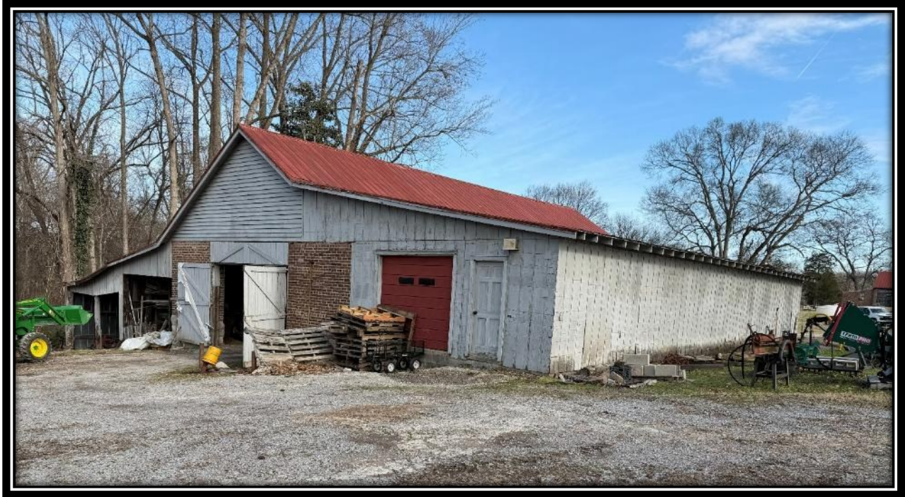
West and south elevations of the Storage Barn, showing storage room on south side and open bay storage on north side, December 2025.
