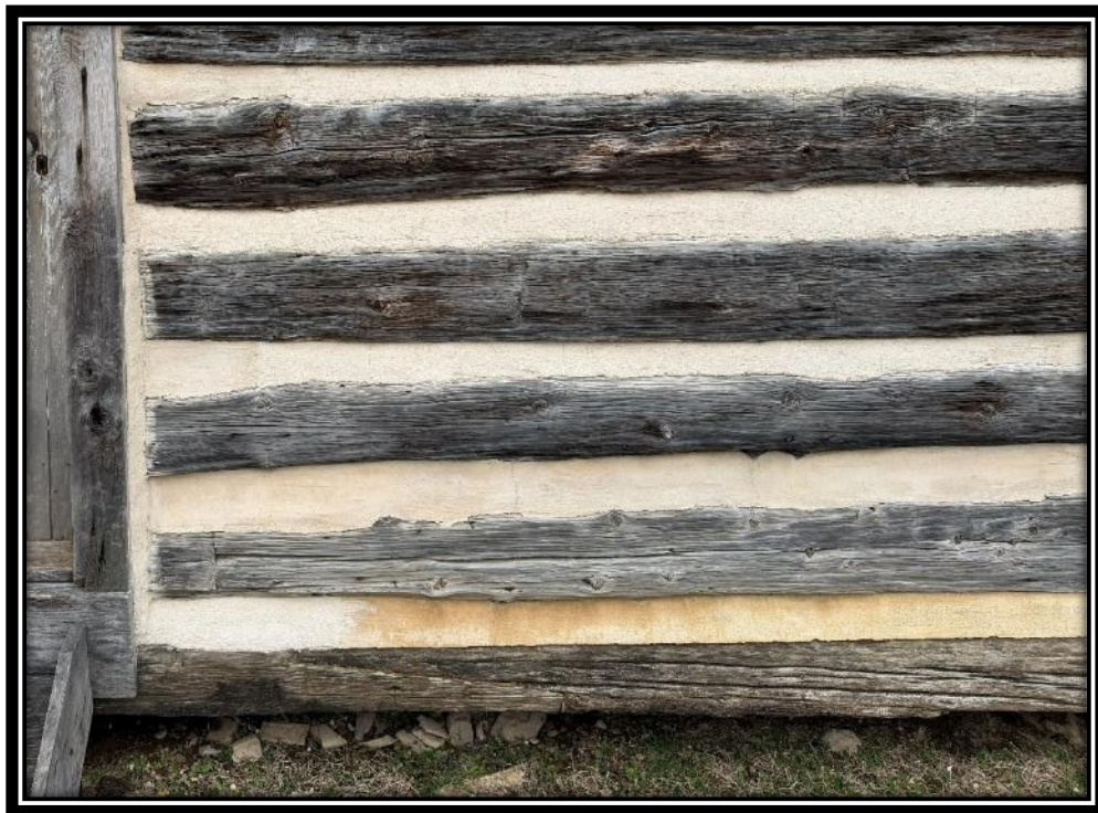
Daubing on Alfred's Cabin after repairs, December 2025.
