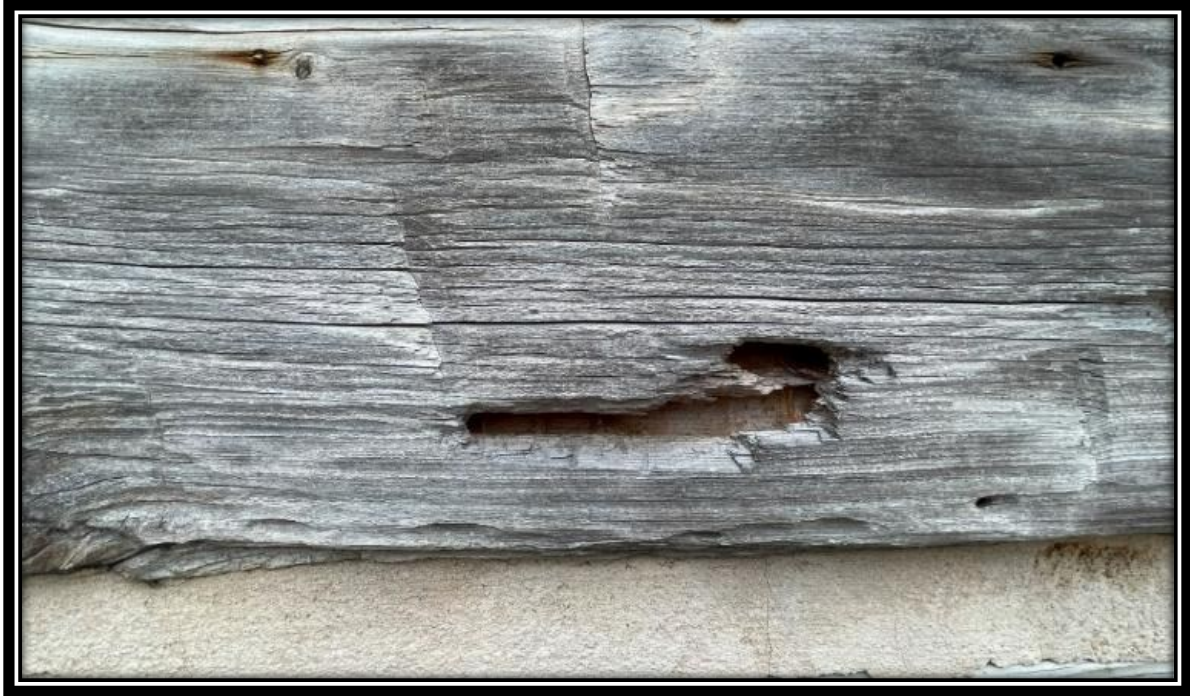
Before, typical log damage at Alfred's Cabin that requires patching to keep water from pooling inside the log cavity, December 2024.
