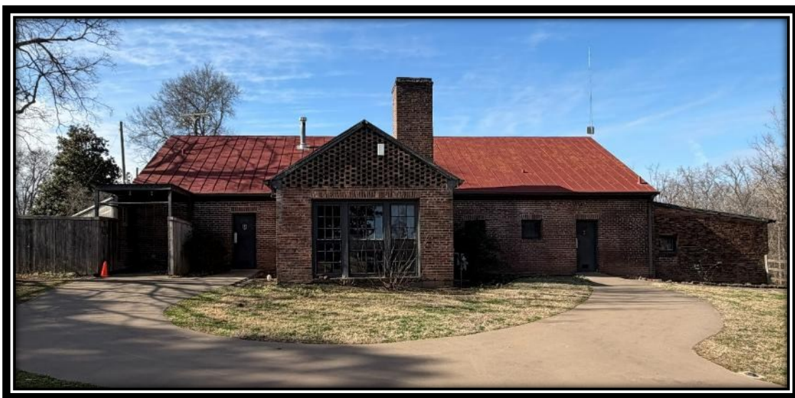
The Maintenance Building East Elevation, December 2025.
