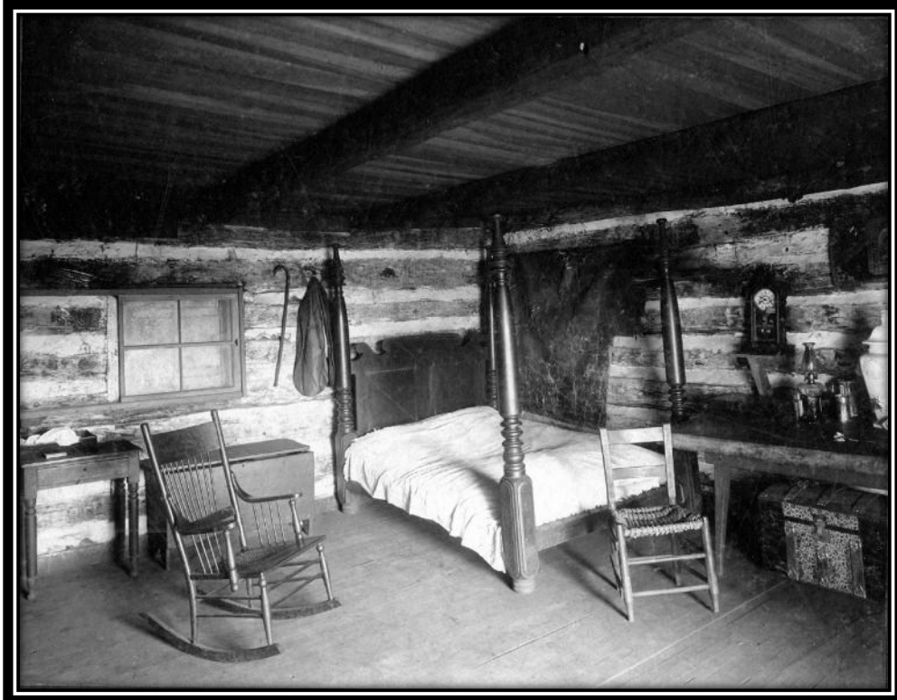
Tulip poplar plank ceiling of in the south pen of Alfred's Cabin as it looked c.1901.
