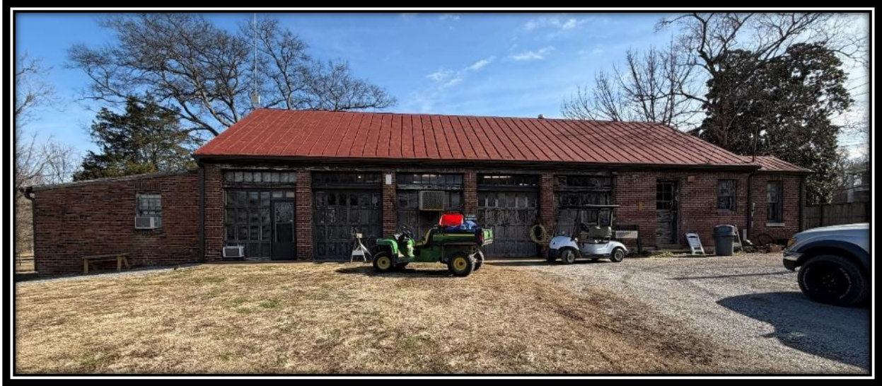
The Maintenance Building West Elevation, December 2025.
