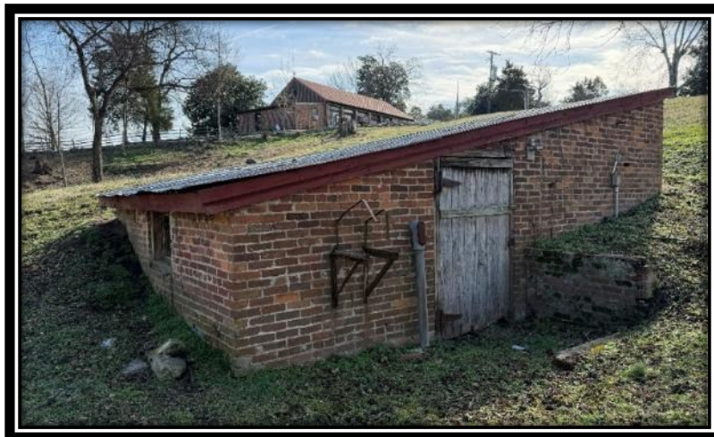
The Pumphouse's north and west elevations, December 2025.
