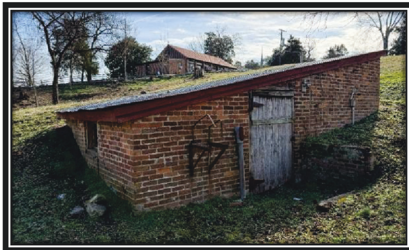
The Pumphouse's north and west elevations, December 2025.
