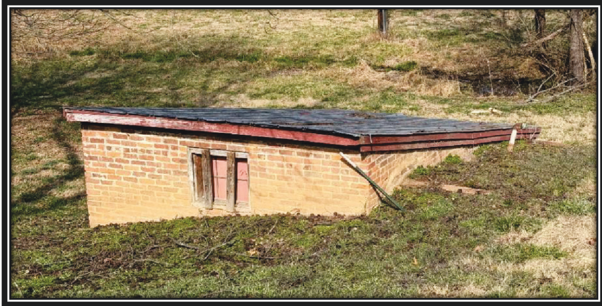
Pumphouse south and east elevations with site of former fire pond in background, December 2025.
