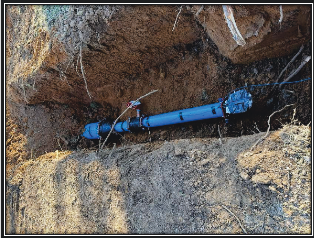
Reducing valve and backflow connection on the new water line at its end point at the Site Operations Facility, December 2025.
