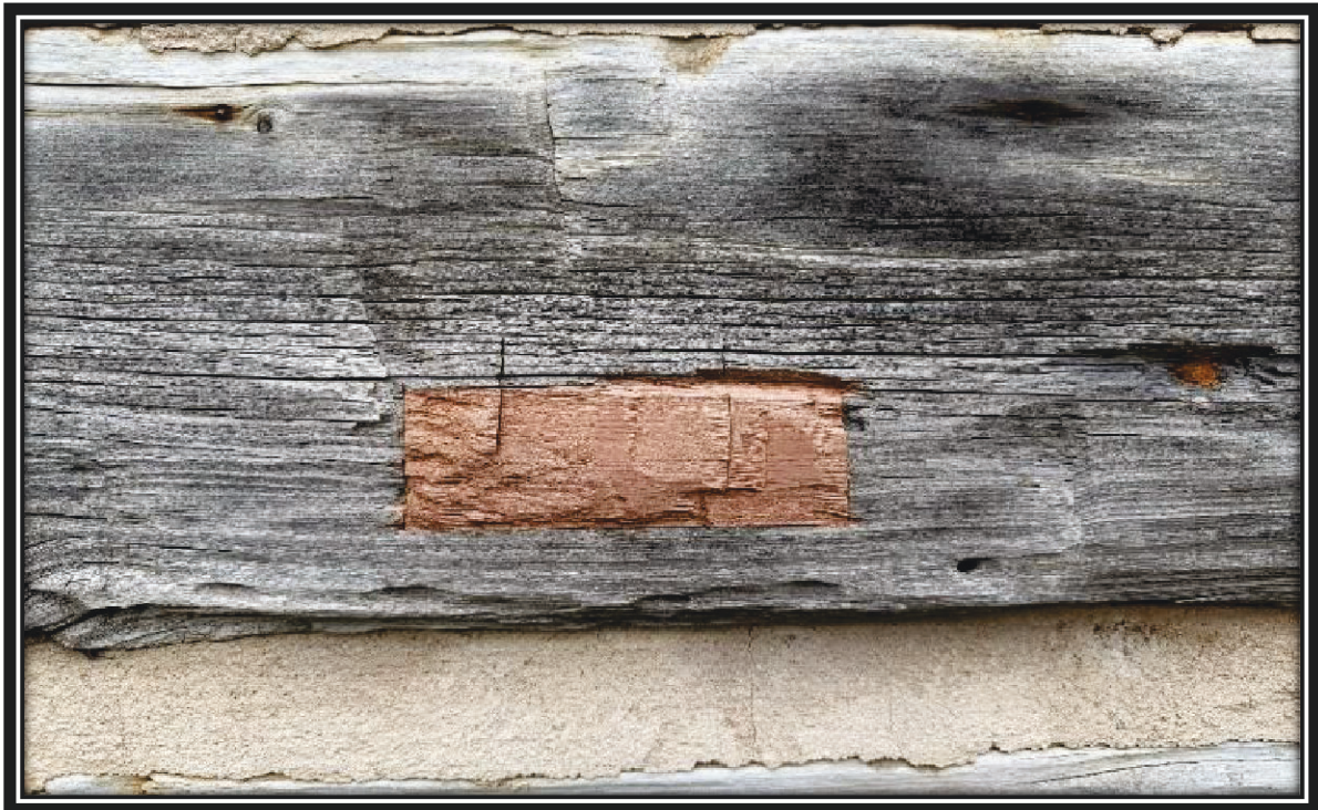
After, log deterioration patched to prevent continued water damage, December 2025.
