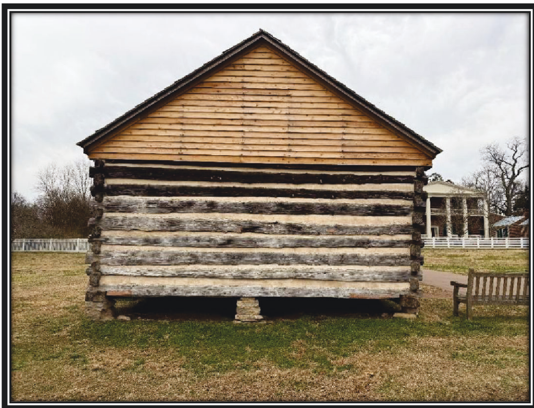
New gable siding several months after installation, December 2025.
