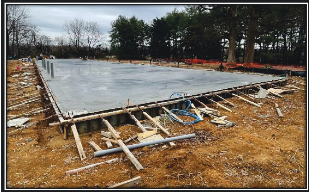
Northwest corner of the Site Operations Building's concrete slab, December 2025.
