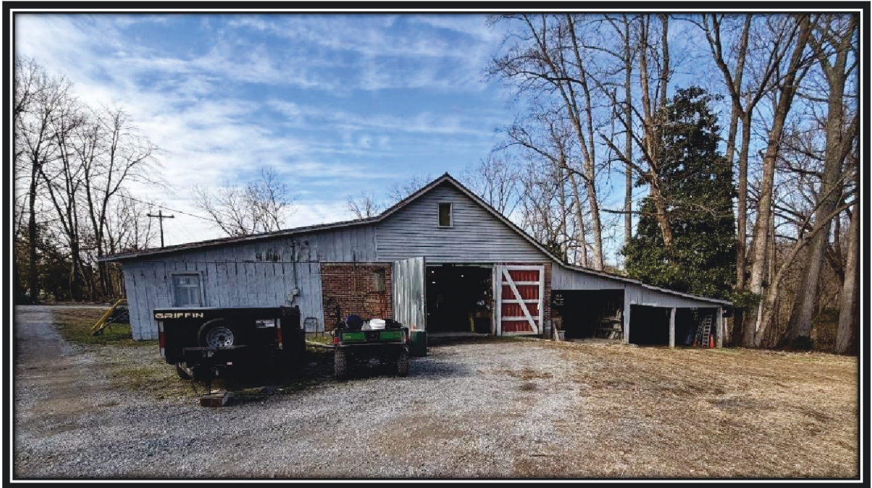
East elevation of the Storage Barn, showing storage room on south side and open bay storage on north side that will be demolished, December 2025.
