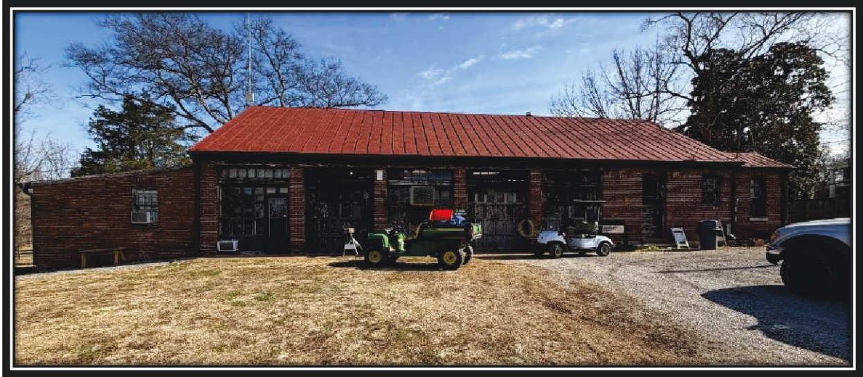
The Maintenance Building West Elevation, December 2025.
