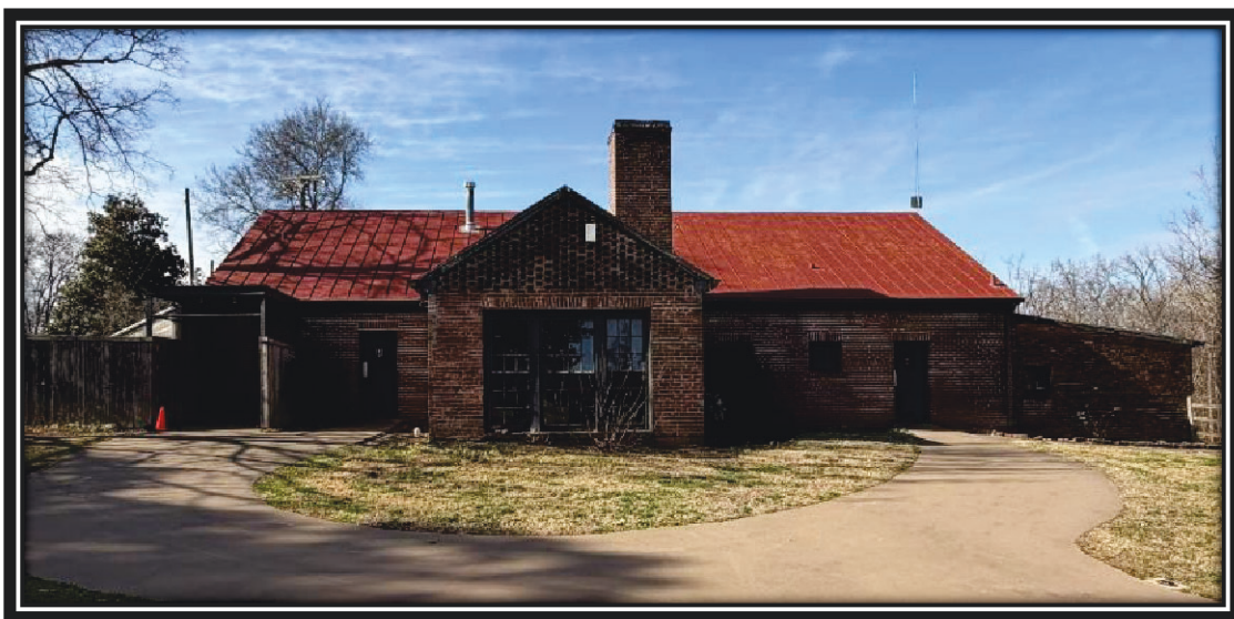
The Maintenance Building East Elevation, December 2025.
