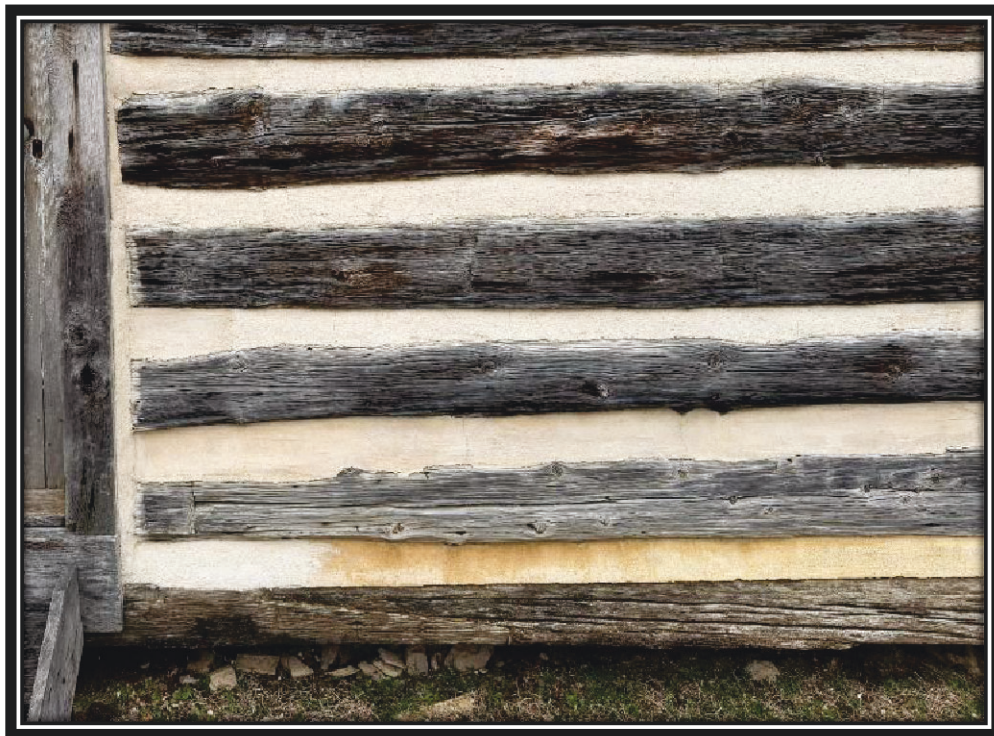
Daubing on Alfred's Cabin after repairs, December 2025.
