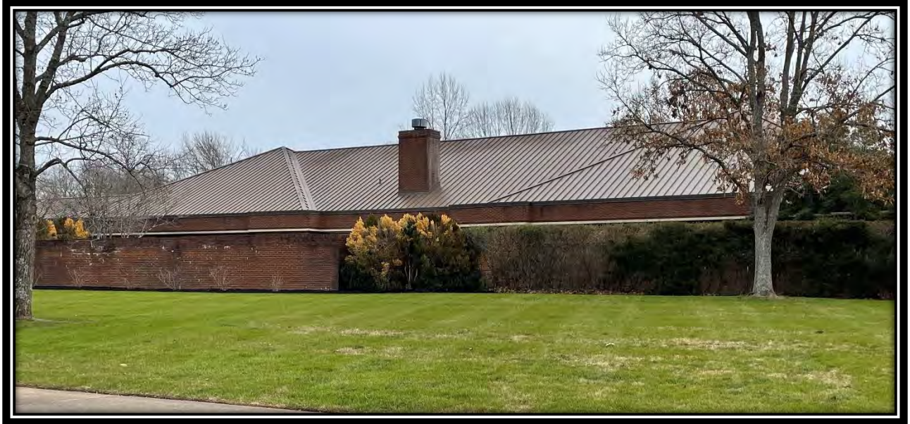
The Andrew Jackson Visitor Center Roof after seal coating and capstone covered with metal, November 2023.
