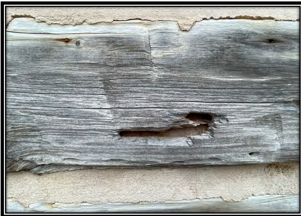
Typical log damage at Alfred's Cabin that requires patching to keep water from pooling inside the log cavity, December 2024.
