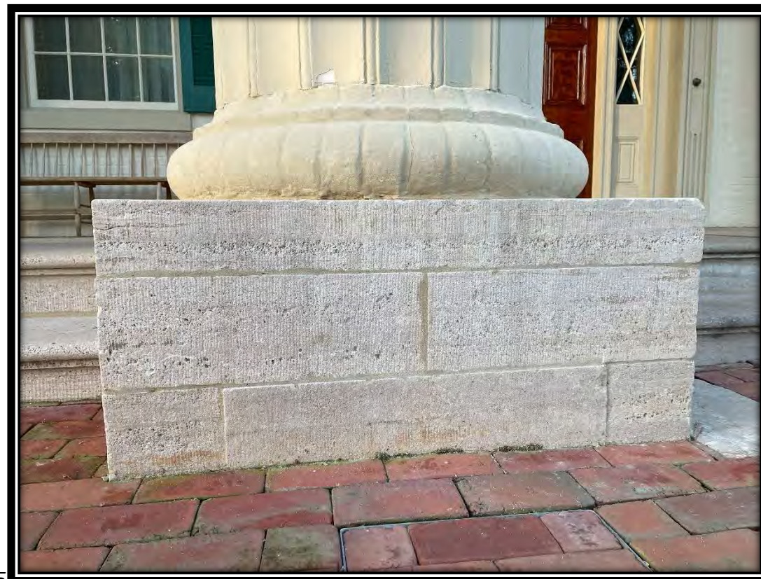
Column bases repointed with masonry mortar, December 2024.
