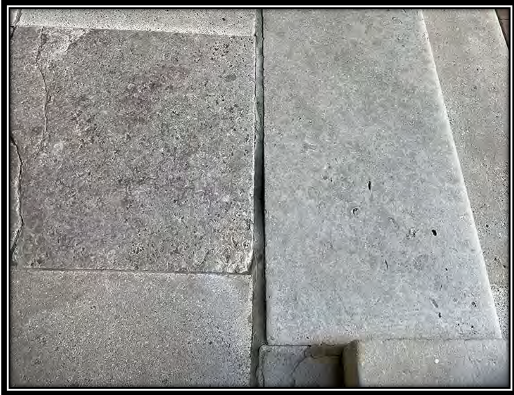
Failed sealant, stone movement, and subsidence, December 2020.
