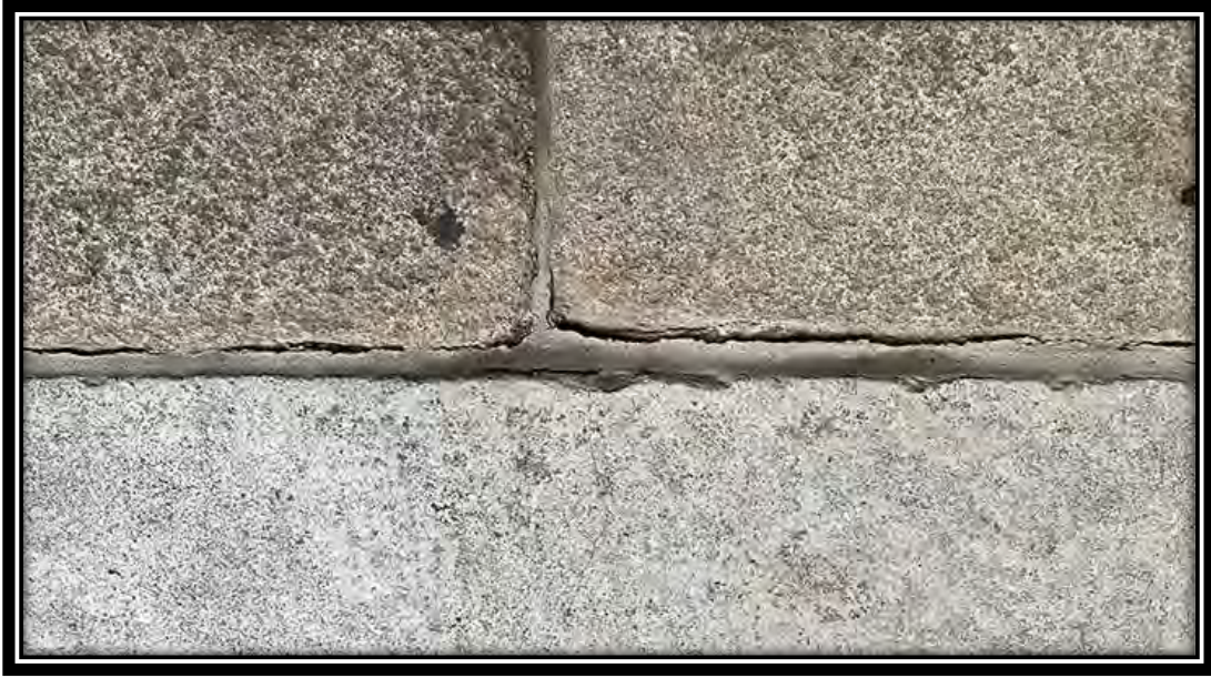
Typical sealant failure in porch floor stone joints, December 2020.
