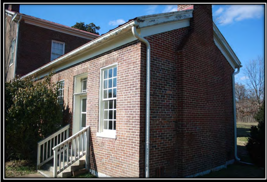
Deteriorated wood trim and gutters, Tulip Grove's kitchen wing, December 2022.
