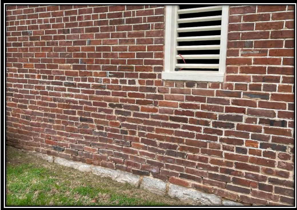
Deteriorated mortar joints on the east elevation of the Hermitage Smokehouse, December 2023.
