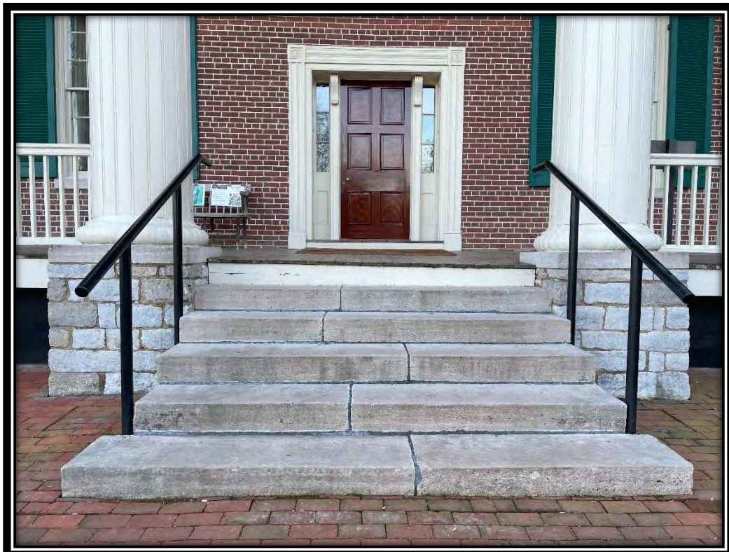
The Hermitage north steps realigned, stabilized, and repointed with lead, December 2024.
