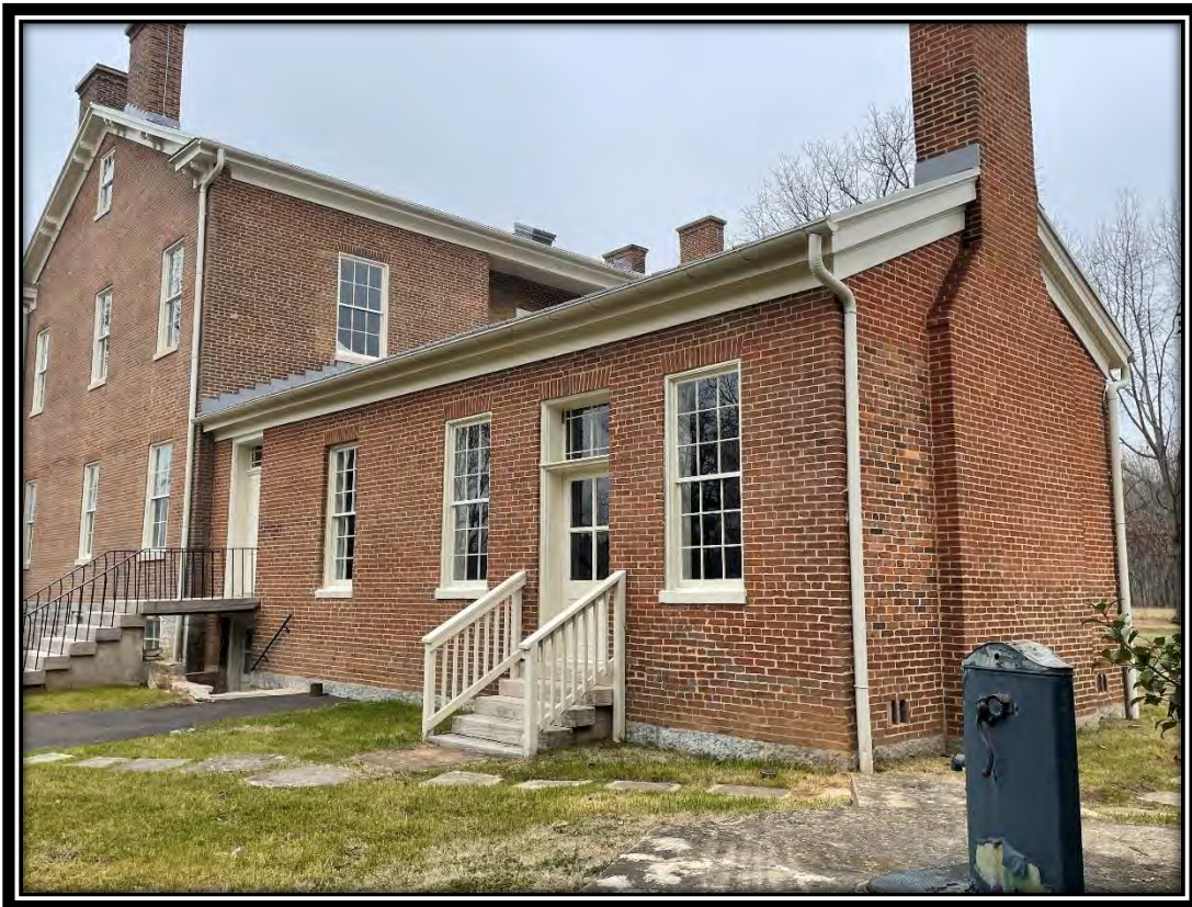
Wood trim repaired and gutters replaced on the kitchen wing, December 2024.
