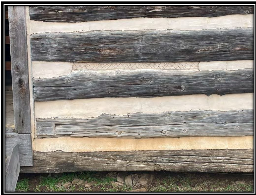
Typical daubing deterioration at Alfred's Cabin, December 2024.
