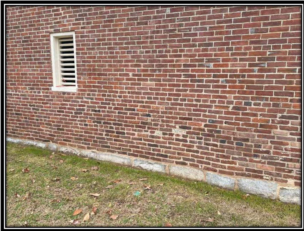
Repointed mortar joints, December 2024.
