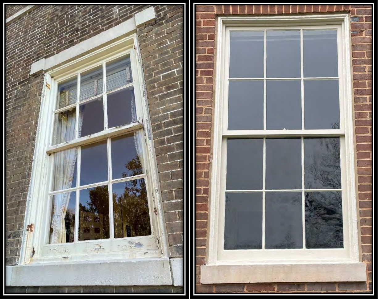
Left, typical window condition prior to work, December 2022. Right, windows after stripping, priming, reglazing, and finish painting, December 2024. All windows are now operable again.
