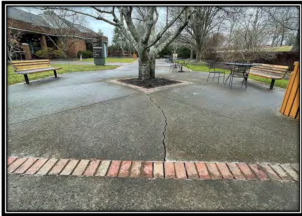
Fractured and heaved concrete slab in the Andrew Jackson Visitor Center courtyard caused by tree roots, December 2021.
