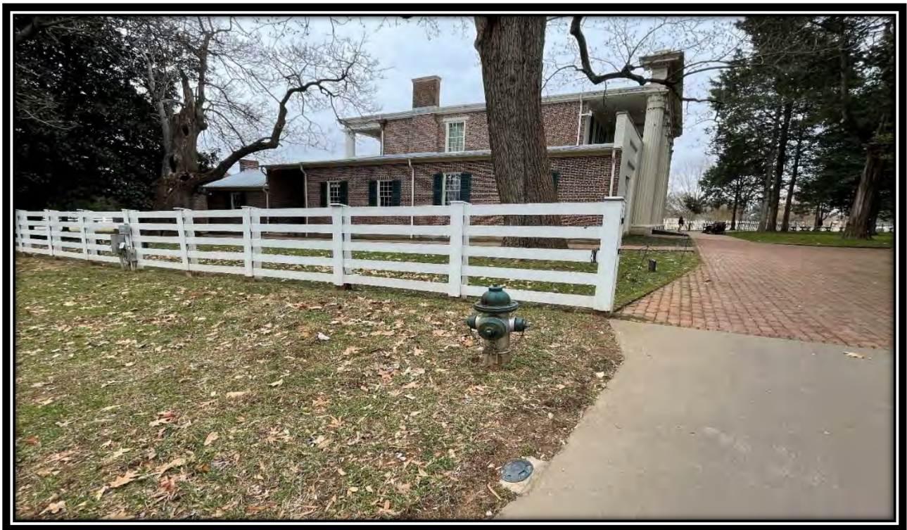
Water volume and residual pressure at this hydrant that protects the National Historic Landmark Hermitage Mansion does not meet modern fire codes, December 2024.
