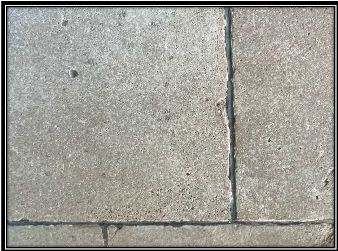
Elastomeric sealants replaced with packed and burnished lead wool between the joints, December 2024.
