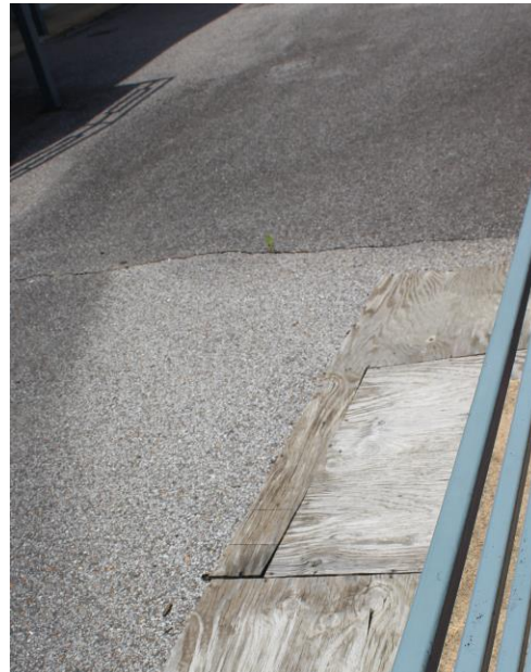
Photograph 8 – Ramp at guard rail
