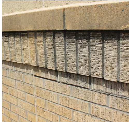
Photograph 4 – Brick/Mortar deterioration
