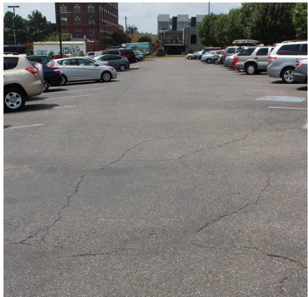
Photograph 6 – Parking lot pavement
