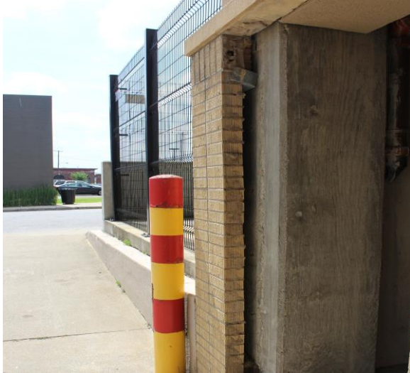
Photograph 3 – Closure at masonry wall
