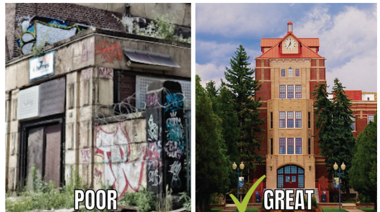
Exceptional maintenance and poor maintenance
