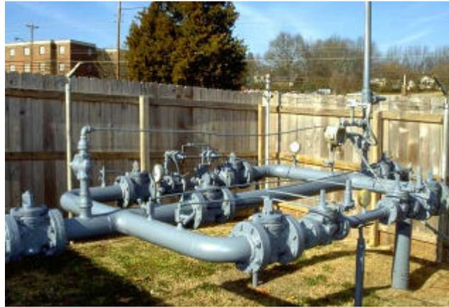
***PRESSURE REGULATING STATION:*** Consists of apparatus installed for the purpose of automatically reducing and regulating the gas pressure in the downstream transmission line, main, holder, pressure vessel or compressor station piping to which it is connected. Included in the station are any enclosures and ventilating equipment, and any piping and auxiliary equipment (such as valves, control instruments or control lines).
