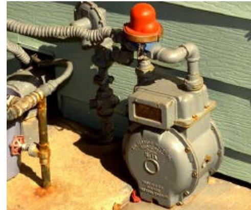
***CUSTOMER REGULATOR:*** A device that maintains a set pressure to the customer.
