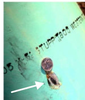
**HOT TAP:** The process of making branch piping connections to operating pipelines, mains, or other facilities while in operation. The connection of the branch piping to the operating line and the tapping of the operating line is done while it is under gas pressure.
