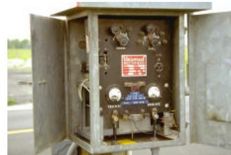
**REGULATOR STATION/DISTRICT:** Equipment installed for the purpose of automatically reducing and regulating the pressure in the downstream pipeline or main to which it is connected. Included are piping and auxiliary devices such as valves, control instruments, control lines, the enclosure, and ventilation equipment.
