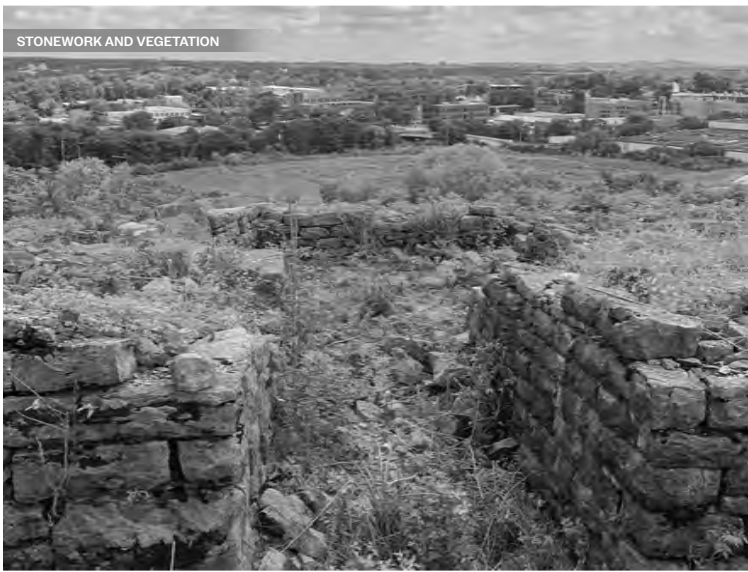
Dry-stacked limestone masonry walls are gravity-type retaining walls, meaning they derive stability from having enough weight to resist sliding and overturning, yet are not so heavy as to cause a bearing capacity failure of the foundation soils. Numerous areas of stonework have collapsed or are at acute risk of collapsing. At the time of this writing, a first phase of stonework repair is underway and is scheduled to be complete by the end of 2022.
