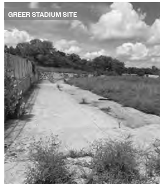
Dry-stacked limestone masonry walls are gravity-type retaining walls, meaning they derive stability from having enough weight to resist sliding and overturning, yet are not so heavy as to cause a bearing capacity failure of the foundation soils. Numerous areas of stonework have collapsed or are at acute risk of collapsing. At the time of this writing, a first phase of stonework repair is underway and is scheduled to be complete by the end of 2022.
