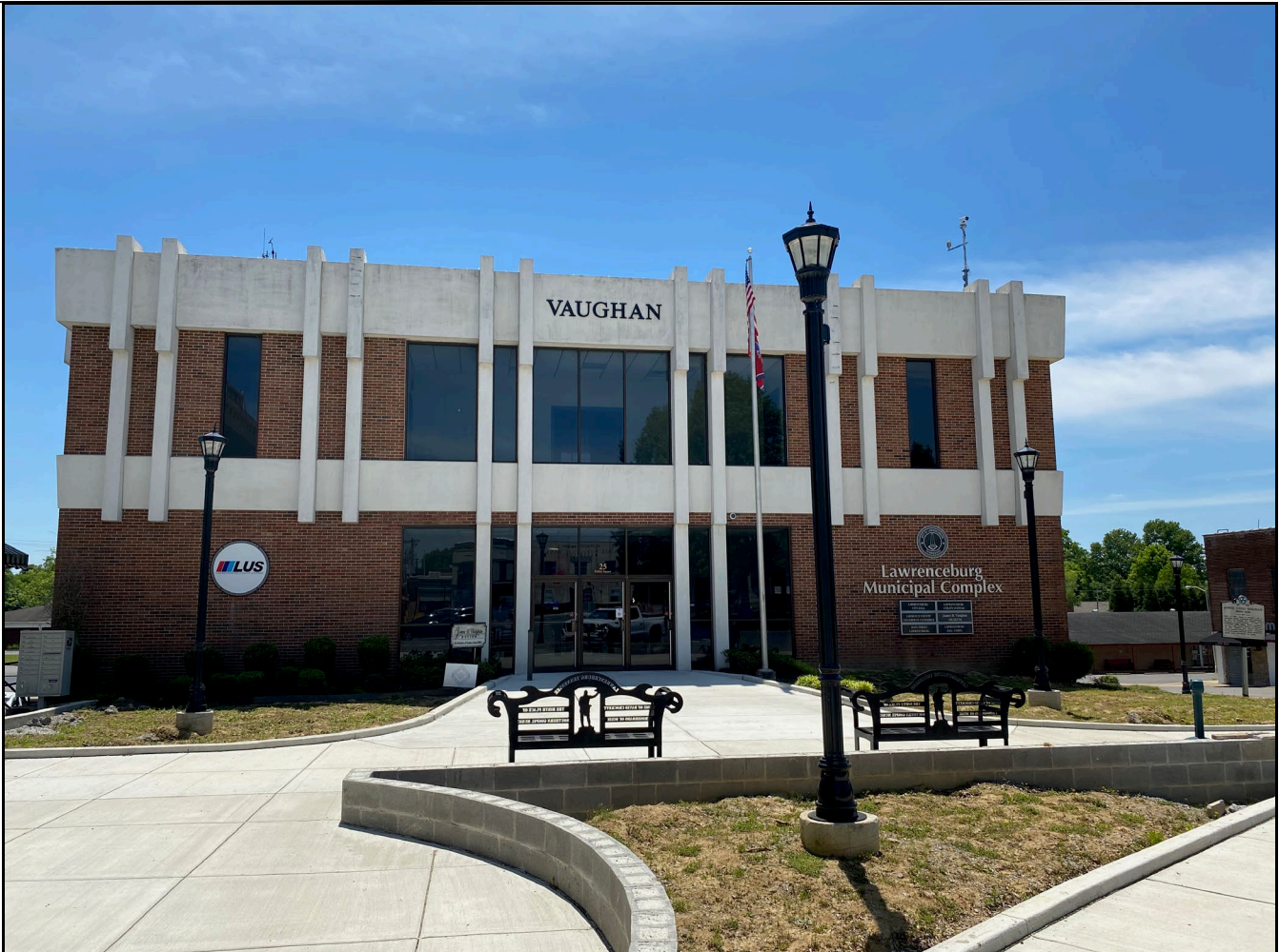
Figure 7: The ca. 1977 Lawrenceburg Municipal Center (formerly Third National Bank). Photo Courtesy of Tennessee Historical Commission.
