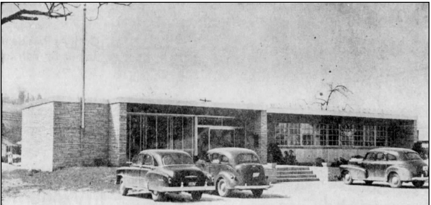
Figure 7: Mountain Electric Cooperative Building, 1925. From the Bristol Herald Courier , April 6, 1952.
