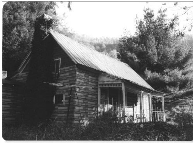
Figure 6: Head House, facade.
