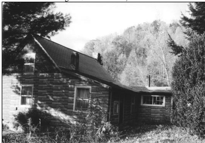
Figure 7: Head house, ell addition.
