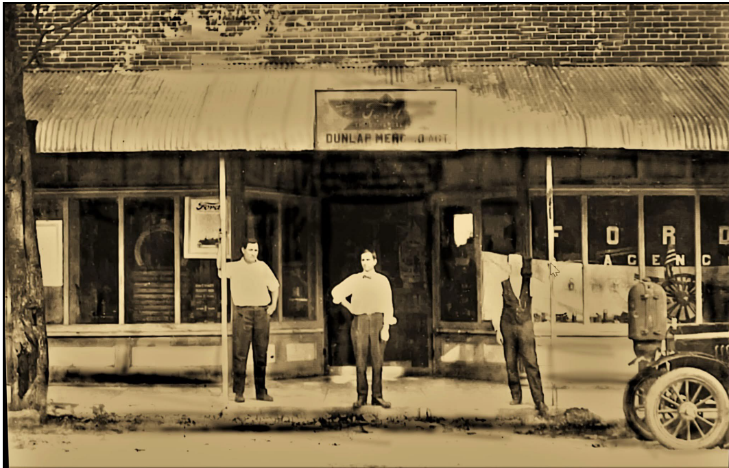
Figure 2: The Dunlap Mercantile Company and Dunlap Automotive Company building was a Ford dealership at one point. Circa 1930s photo provided by the Sequatchie Valley Historical Association – Dunlap Coke Ovens Museum.
