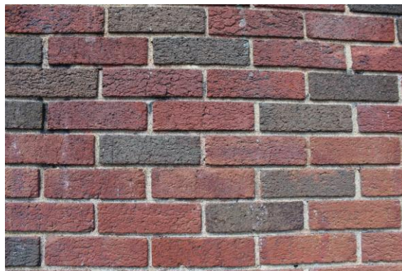
Figure 4: Exterior wall on the west elevation of the Coca-Cola Bottling Plant.
