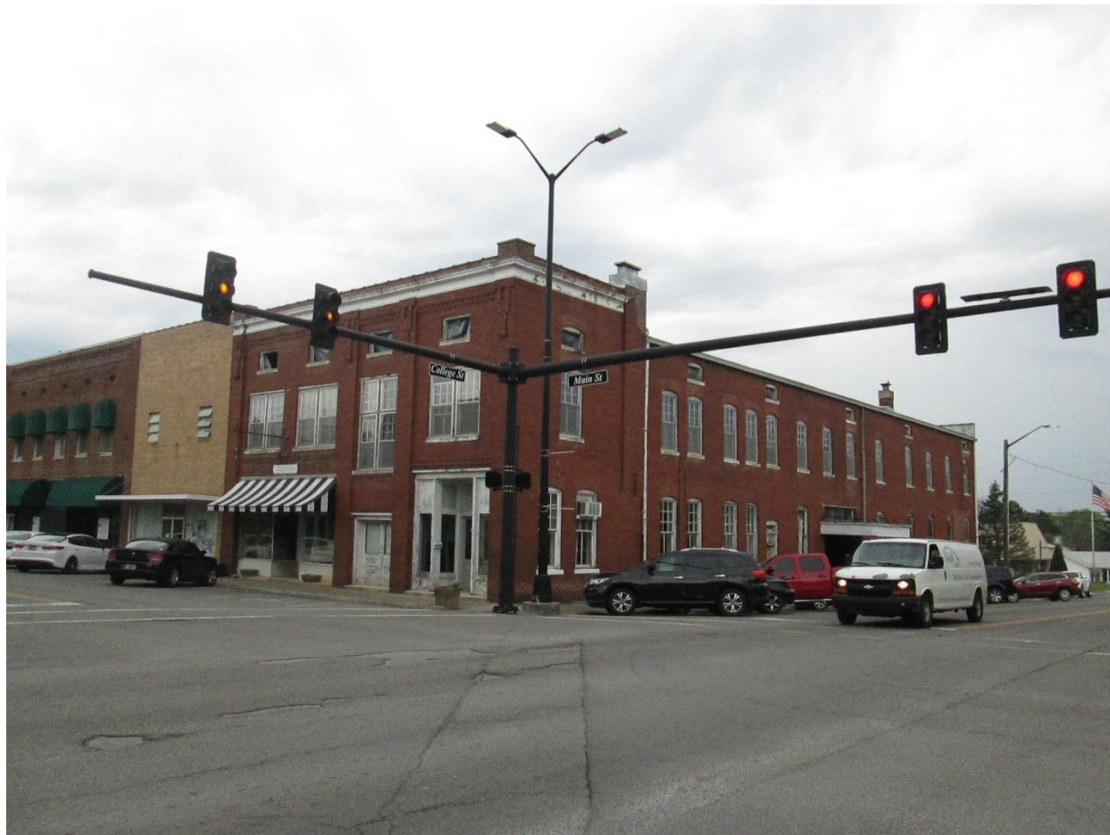
Photograph 4. Kefauver Hotel façade (south elevation) and east elevation, at the intersection of Main Street (left) and College Street (right), facing northwest.
