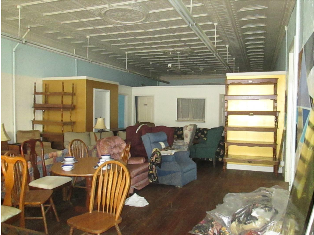
Photograph 17. First floor retail space in Kefauver Hotel building, showing partial walls added at an unknown date, facing northwest.
