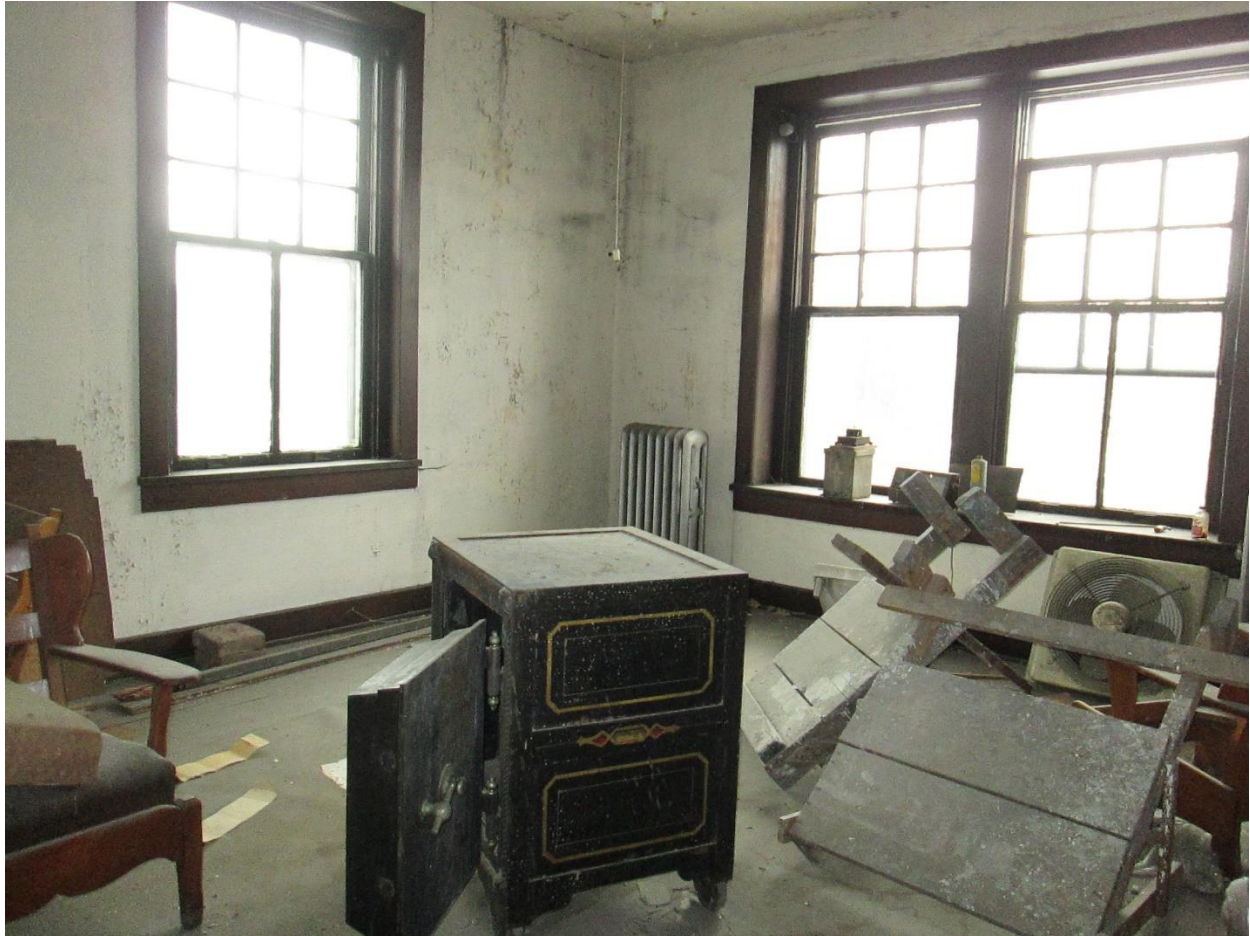
Photograph 25. Example of an office space on the second floor of the Kefauver Hotel, facing southwest.
