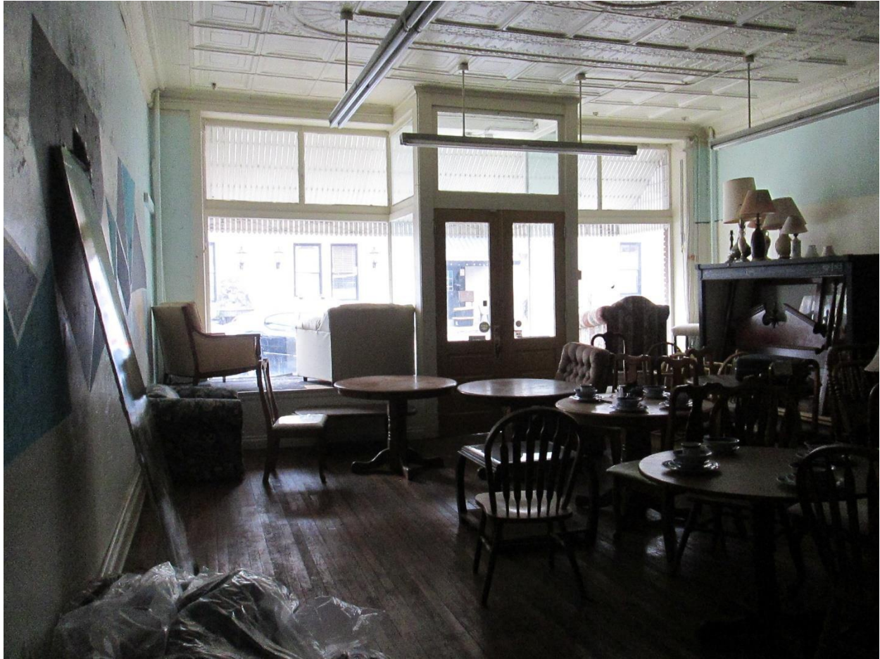
Photograph 16. First floor retail space in Kefauver Hotel building, facing south-southwest.
