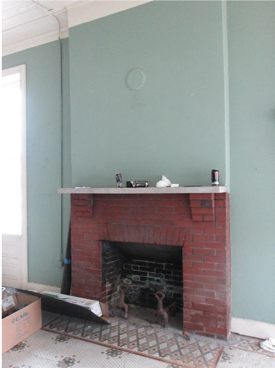
Photograph 12. Fireplace in Kefauver Hotel lobby, facing east-northeast.
