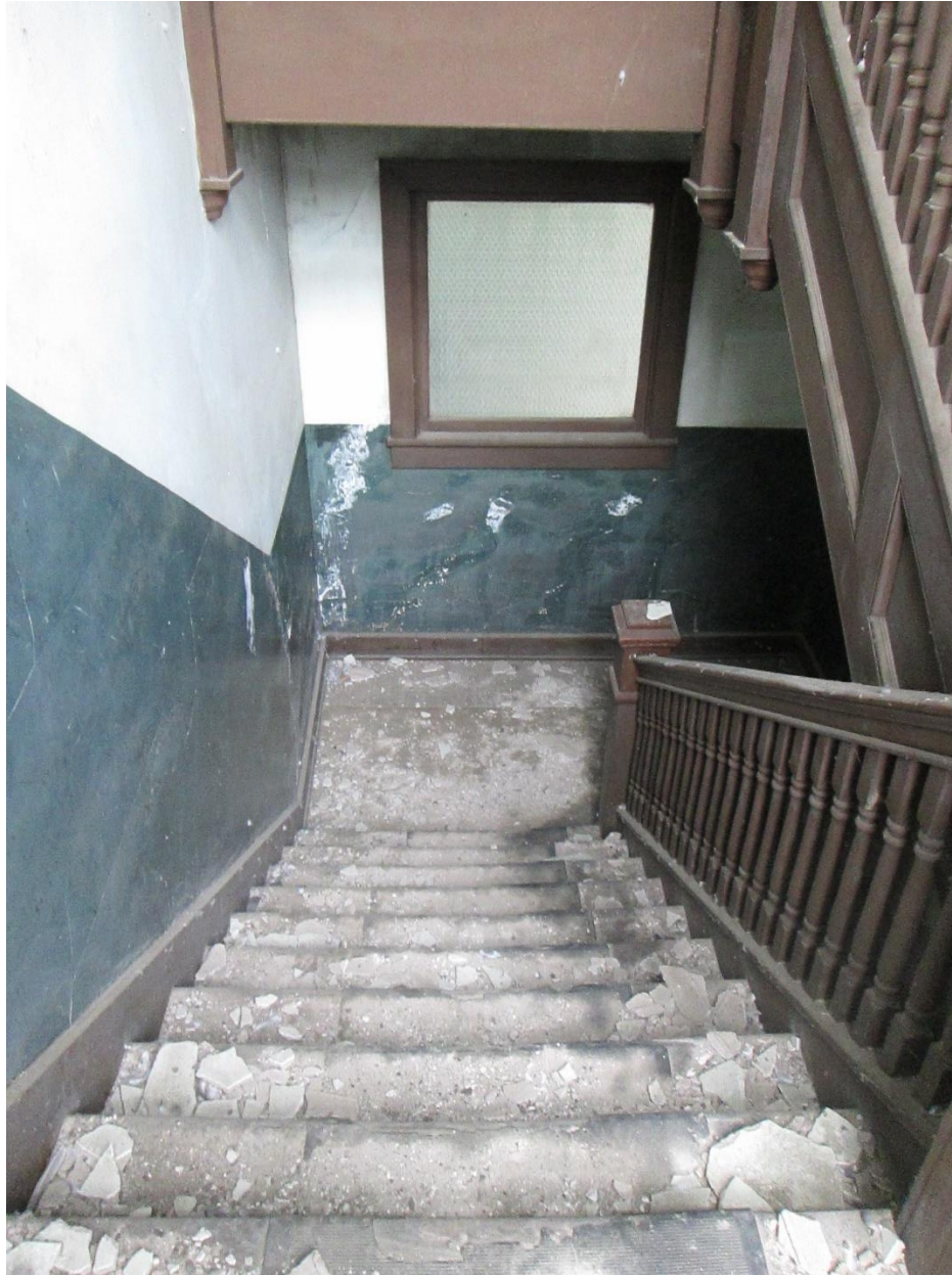
Photograph 27. Front stairway to first floor of Kefauver Hotel, facing north.
