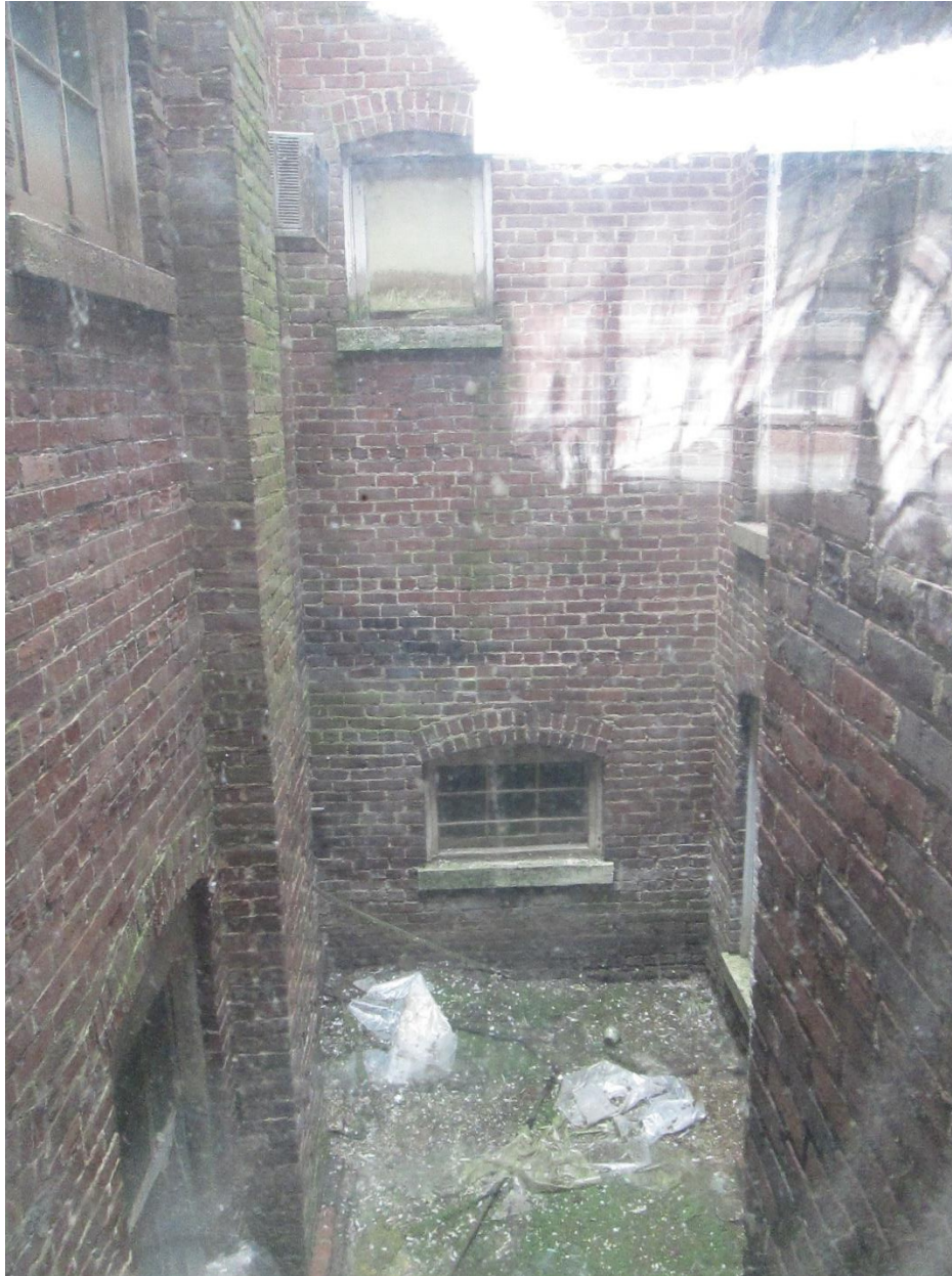
Photograph 15. Interior atrium centrally located within the Kefauver Hotel, facing west.
