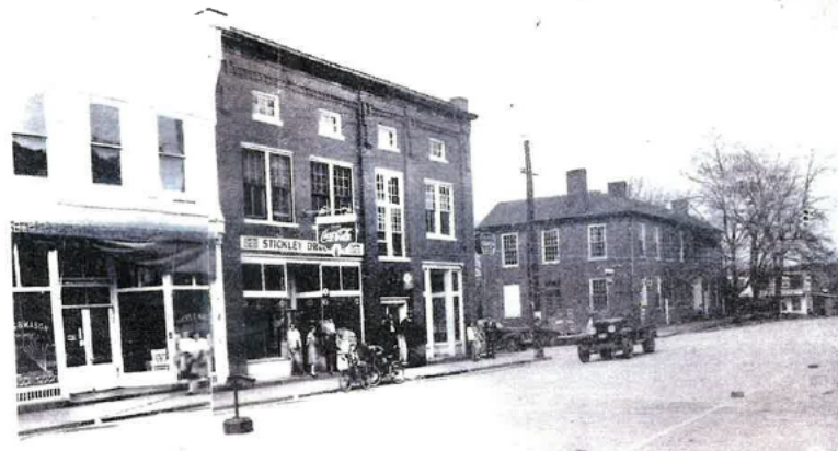
THE KEFAUVER HOTEL in Madisonville was in operation when this picture was made in the 1930's.
