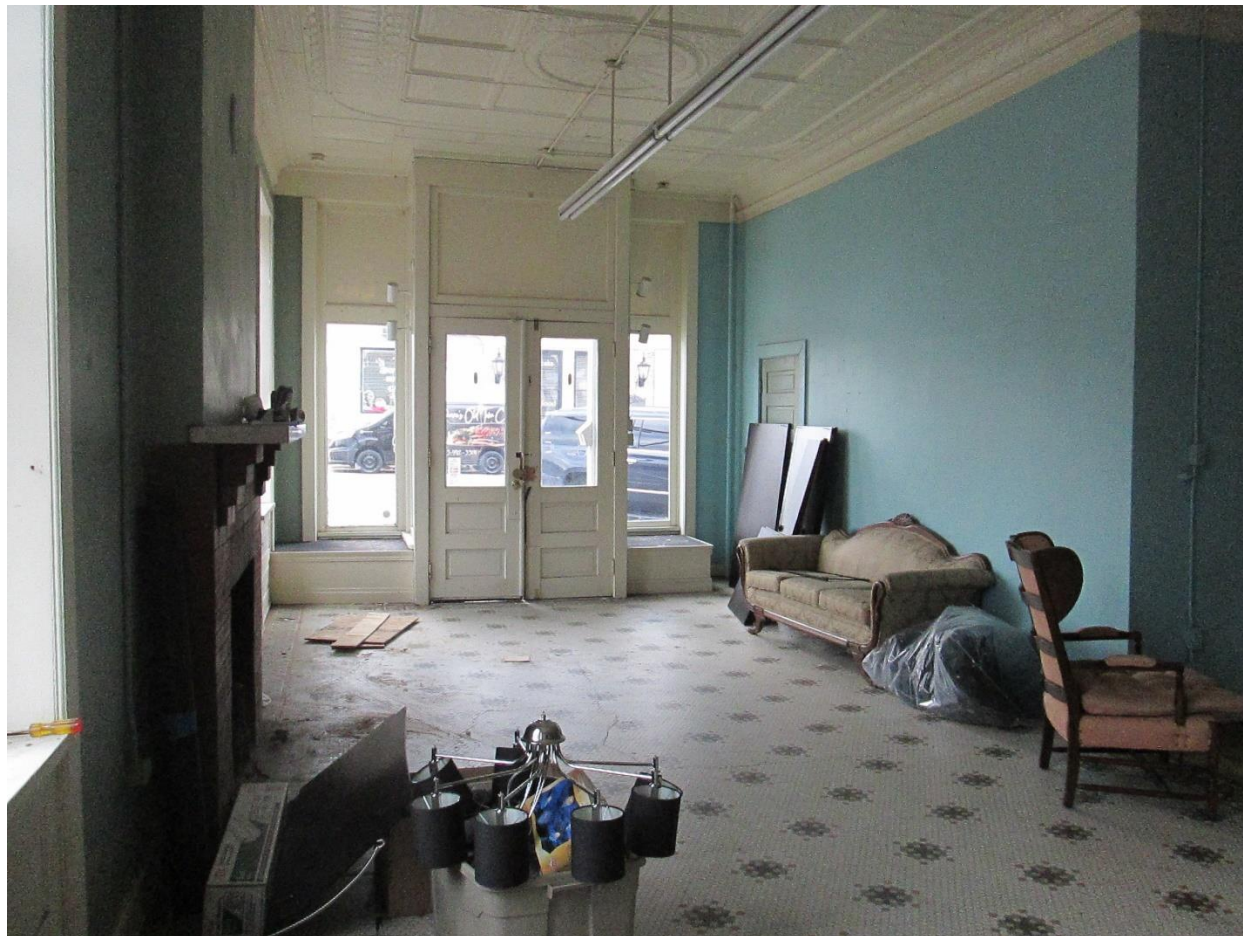
Photograph 9. Original Kefauver Hotel lobby, including original pressed metal ceiling, mosaic tiled floor, and doors, looking south-southwest.
