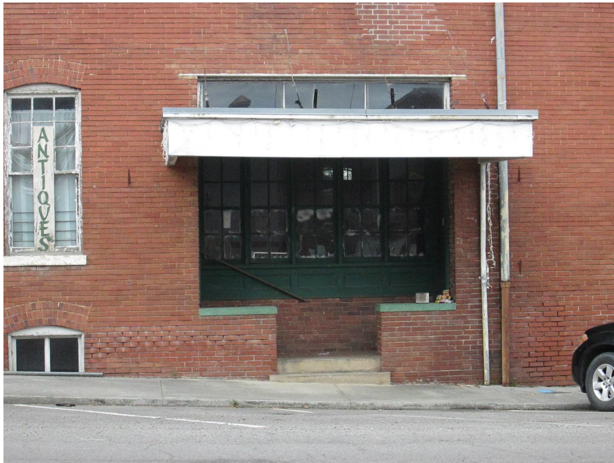
Photograph 5. Detail of entry along east elevation of the Kefauver Hotel, added circa 1940, facing west.
