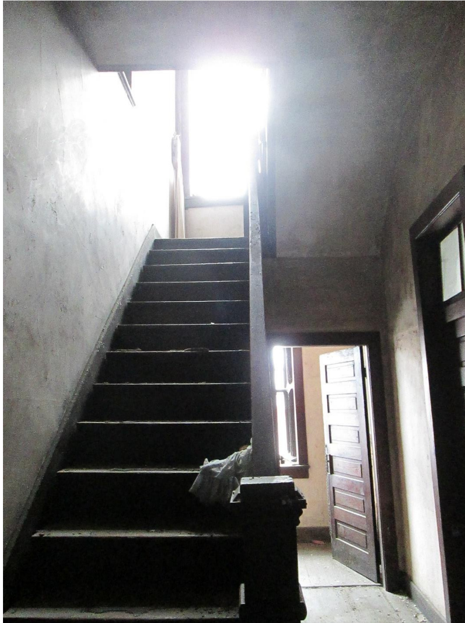
Photograph 20. Back stairway to second floor of Kefauver Hotel, facing north.
