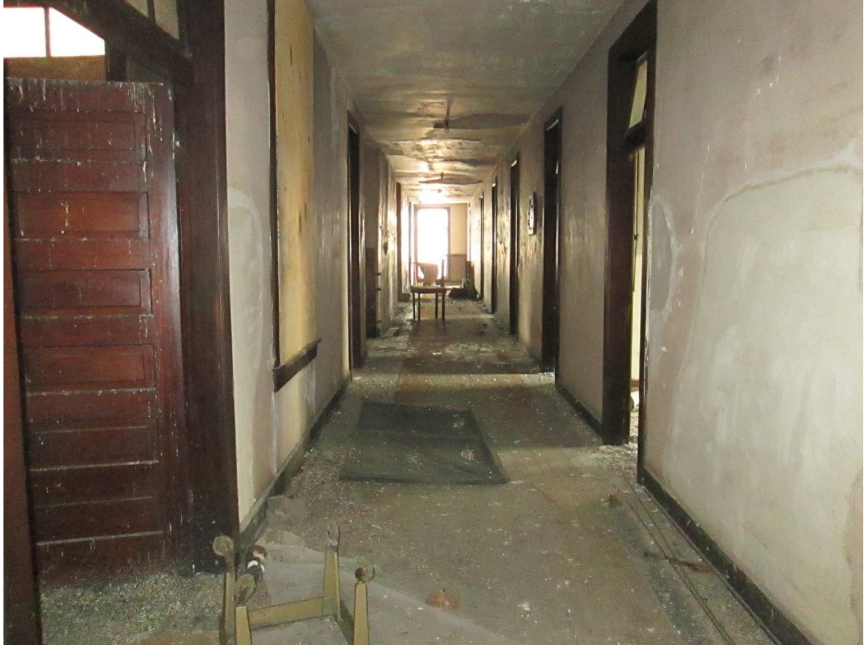
Photograph 21. Second floor hallways in Kefauver Hotel, facing north.
