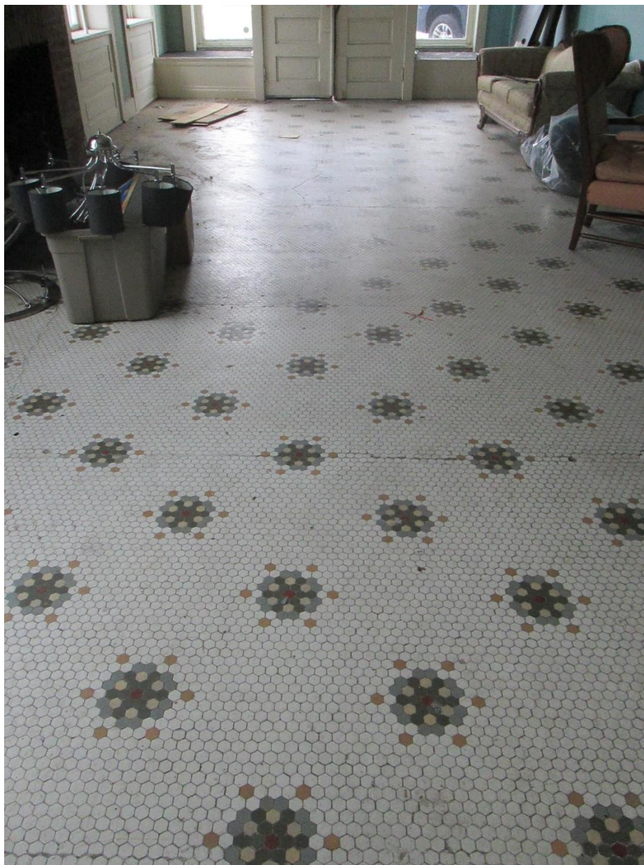
Photograph 11. Detail of original mosaic tile floor in Kefauver Hotel lobby.
