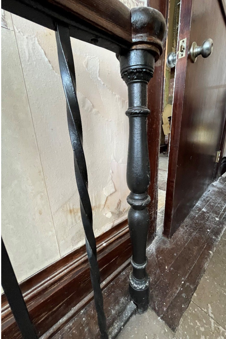
3: Detail of lobby staircase balusters, looking west.
