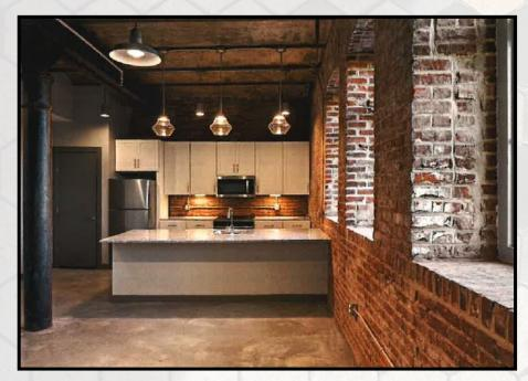
Exposed brickwork (above) or floor joists (right) are acceptable treatments in buildings that were historically unfinished spaces, such as former industrial buildings. In the photo on the right, exposed brickwork and joists are maintained, while gypsum was used for new partition walls. In historically unfinished spaces, systems can remain exposed as well. For more information about systems and interior finishes, see Treatments Resource Guide: Systems, Codes, and Energy Efficiency.
