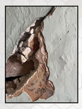
Deteriorated finishes, such as plaster on walls (left) and ceilings (right), must be repaired and the space must be finished to match the historic character. "Cow-patching," or leaving spots of deteriorated plaster, to give a "rustic" look, is not an approved treatment.
