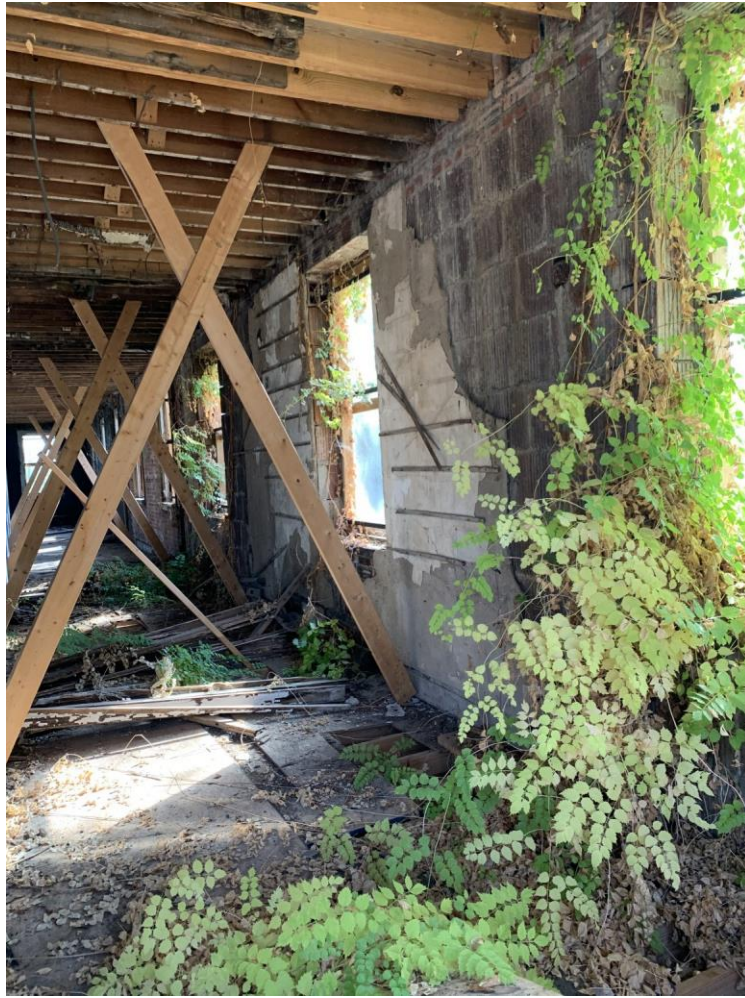
Photo 15, First Floor, west wall from front of building
