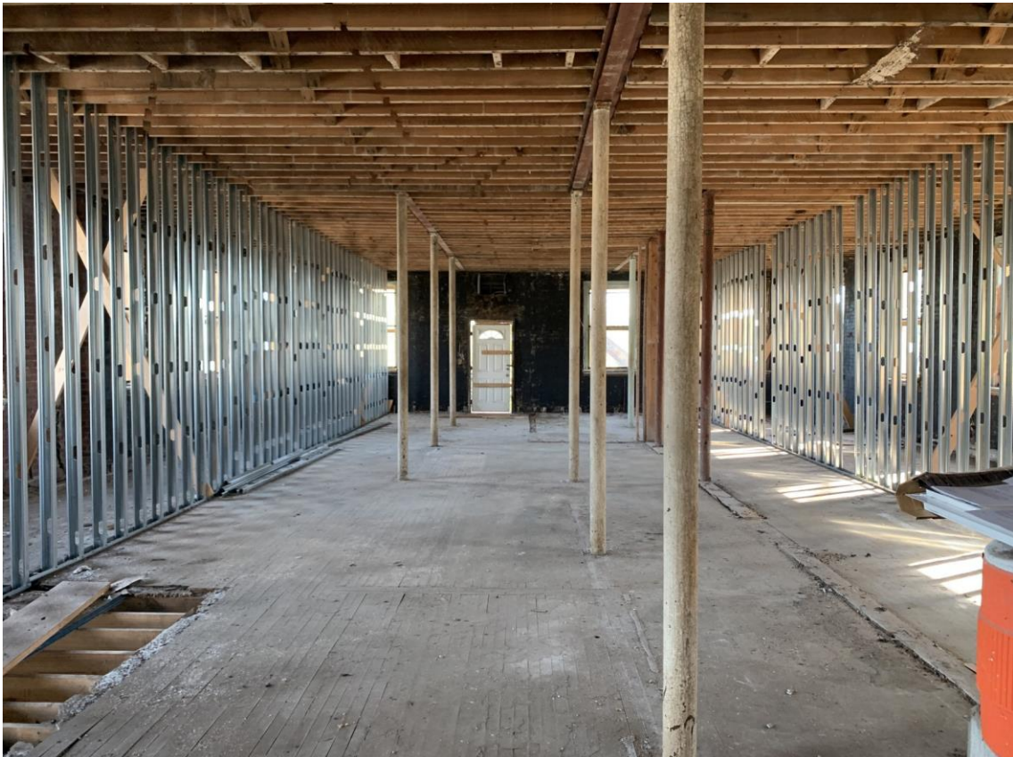
Photo 12, First floor, Looking from left of stairs
