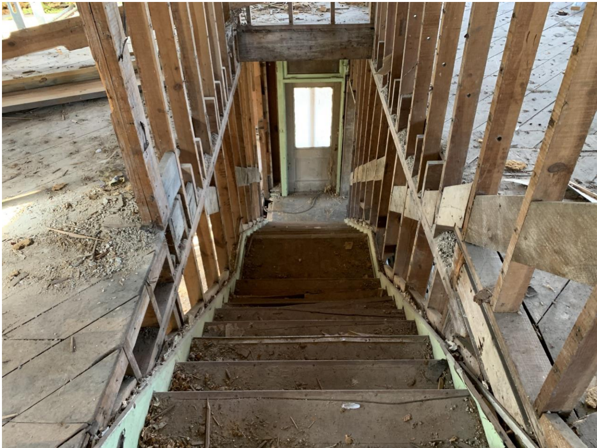
Photo 18, second floor, top of stairs facing front entryways
