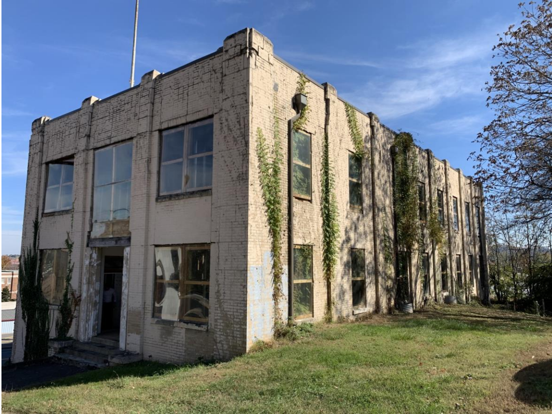
Photo 11, Front and east elevations from W 2nd North Street
