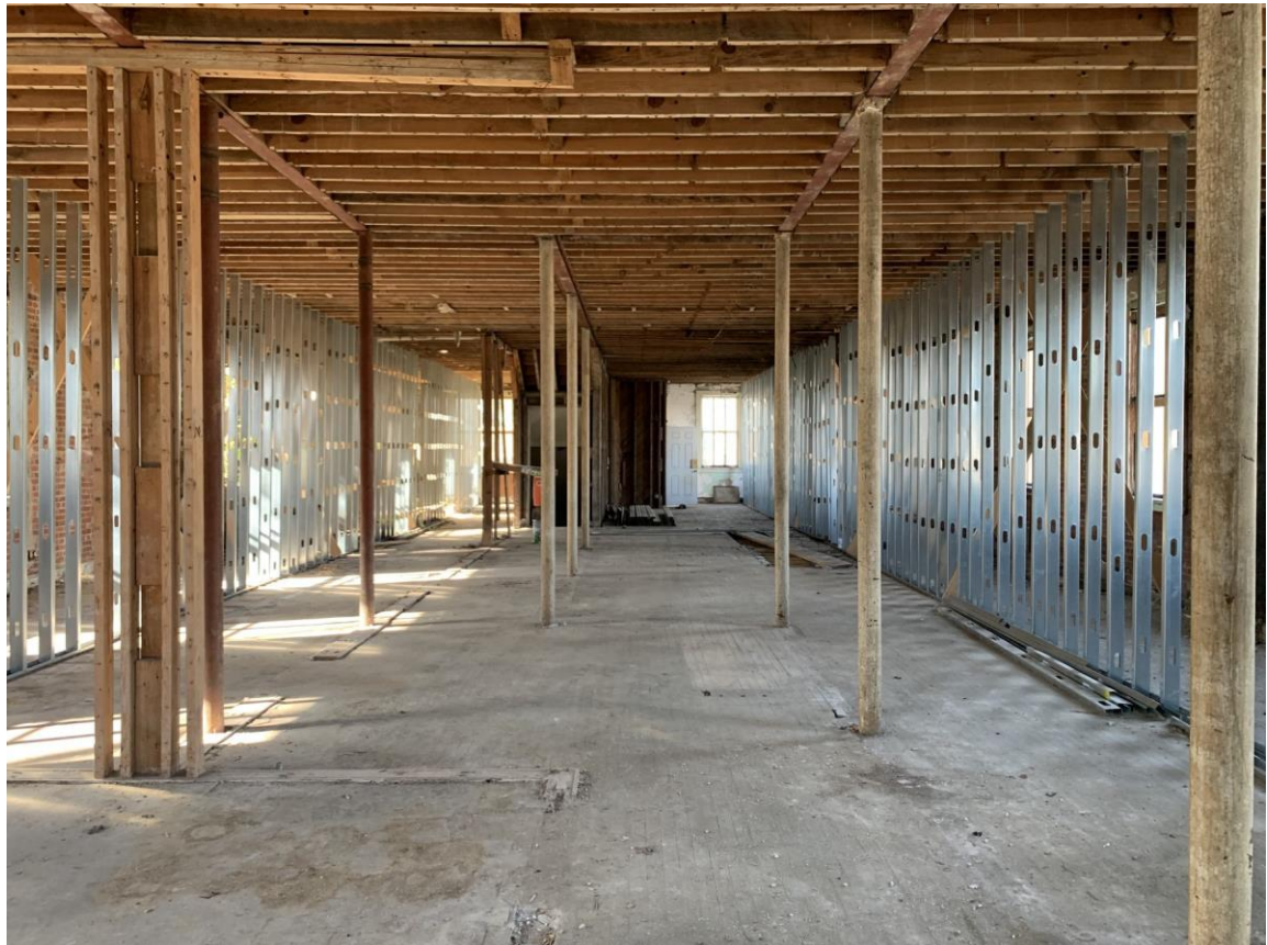
Photo 16, first floor, facing front of building
