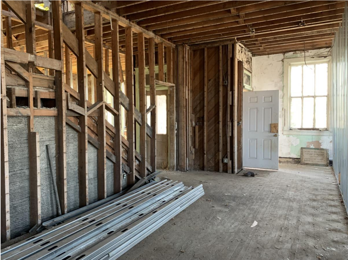
Photo 14, First Floor facing front entryways and stair
