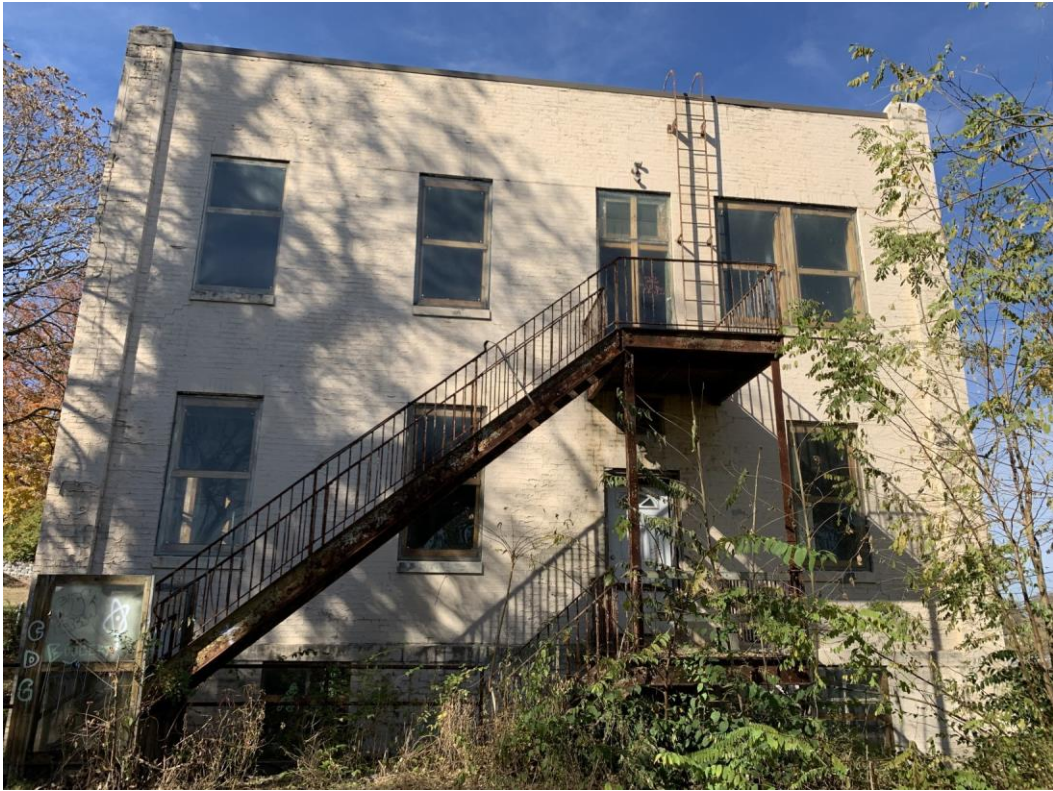
Photo 9, Rear elevation, camera facing northwest
