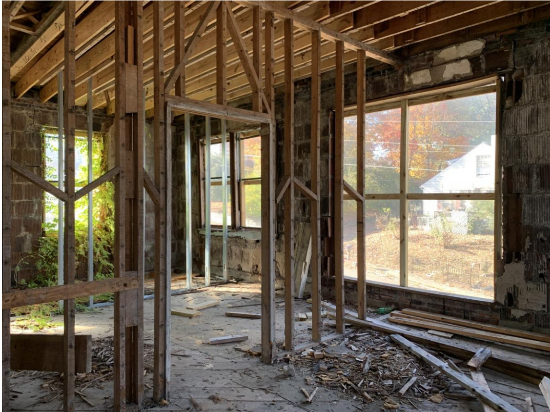
Photo 19, second floor, northwest corner of building
