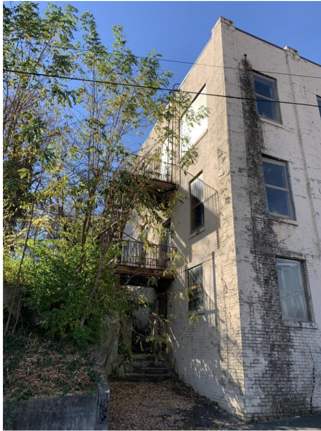
Photo 7, Rear elevation as seen from North Henry Street
