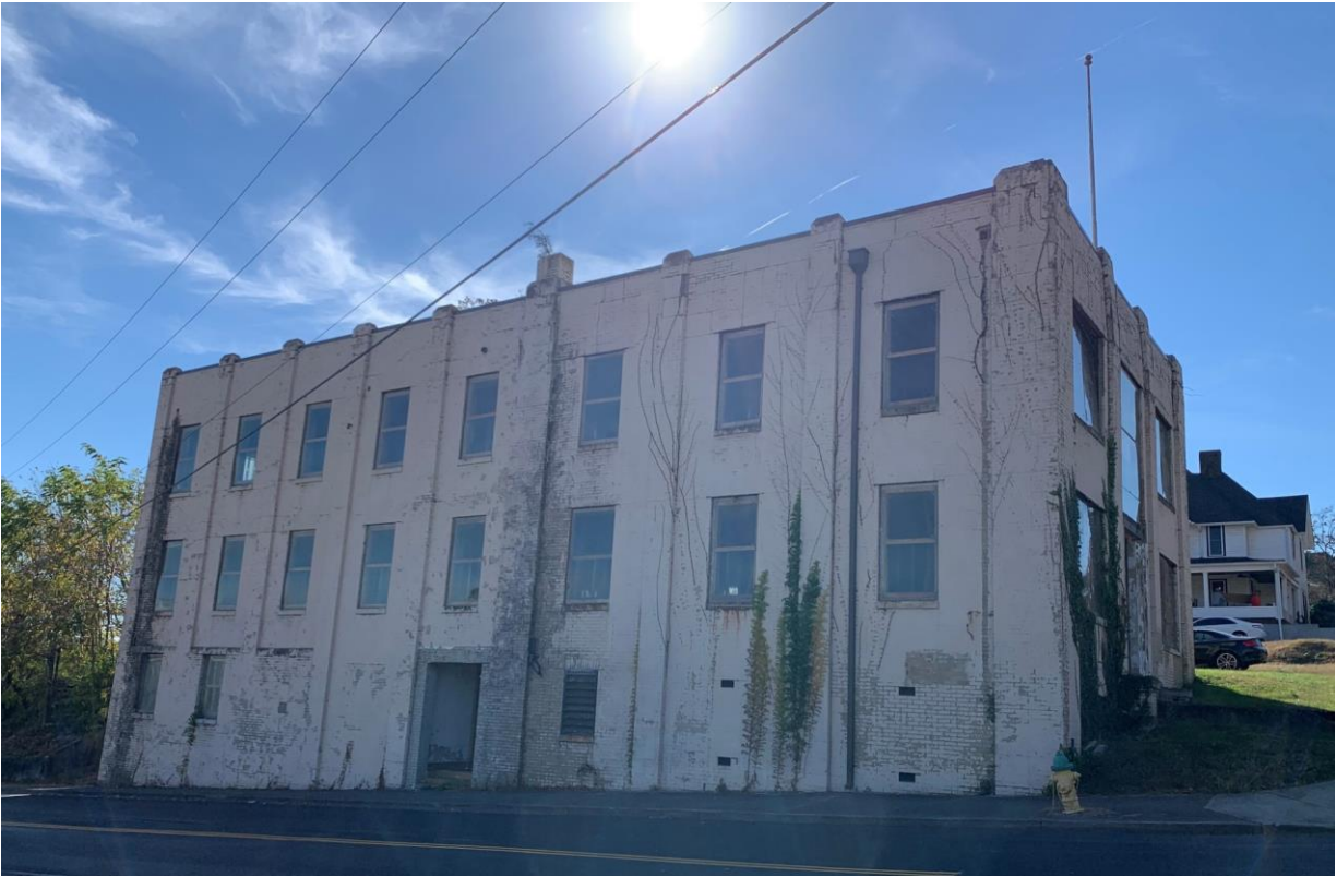
Photo 5, East elevation from North Henry Street
