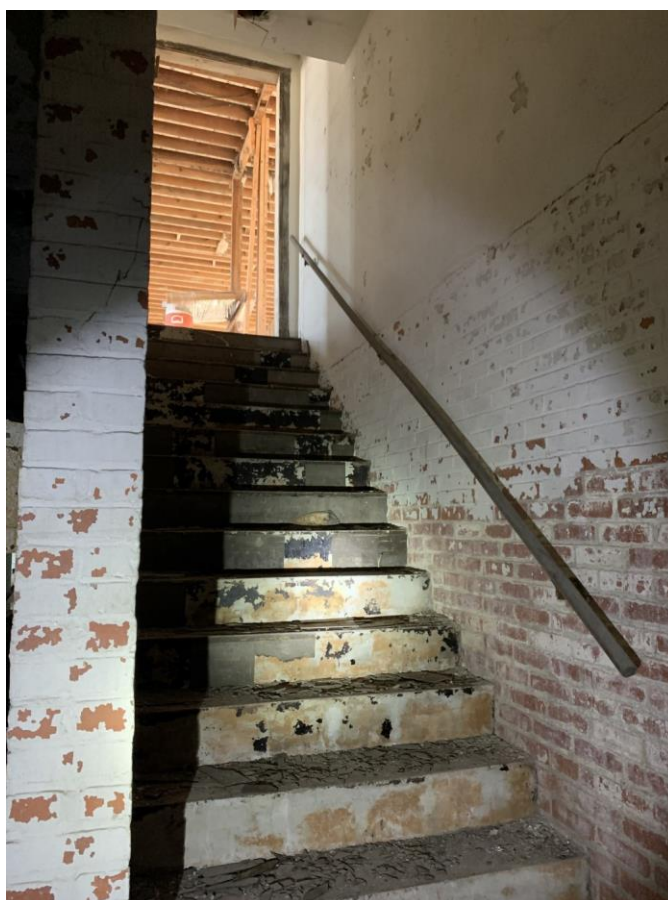
Photo 24, basement, camera facing stairs to first floor
