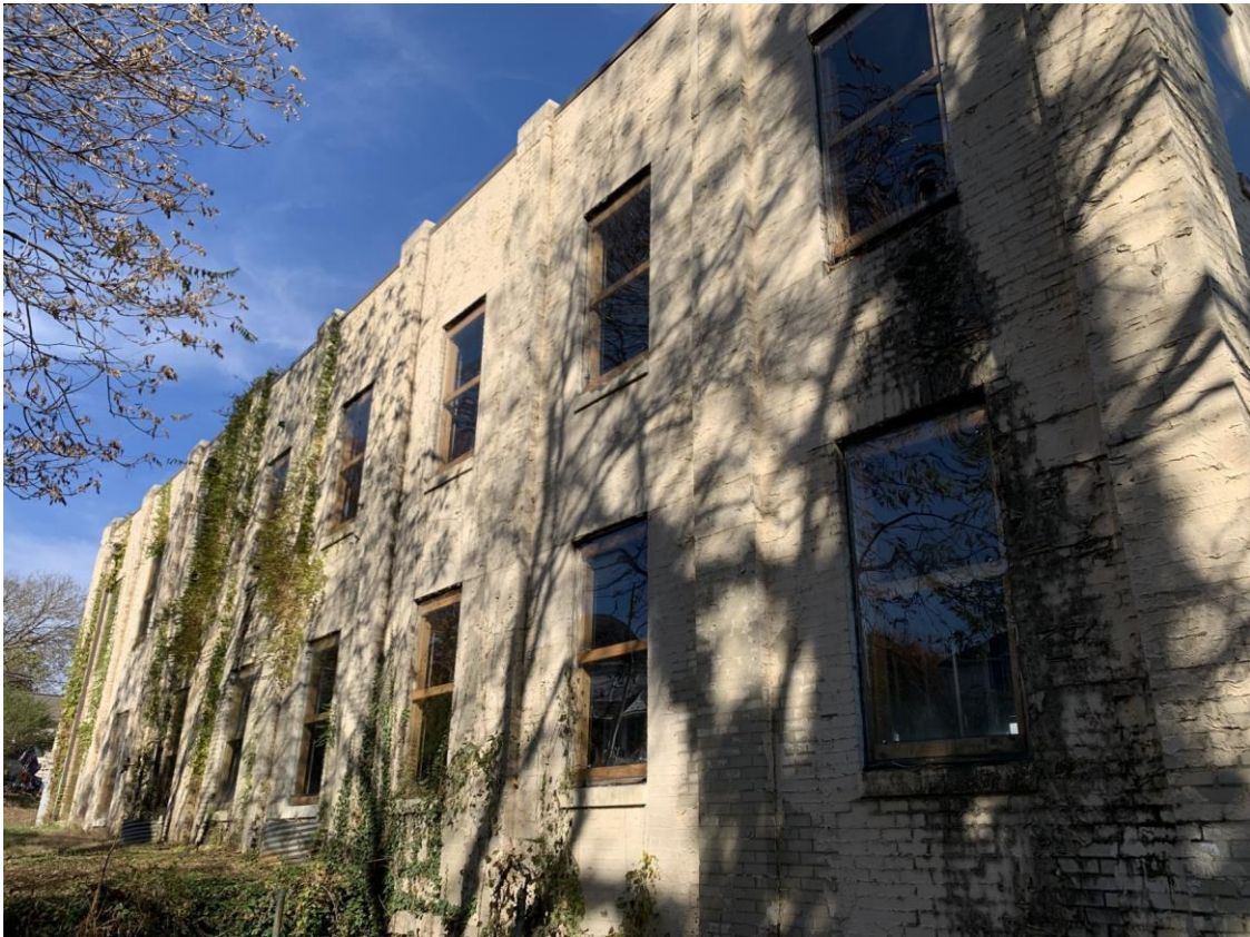
Photo 10, West elevation, camera facing northwest
