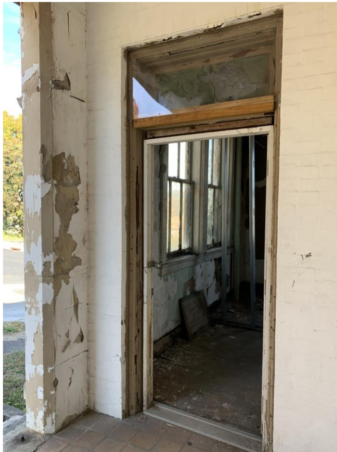
Photo 4, Front façade, inset entryway, left door
