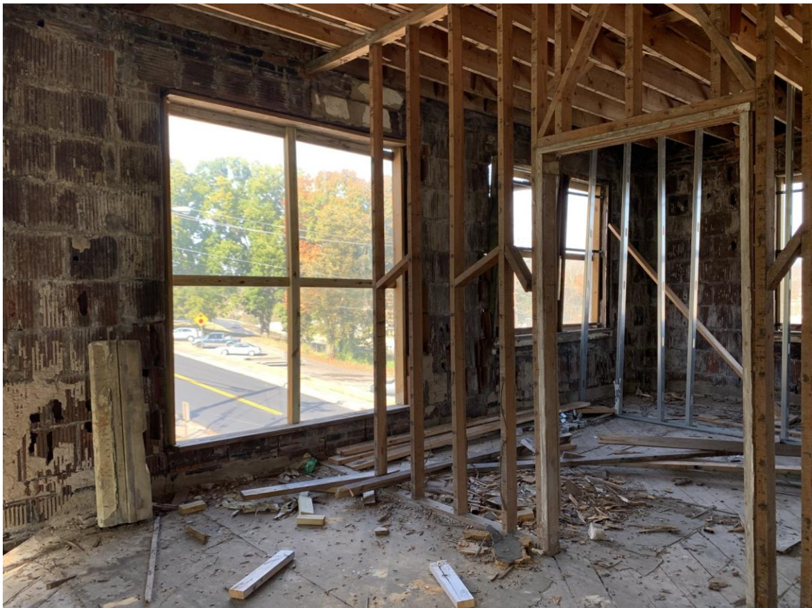
Photo 20, second floor, front façade and northeast corner of building
