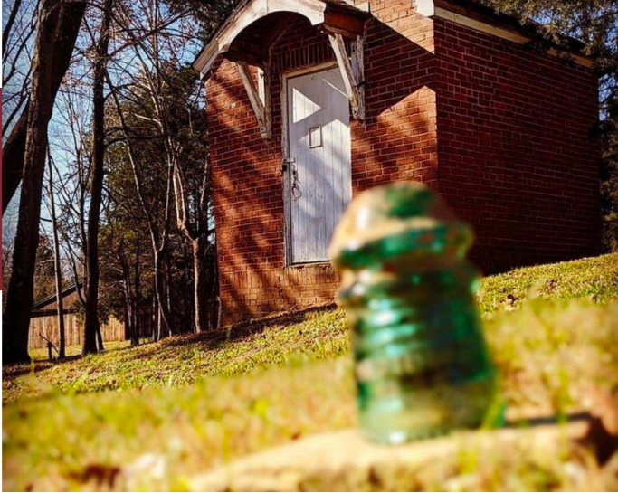
This is the Telephone Switchboard Office at Port Royal State Historic Park, with an early 20th century insulator in the foreground. The switchboard office was constructed in the 1920's.
