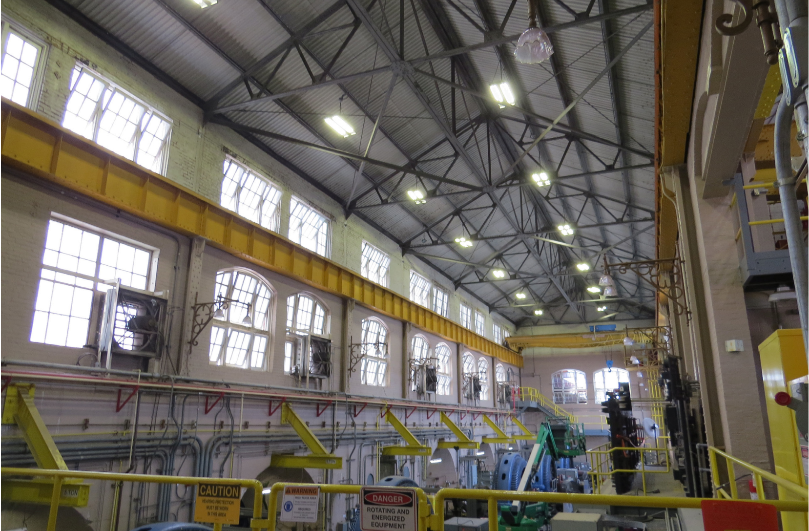
Ocoee No. 1 powerhouse interior, 2023. Photo courtesy of Caty Dirksen.
