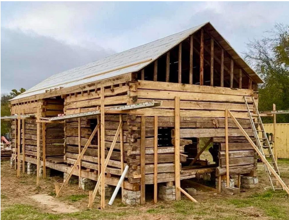
Reconstruction Progress at the ca. 1810 Frontiersman Cabin in Fayetteville.
