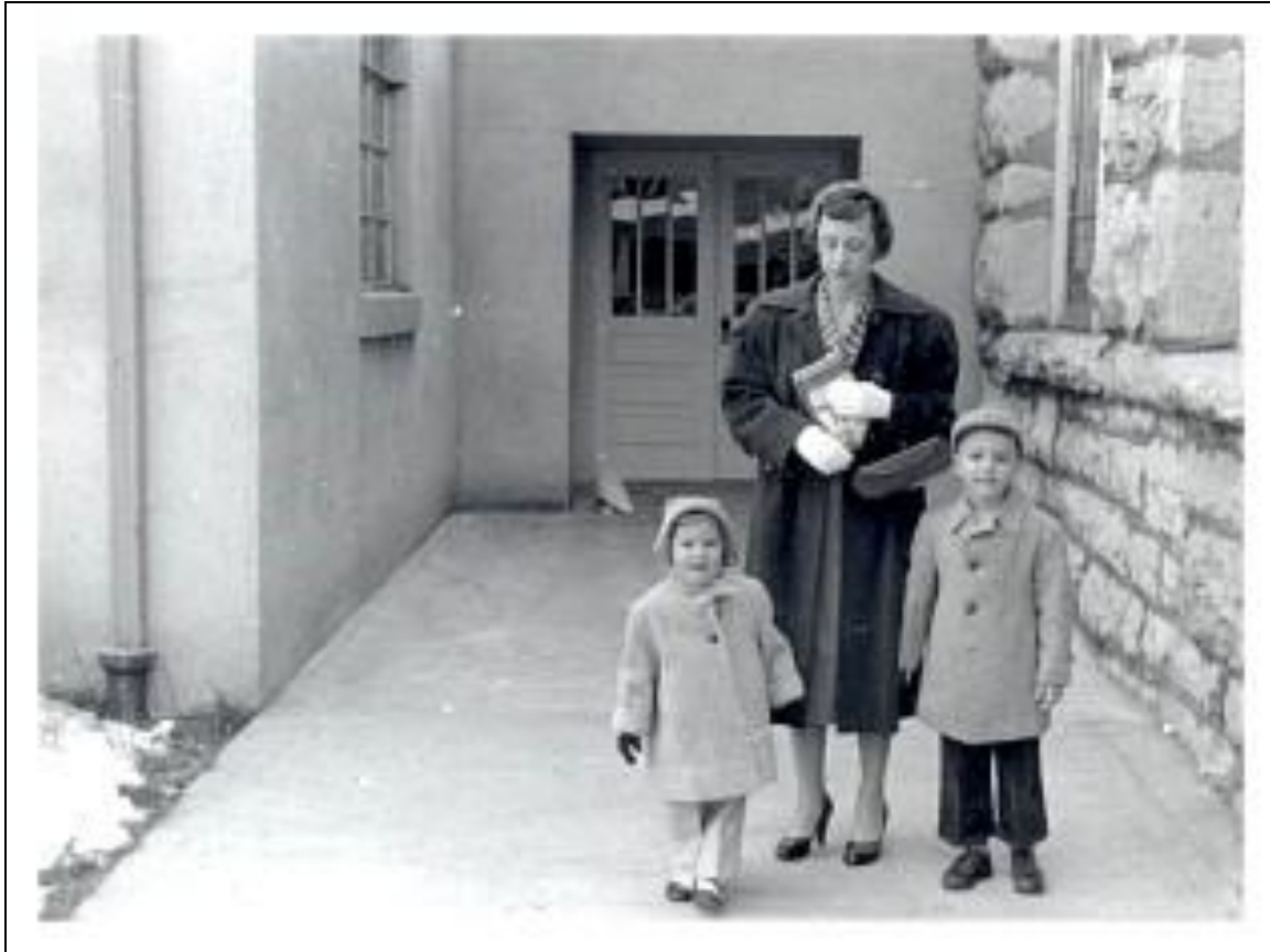
Figure 6. Circa 1955 archival photograph, showing the rear addition shortly after construction at left and center, and the west elevation of the original church building. Photograph courtesy of Joseph Payne.
