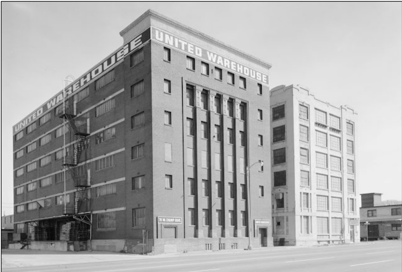
Figure 7: Photo from the HABS Collection, 1974, shortly after United Warehouse purchased it. Whitehead, Josh. "J. R. Watkins Building", Crème de Menth, Accessed November 17, 2025. https://cremedememph.blogspot.com/2020/03/jr-watkins-warehouse.html .
