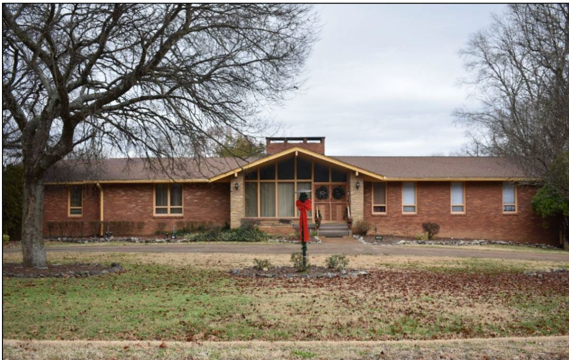
Figure 32. Photograph of 4320 Setters Road, looking east, 2018.
