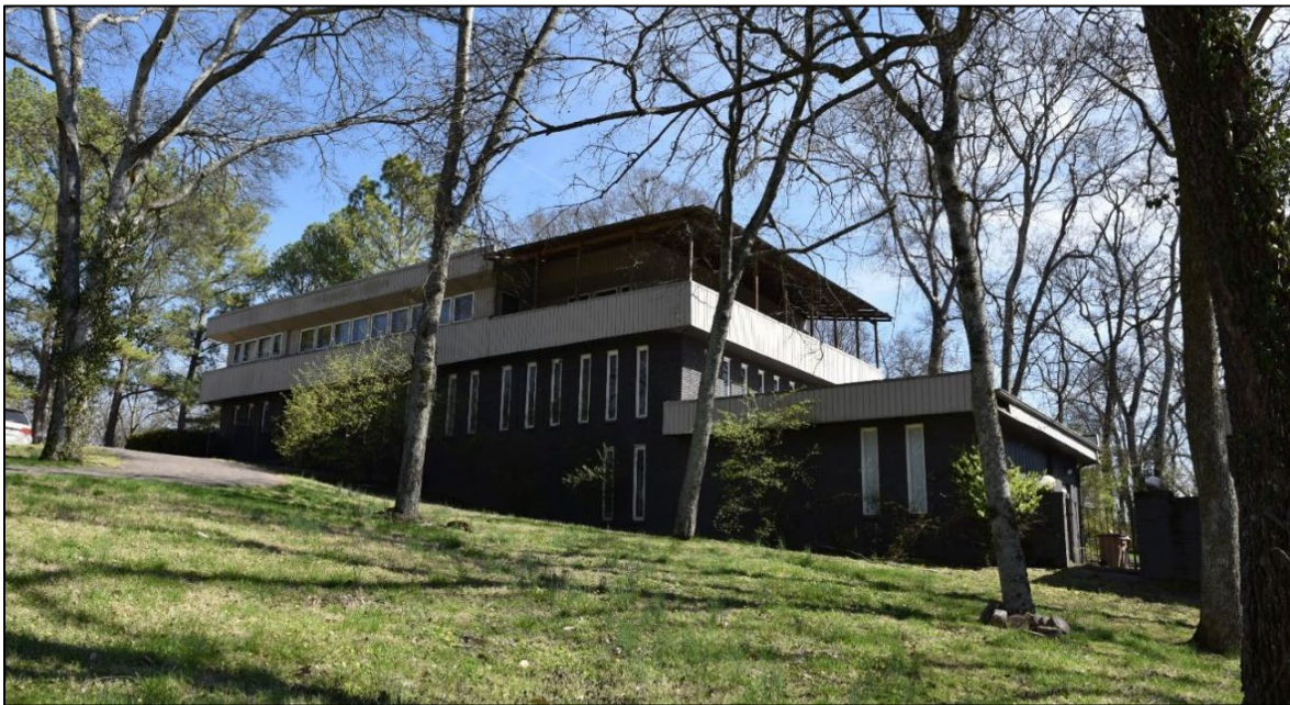
Figure 23. Photograph of the Sowell-designed house at 2488 Walker Lane, 2025.
