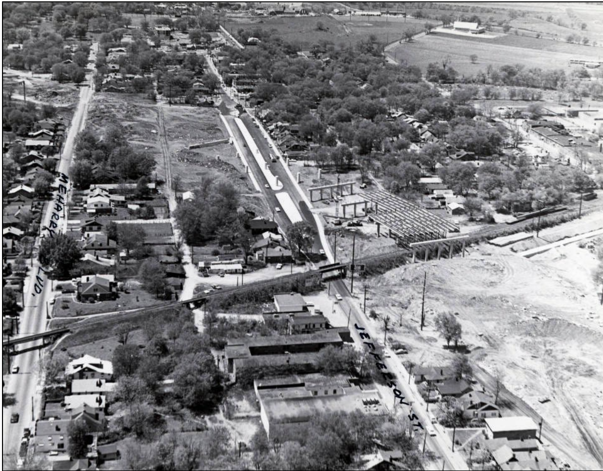
Figure 9. Aerial photograph of the I-40 interchange under construction at Jefferson Street, c. 1969. 109
