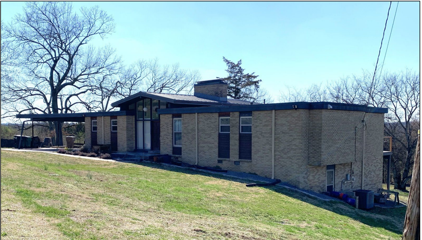
Figure 22. Photograph of 1716 Windover Drive, looking southwest, 2024.
