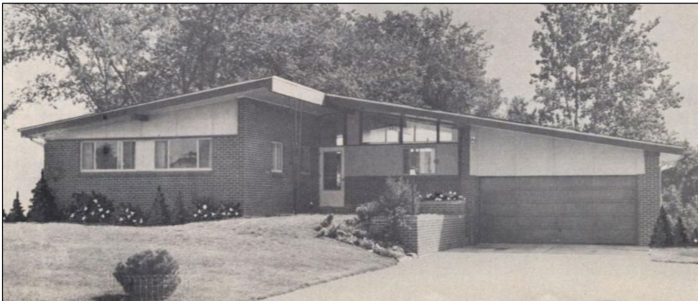
Figure 166. Photograph of a typical Contemporary-style dwelling, 1960. 167
