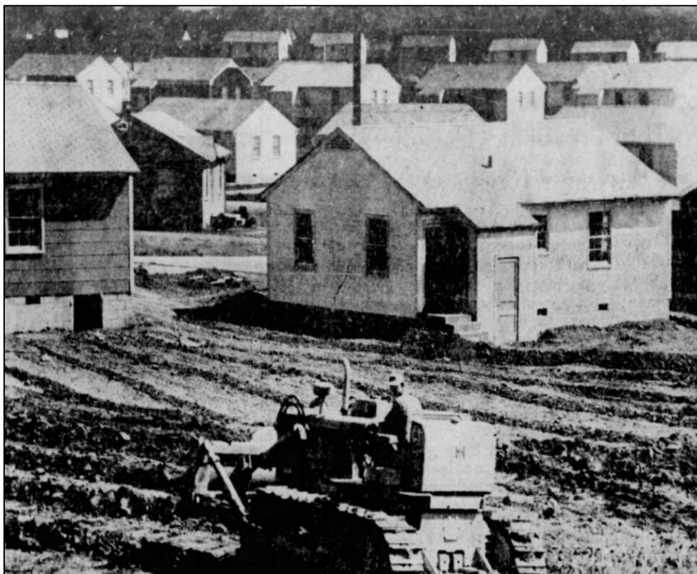
Figure 30. Photograph of dwellings in Cumberland Gardens under construction, 1959. 191
