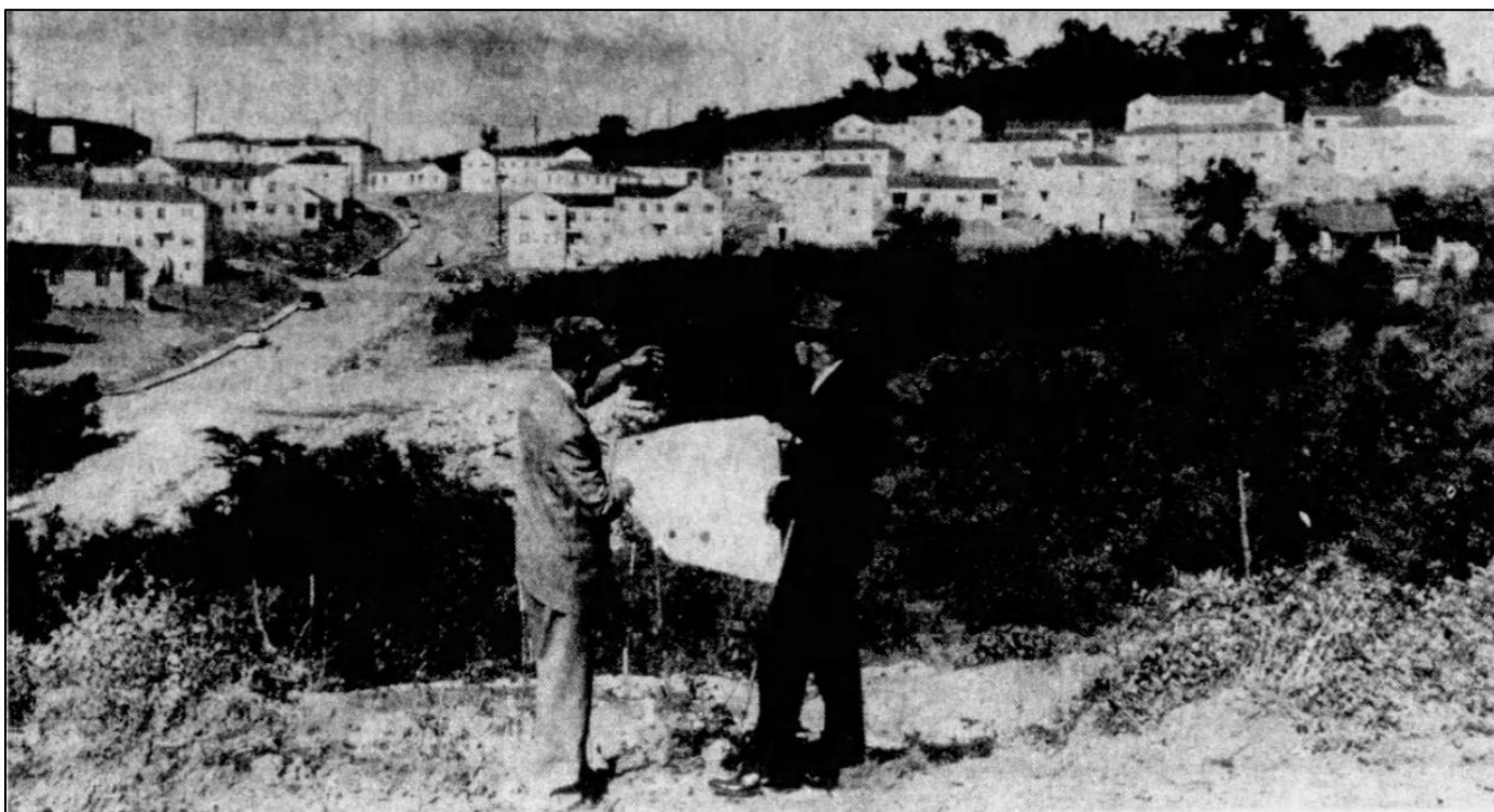
Figure 18. Photograph of Calvin McKissack (left) and Moses McKissack III (right) at the College Hill development site, 1952. 173
