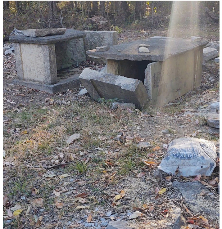
Box tombs as they looked prior to the repair, note they have sunken in the ground over time. Portions of the tombs were not initially visible and had to be recovered to complete the work.
