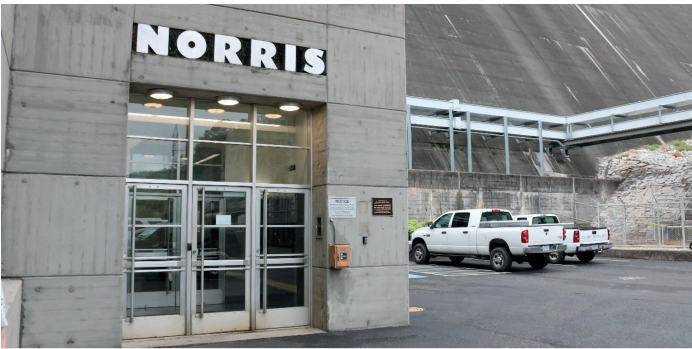
Figure 2 Norris Dam Powerhouse Source: Hallie Hearnnes, Tennessee Valley Authority
