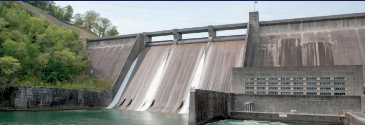
Figure 1 Norris Dam, featuring its central spillway Source: Tennessee Valley Authority
