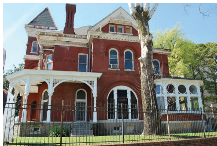
Side elevation view of the Lowenstein House.
