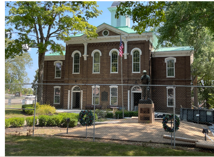
Loudon County Courthouse. The courthouse was undergoing restoration efforts and ADA upgrades at the time the photograph was captured. Photograph by Rebecca Schmitt, August 2024.
