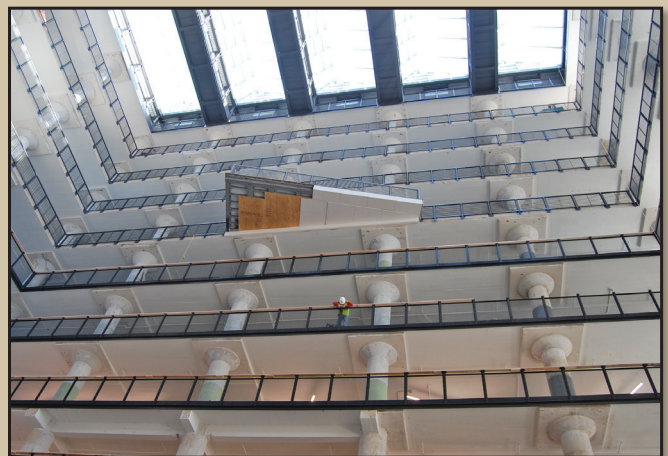
View of the Crosstown Concourse atrium
