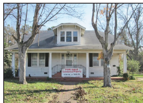
Dr. Thomas H. Price House, west façade, view to east.
