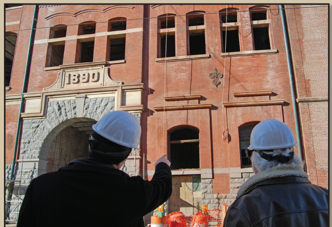
Tony Pellicciotti and Louis Jackson check out progress on the Tennessee Brewery rehabilitation.
