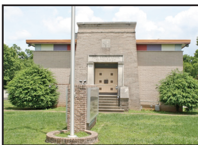
West façade of Egyptian Revival-style Jere Baxter Masonic Lodge, view to east.
