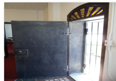
Old Grainger County Jail original entry door
