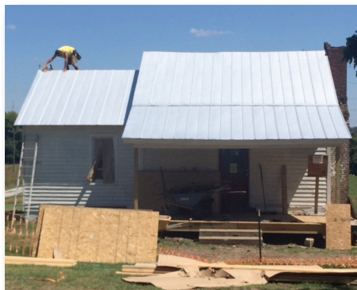
Restoration Work on Clover Bottom Slave Cabin.
