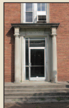
Griggs Hall, detail of entrance on south facade
